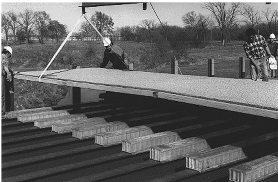
FIGURE 1.5 Placement of FRP sandwich deck.
