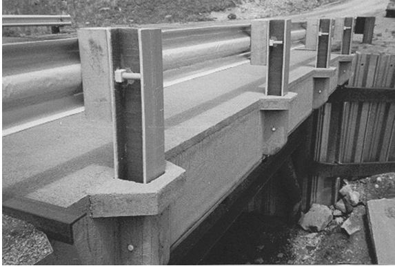
FIGURE 1.4 FRP sandwich deck with attached guardrail.
