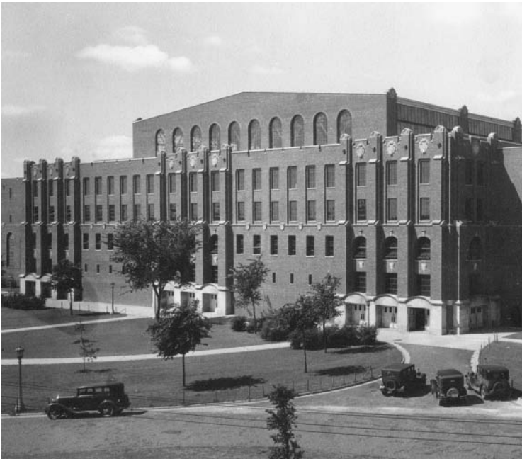
An archival photograph of the Field House shows the façade prior to the administrative addition of 1955.
