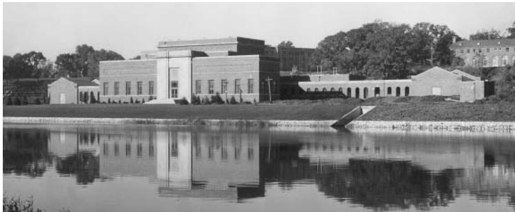
An archival photograph of the late 1930s shows the Art Building prior to the construction of Abramovitz's 1968 Printmaking Wing.
