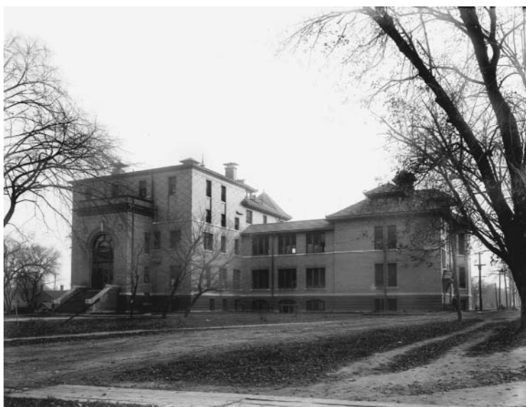
An archival photograph of circa 1900 shows the original Seashore Hall facing Jefferson Street.
