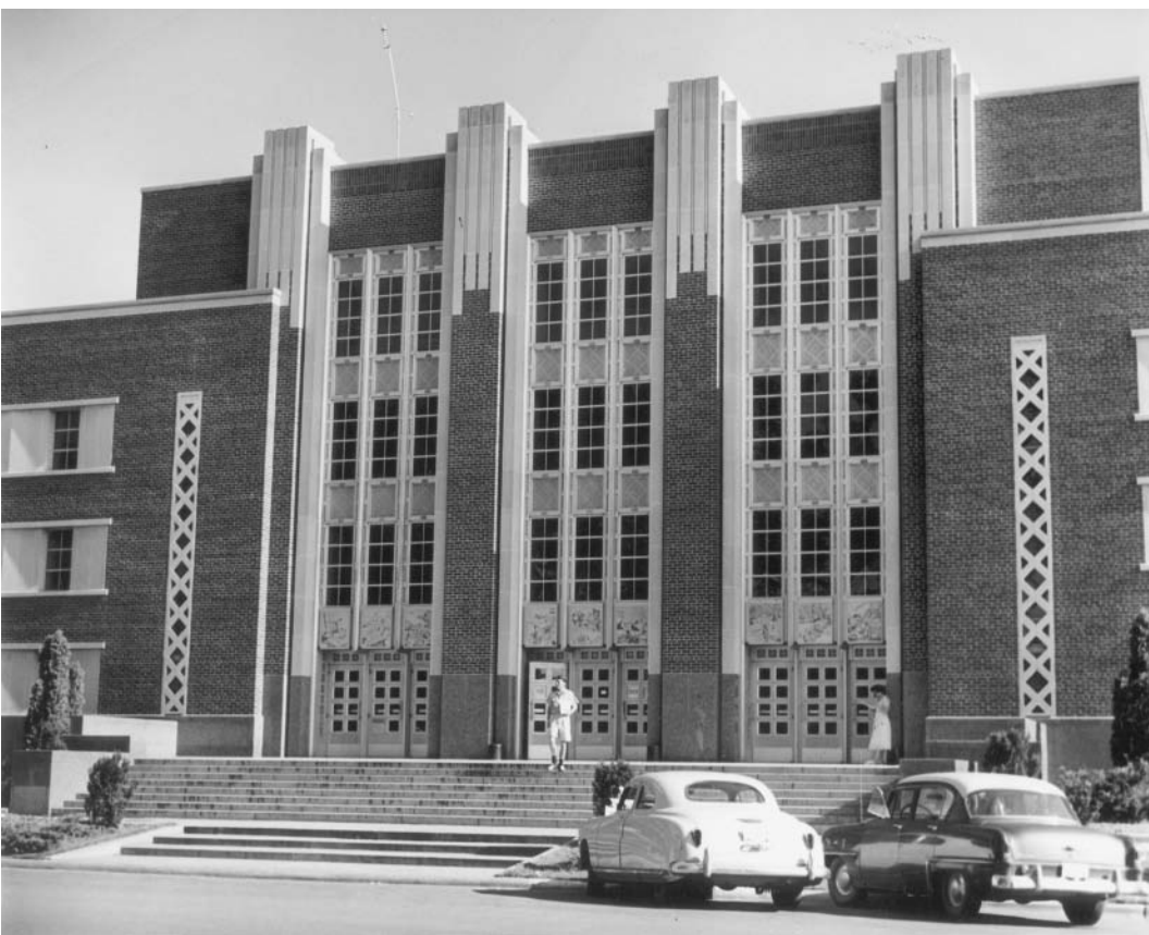
The original 1951 Keffer and Jones Main Library north façade was the sole example of Zigzag Moderne on the UI campus. Twenty years later it was masked in a Modernist remake of the library.
