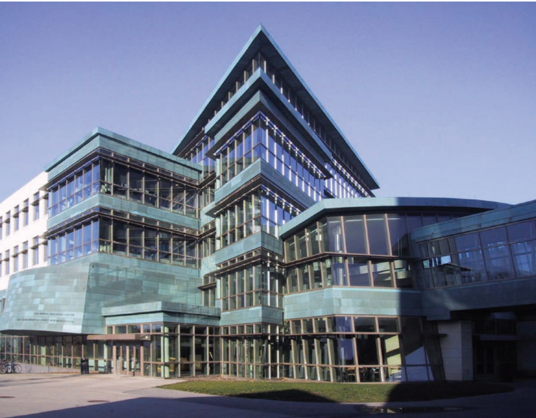
14. The asymmetrical volumes and upward mounting acute angles of the copper-clad Medical Education and Research Facility, 2002, make it the leading exponent of Postmodernism on the Medical Campus.
