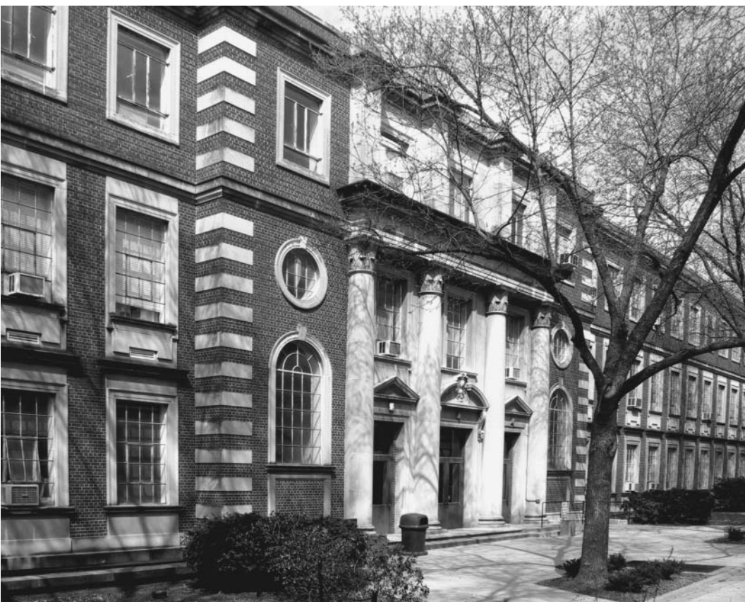
The Chemistry Building combines classical formality (columns, portico, pediments, quoins) with industrial-duty steel windows.
