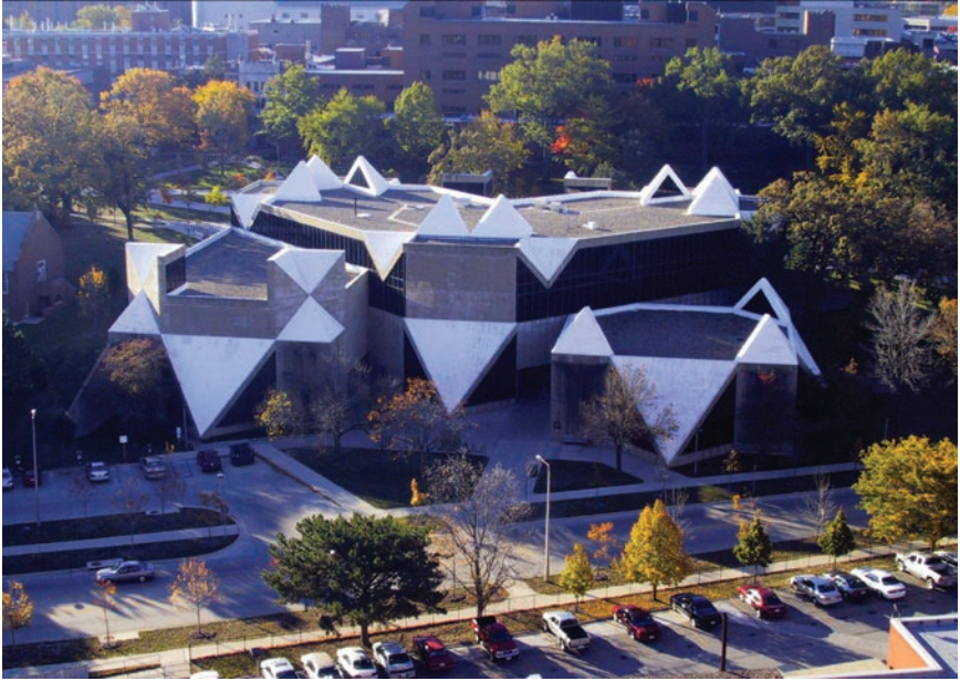
9. Hardin Library for the Health Sciences, 1974, has distinctive pyramidal skylights and prominent inverted triangles.
