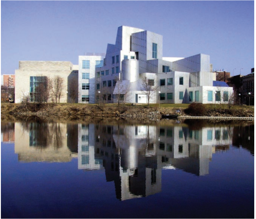
12. Iowa Advanced Technology Laboratories, river façade, 1992, unfolds a composition of fragmented volumes referencing the geometry of the Iowa farmscape.
