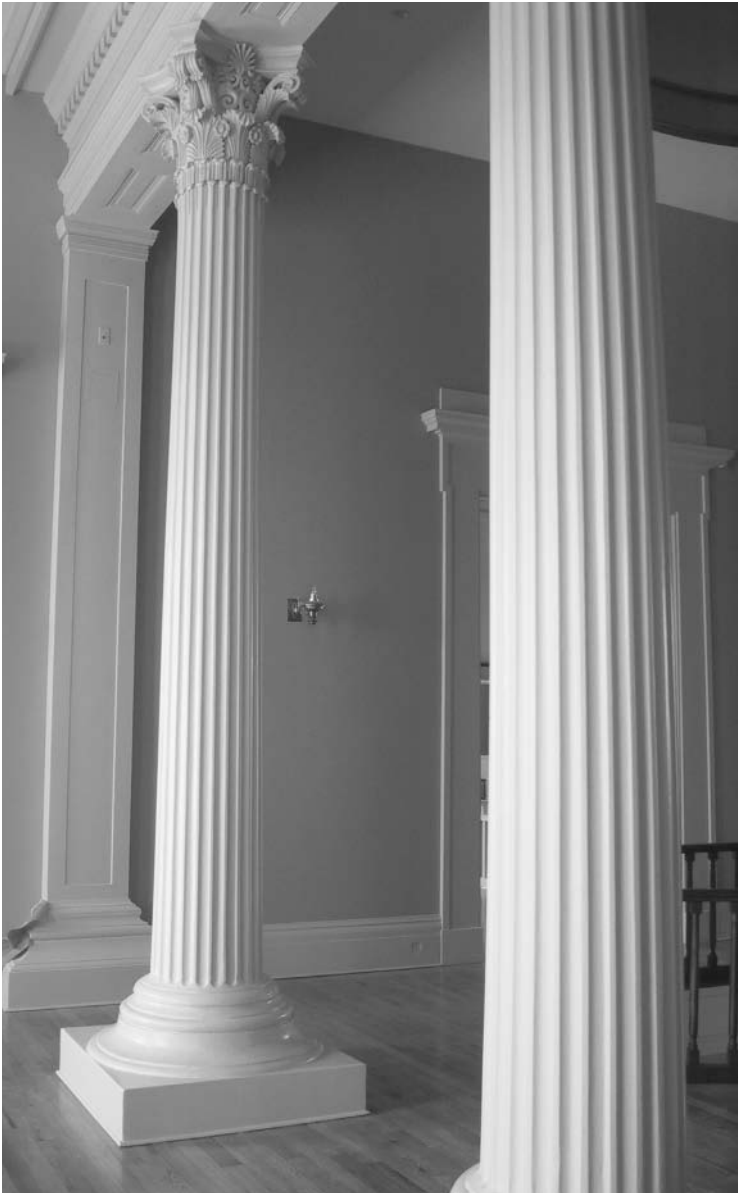
The elegant fluted Corinthian columns of the second floor interior, with capitals based on those of the Choragic Monument of Lysicrates, Athens.
