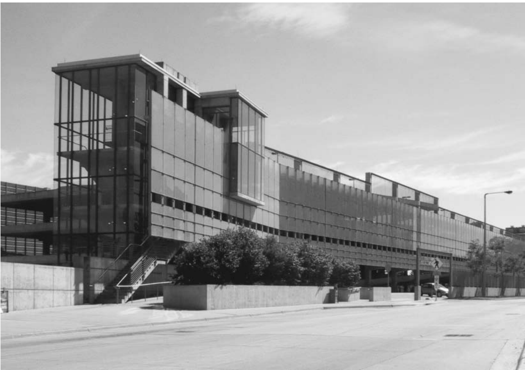
The Newton Road Parking Ramp exemplifies how good design can grace even utilitarian structures.
