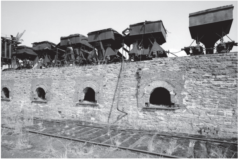
FIGURE 2.2 Coke ovens built in 1906, Shoaf Mine & Coke Works, Fayette County, Pennsylvania. Courtesy of US Library of Congress, Prints & Photographs Division. Reproduction number: HAER PA, 26-SHO, 1–3
