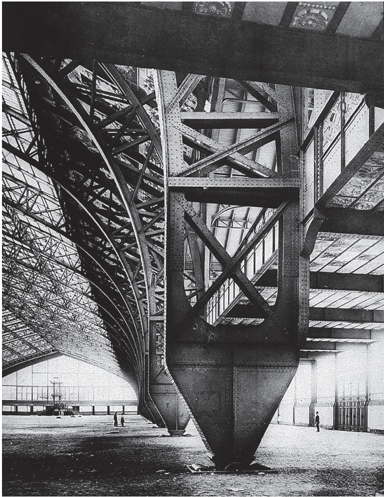
FIGURE 5.8 Galerie des Machines constructed for the Paris Exhibition of 1889. Source: Leonardo Benevolo History of Modern Architecture Volume 1 London: RKP, 1971; trans. from Storia dell'architettura moderna , Italy: Giuseppe Laterza & Figli, 1960
