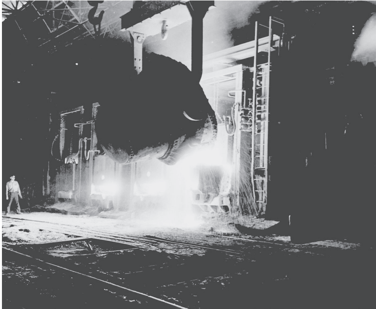
FIGURE 4.1 Molten steel pour at Jones and Laughlin Steel Company, Pittsburgh, May 1942. Courtesy of US National Archives and Records Administration
