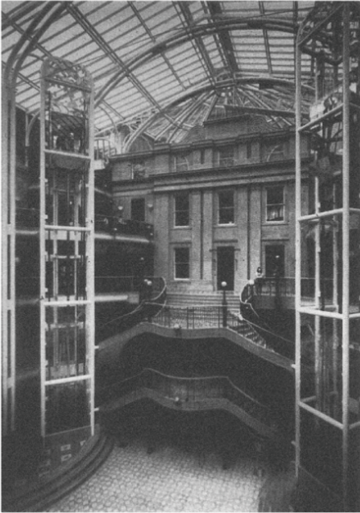
Exposed columns support the roof of Princes' Square.
