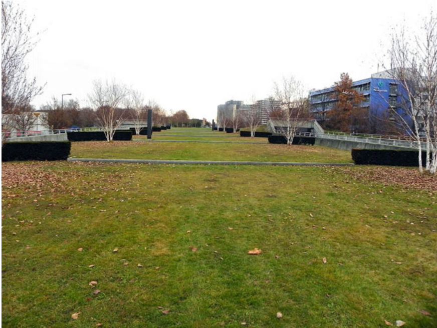
Fig. 11.5 The Petuelpark in Munich presents a pioneering attempt to cover a major highway with a concrete deck to abate its chronic environmental nuisance. A greenroof has been installed on the top of the huge deck to bestow considerable landscape and ecological value on the neighbourhood. Opened in 2002, it denotes an innovative solution to urban blight caused by major transport infrastructure in cities ( Photo credit C.Y. Jim )
