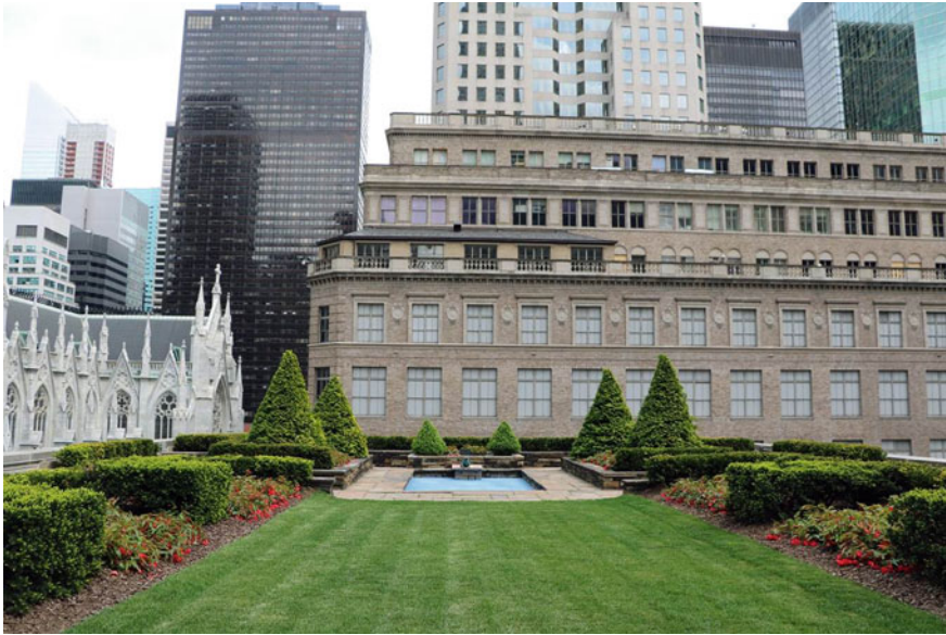
Fig. 11.1 One of the greenroofs with formal design on the podium of the Rockefeller Center in New York. It is composed of extensive and semi-intensive types and a shallow pond. Opened in 1936, it is the oldest remaining greenroof on a commercial building in North America ( Photo credit Tishman Speyer)
