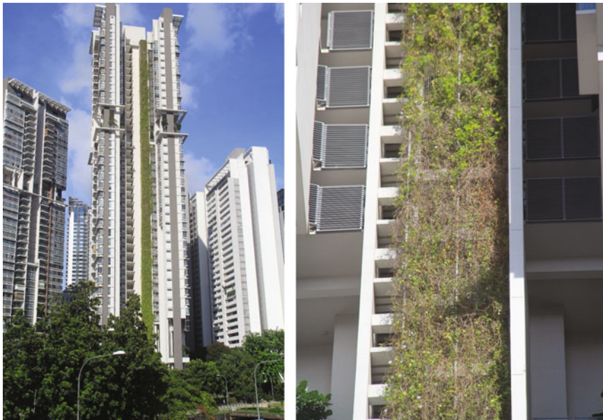
Fig. 2.1 A towering green wall covering the stairwell of a residential building in Singapore ( left ). However, while ambitious as a design feature, the creepers on trellis can reduce daylight and ventilation in the stairwell, and the green wall is only visible on exterior of the building. The visual attractiveness is questionable, ecological functions are limited, and maintainability of the system is low ( right ) (Photo credit P.Y. Tan)
