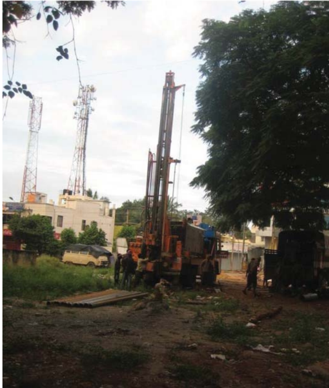
Figure 3.6 Bore well drilling under progress.
