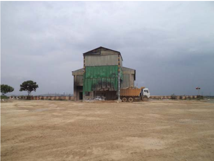
Figure 6.19 A crusher hopper in mining area.
