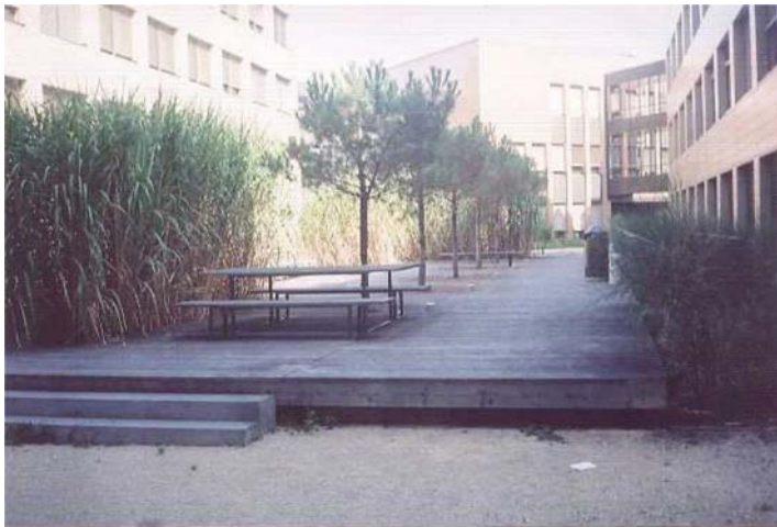
Plate 4.35 Constructed wetlands built between buildings.
