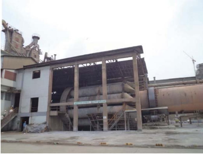
Figure 5.3 Air-cooling arrangement made to cement kiln.
