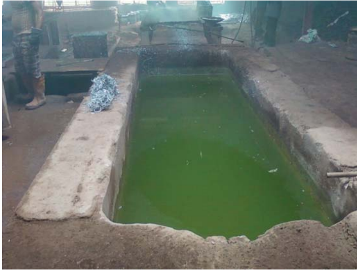
Figure 8.16 Example of bad safety procedures that still exist in developing countries.
