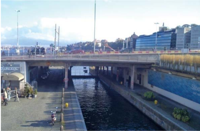
Figure 6.2 A canal connecting water bodies in Stockholm.
