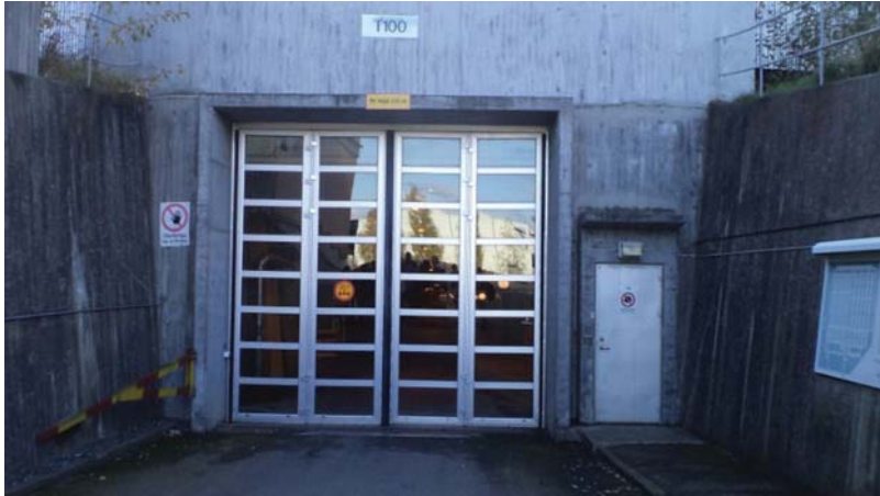
Figure 7.2 Entrance to wastewater treatment plant located underground at Stockholm. Such a location can avoid freezing of water during a severe winter and save construction costs.
