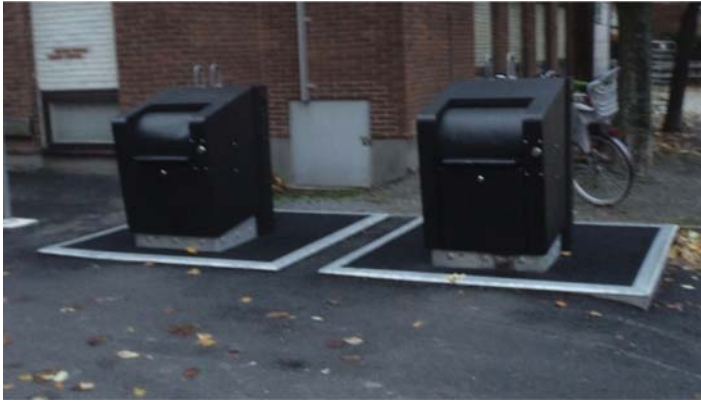
Figure 2.31 Waste-dropping place; pneumatic solid waste conveying system.
