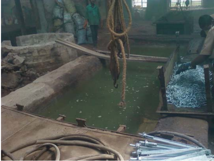
Figure 5.14 A typical galvanizing rinsing tank.
