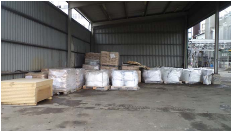
Figure 8.21 Chemicals stored at a wastewater treatment plant site.
