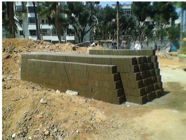
Figure 7.8 Stabilized mud blocks moulded using soil at site.
