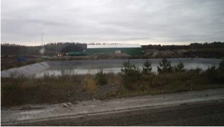
Figure 7.6 Earthen pond with liner to store leachate from landfill.
