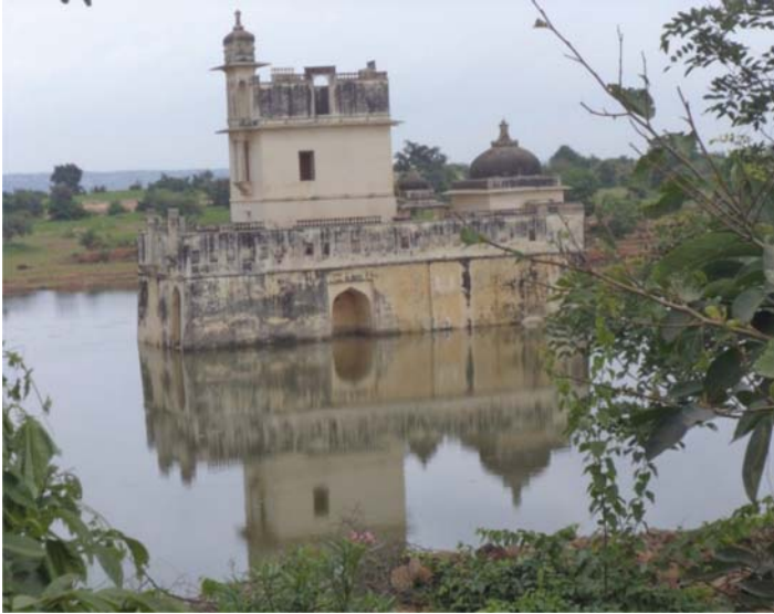
Figure 2.3 Water storage for drinking, agriculture, animal rearing and temperature maintenance of a building in ancient India.
