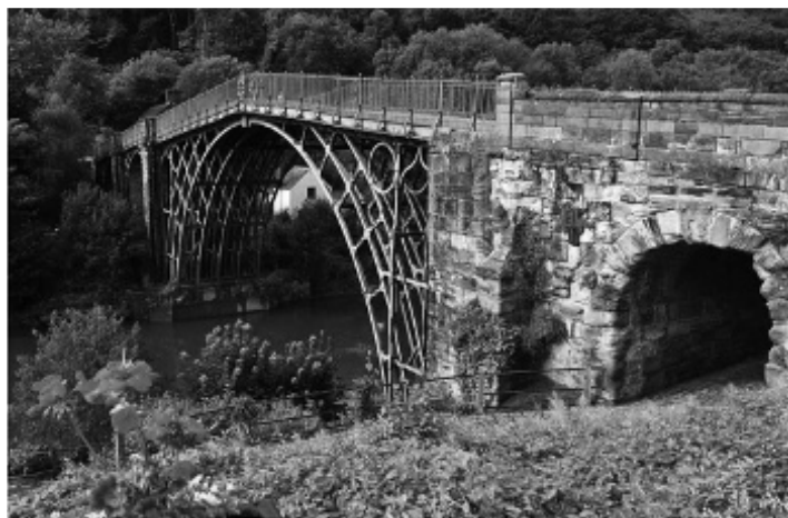
Figure 2.5 Ironbridge at Ironbridge Gorge, Shropshire, UK. This was the first bridge made of iron ever to be erected ( http://commons.wikimedia.org/wiki/File:The_Iron_Bridge_%28272205816%29.jpg ).
