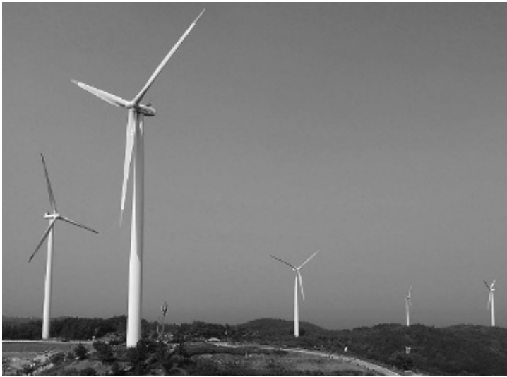
Figure 13.7 Wind power turbines.
