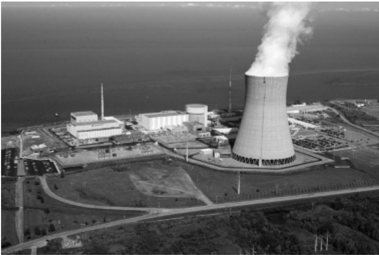
Figure 6.9 Nuclear power plant.
