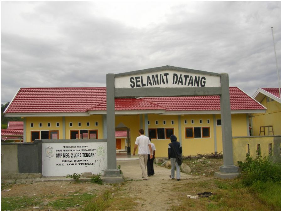
Fig. 5. Construction of Junior High School in Rompo (Lore Tengah) by an APBN-Grant along with exemption from school fees for the next years
