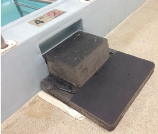
Cushioned nonskid steps leading to pool (Photo courtesy of Alan Schleier)
