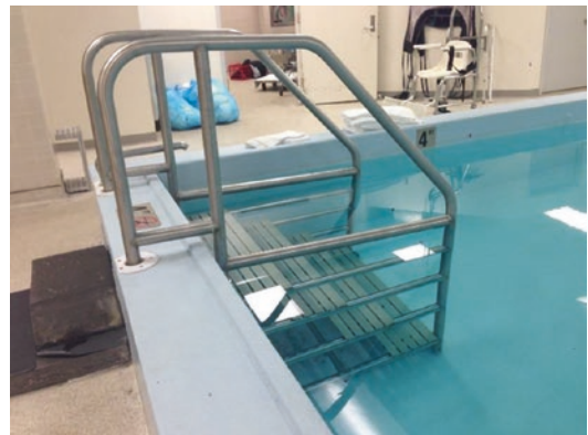
A set of nonskid stairs, complete with handrails to assist with safe transfer in and out of the pool (Photo courtesy of Alan Schleier)
