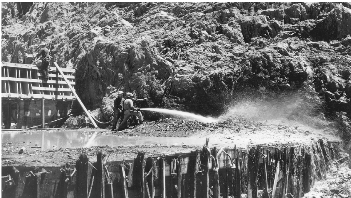
Workers remove dirt and rock from the construction site of Shasta Dam in 1942. Construction involved PWA funds as well as some CCC labor. (The Library of Congress.)
