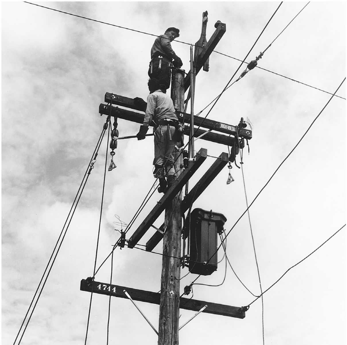
Workers on a transmission line in rural San Joaquin Valley, California in 1938. REA engineers worked to bring down the cost of rural electricity by employing more efficient materials and construction methods. (The Library of Congress.)
