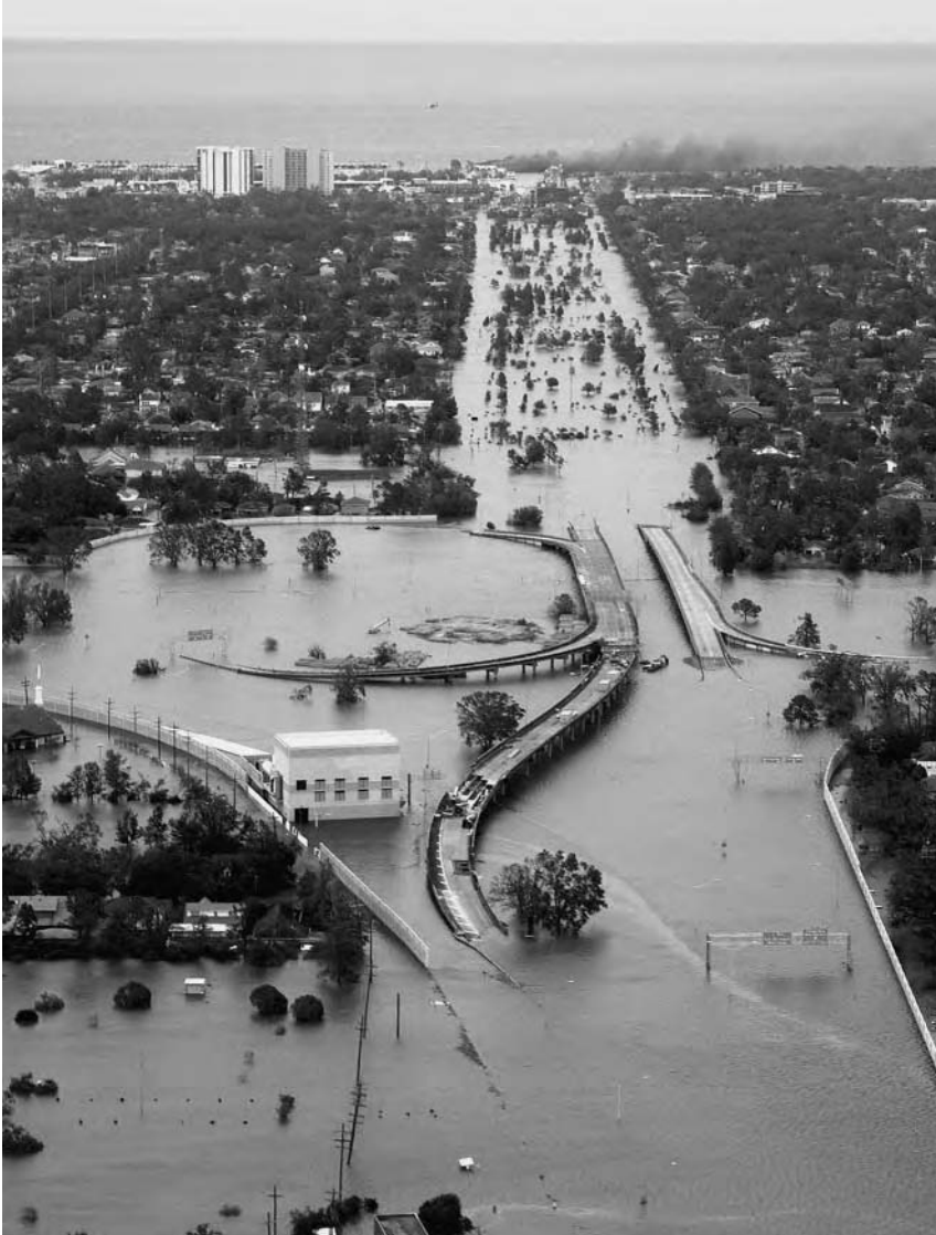
Plate 19.1 Flood impacts of Hurricane Katrina in New Orleans
