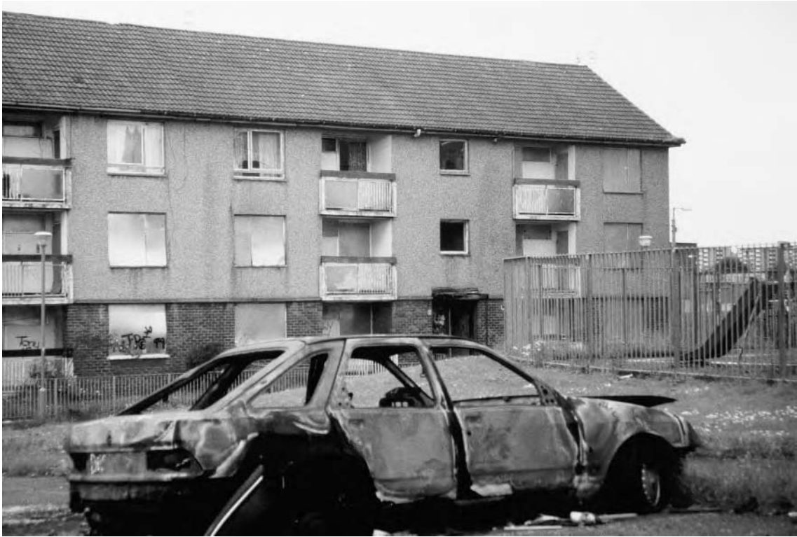
Plate 15.2 A stolen car lies burnt out next to a fenced-in children's play area in front of a block of local authority flats in the Possilpark district of Glasgow
