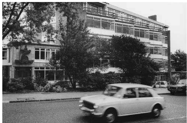
Plate 12 St Christopher's under construction, spring 1967.
