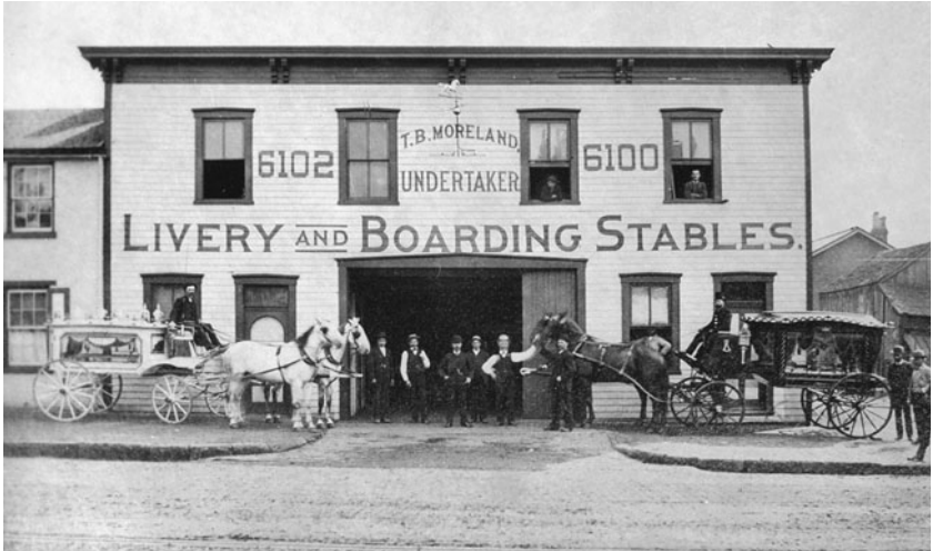
A combination livery stable and undertaking establishment in the East Liberty neighborhood of Pittsburgh, c. 1870. Notice the hearses on each side of the stable. Several Pittsburgh livery stables doubled as undertaking establishments. Source: Used with permission, Carnegie Library of Pittsburgh.
