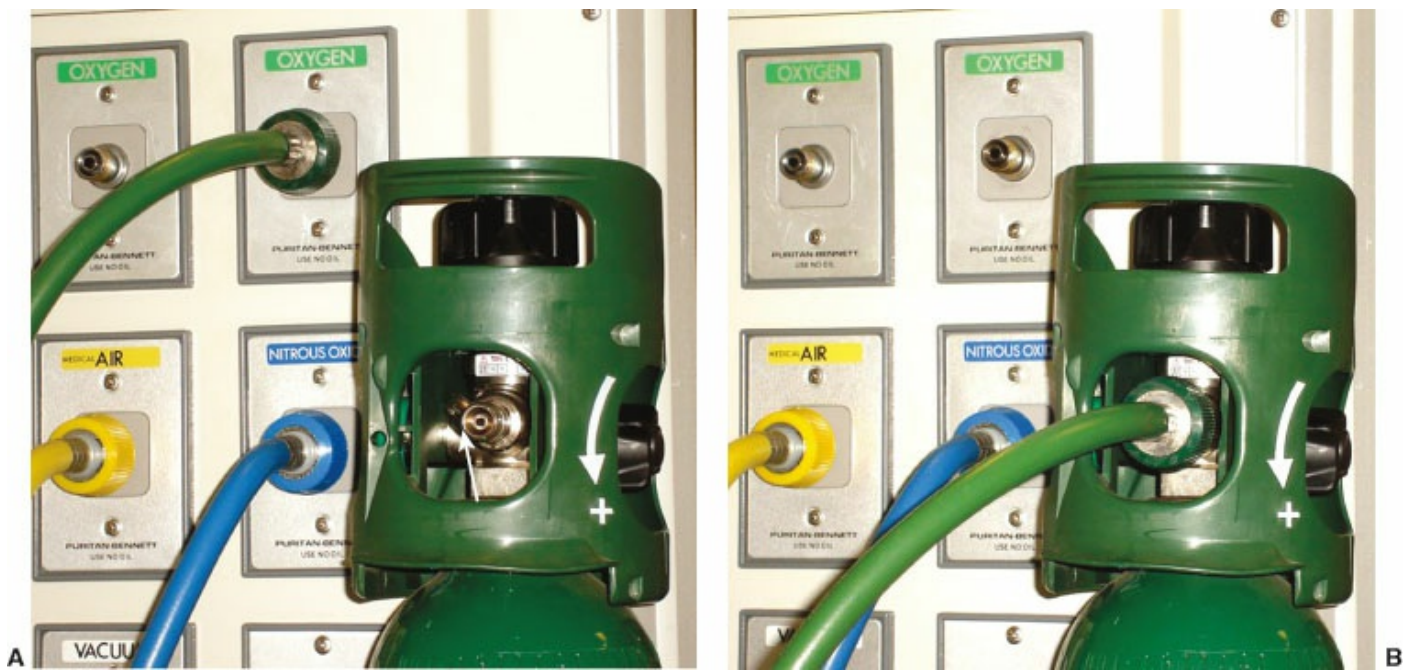
Figure 25-13 3,000 psig E-cylinder valve showing 50 psig DISS connection (arrow) (A) that could be connected to the machine oxygen hose if wall oxygen supply fails (B).
