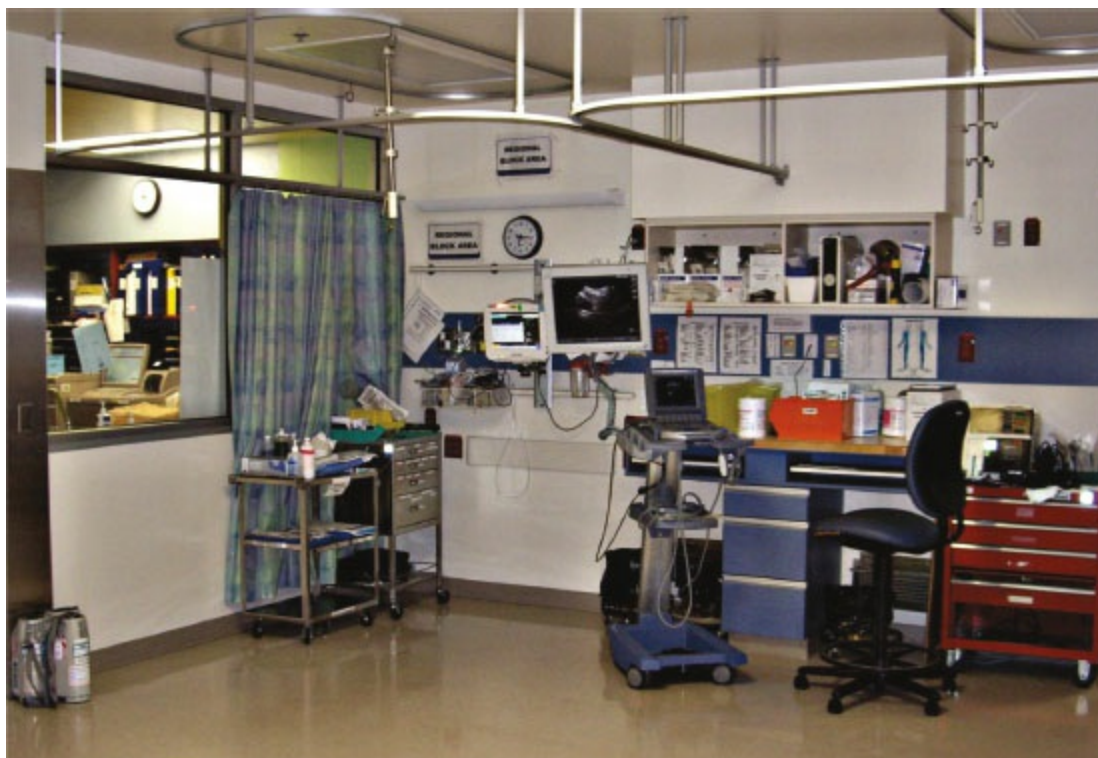
Figure 36-1 Designated regional block room with labeled storage cart.
