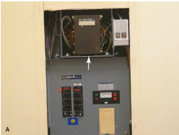
Figure 5-20 A: Isolated power panel showing circuit breakers, LIM, and isolation transformer ( arrow ). B: Detail of an isolation transformer with the attached warning lights. The arrow points to ground wire connection on the primary side of the transformer. Note that no similar connection exists on the secondary side of the transformer.
