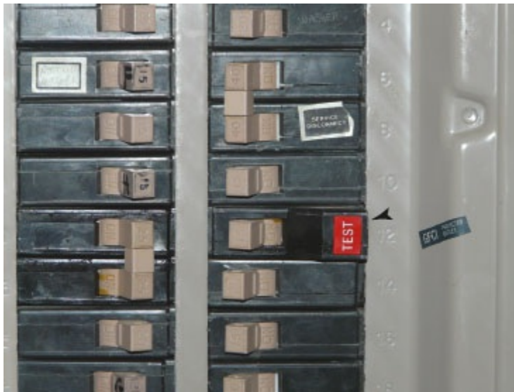
Figure 5-29 Special GFCI circuit breaker. The arrowhead points to the distinguishing red test button.
