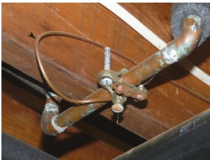
Figure 5-8 The arrowhead indicates the ground wire from the circuit breaker box
