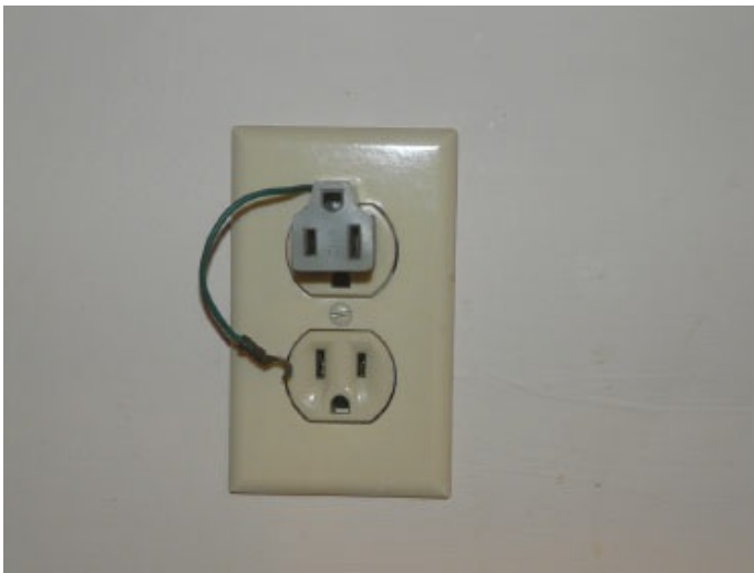
Figure 5-19 Right: a “cheater plug” that converts a three-prong power cord to a two-prong cord. Left: The wire attached to the cheater plug is rarely connected to the screw in the middle of the outlet. This totally defeats the purpose of the equipment ground wire.
