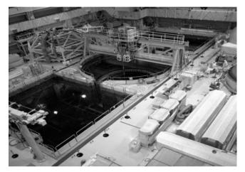
*5.1* Example of a fuel storage pool. This photo was taken during transfer of fuel from the reactor core (center) to the fuel storage pool (left). Courtesy of Energy Northwest, Richland, WA.
