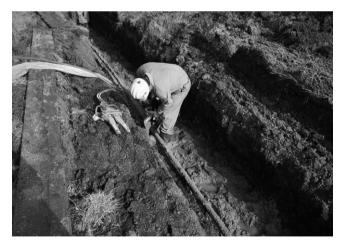
8.3 Removal of underground pipes, Argonne National Laboratory, USA.
