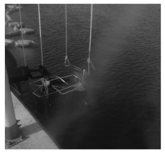
*24.7* Submerging zeolite into a water outlet from the Fukushima Daiichi NPP to reduce the radiation contamination to the ocean environment [39]. Used with permission from Tokyo Electric Power Company (TEPCO).
