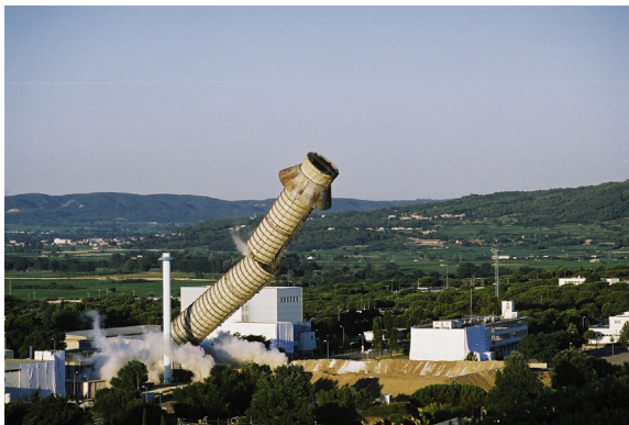
Figure 2.2 Stack at G1 reactor being dismantled.
