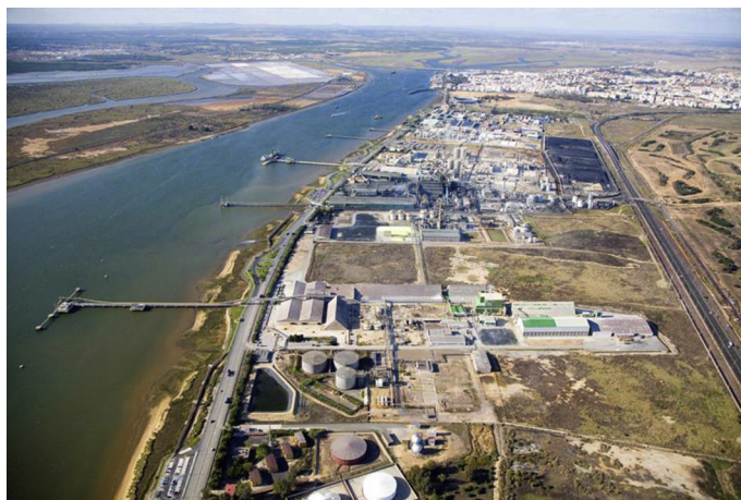
Figure 5.5 Processing and use of naturally occurring radioactive material (NORM) (pictured: phosphate processing plant, S Spain (García-Tenorio, 2010)).
