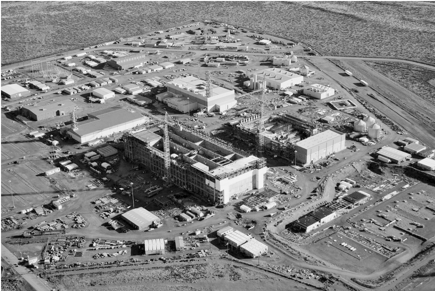
4.1 Waste Treatment Plant under construction, Hanford, Washington, 2012.
