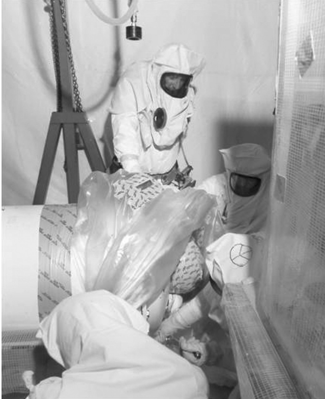
11.3 Size reduction of gloveboxes in building 771 (once known as the most contaminated building in America).
