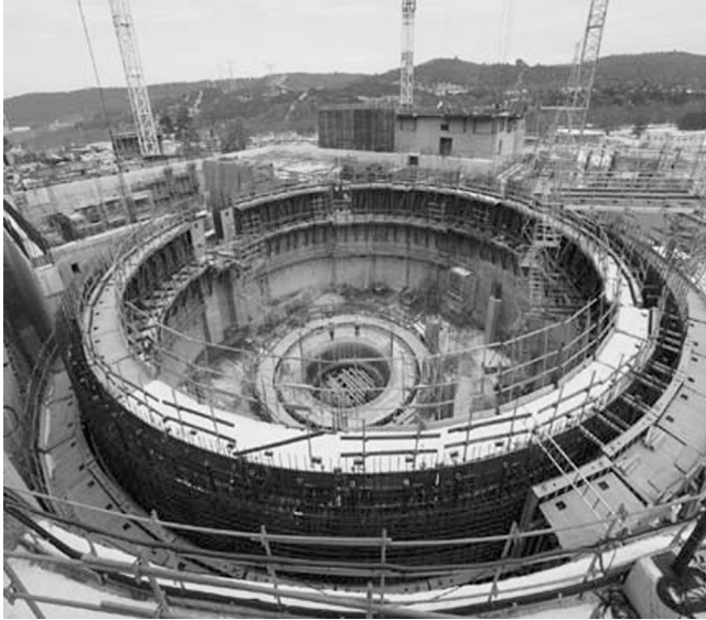
7.4 Reactor containment building under construction, February 2012 (photo courtesy of CEA).
