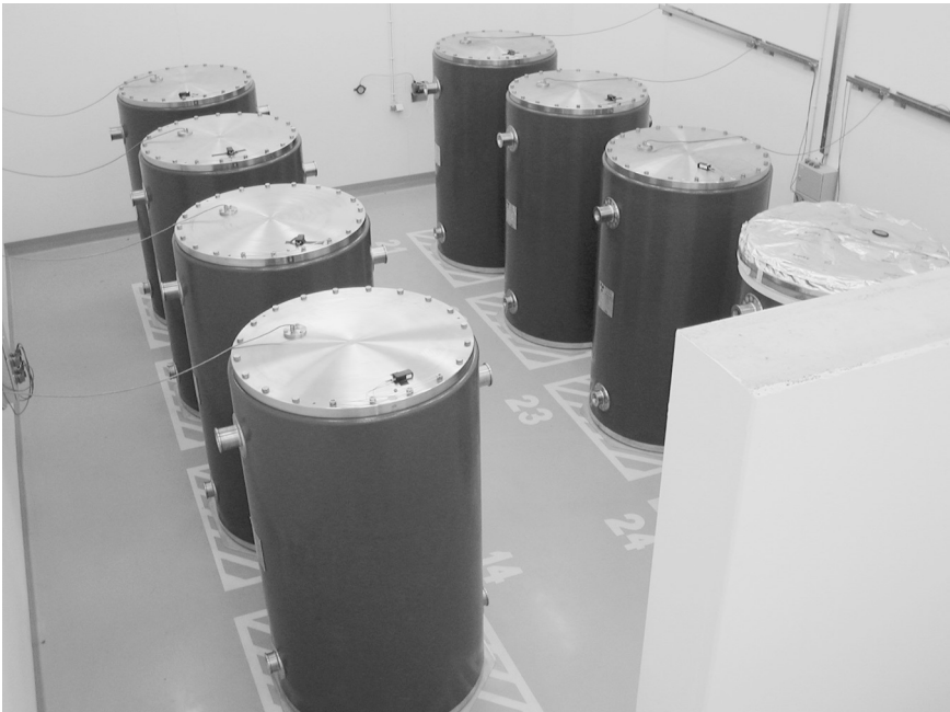
9.2 Loaded CASTOR casks in dry storage.
