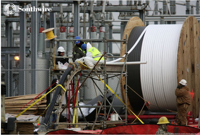
Figure 5.13 HTS Triax™ cable installation at the AEP Bixby substation. The white cable on the drum is the superconductor and dielectric portion being fed into the black cryostat and outer jacket of the final cable. The cryostat and outer jacket were already placed in a below-ground trench at the substation. The cable will be connected to the above-ground terminations in the background (Demko et al., 2007).
