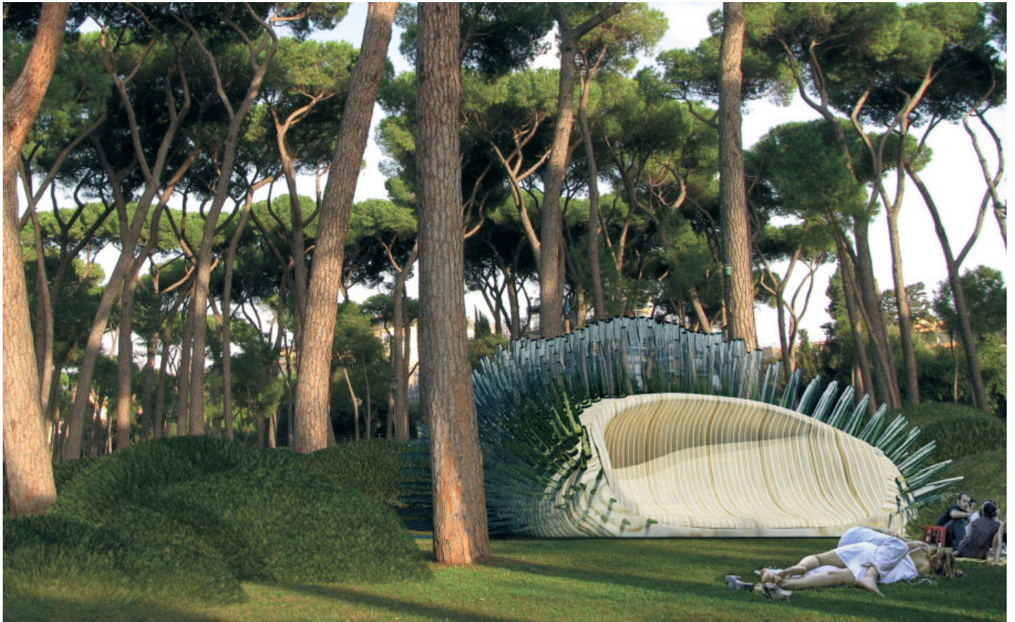
The kiosk and the two pavilions designated for storage and toilets, and wi-fi, are three more hills in the public space defined by operations of stretching the surface; but these hills are built with wood instead of land. The construction system is based on wooden dowels consisting of flat sections cut by CNC. The exterior is modelled with a three-axis milling machine of assembled sections, while the interior sections are offset to prevent surface milling.
