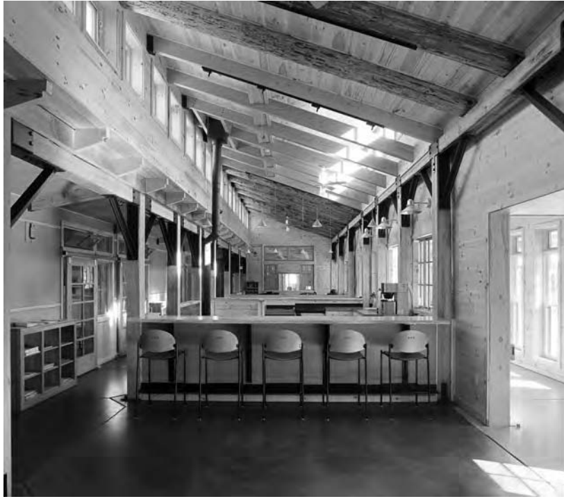
Fig. 3.43 Administrative center of the Aldo Leopold Legacy Center, with clerestories and daylight zoning throughout the building—strategies that helped to reduce the use of electric lighting. (© The Kubala Washatko Architects, Inc.; used with permission.)
