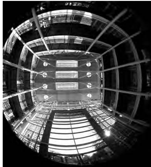
Fig. 29.24 Fisheye view of the Lillis Business Complex atrium. The south-facing panels of the rectangular skylights also contain embedded PV cells. (Photo © 2004 by Alison Kwok; all rights reserved.)
