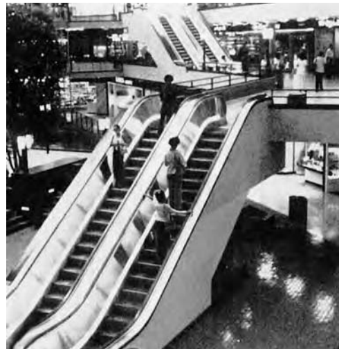
Fig. 33.14 Stair lighting is supplied by a continuous fluorescent strip at the base of the balustrade in this California shopping mall. (Photo courtesy of Montgomery-KONE.)
