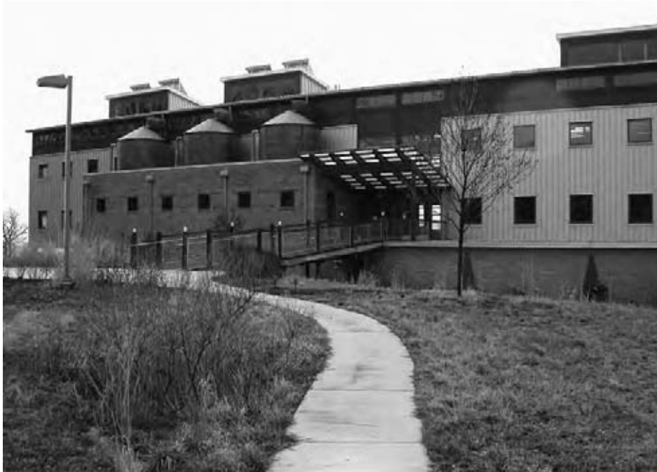
Fig. 2.13 North (inland) façade of the Philip Merrill Environmental Center showing the visual impact of rainwater collection intent and solution. Water conservation has informed this façade. (Photo © 2004 Walter Grondzik; all rights reserved.)
