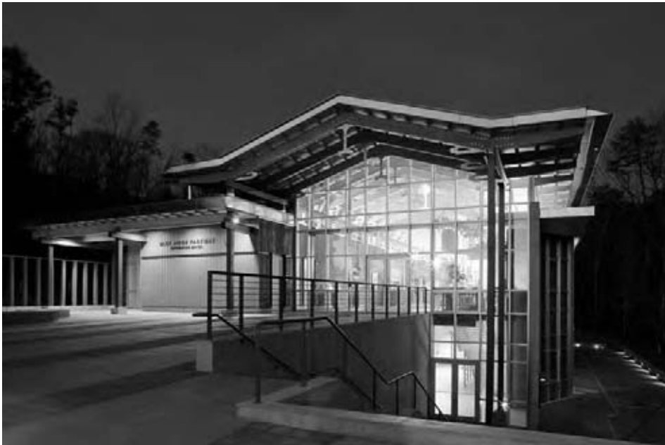
Fig. 8.59 Blue Ridge Parkway Destination Center near Asheville, North Carolina. (© Jonathan Hillyer Photography, Inc.; used with permission.)
