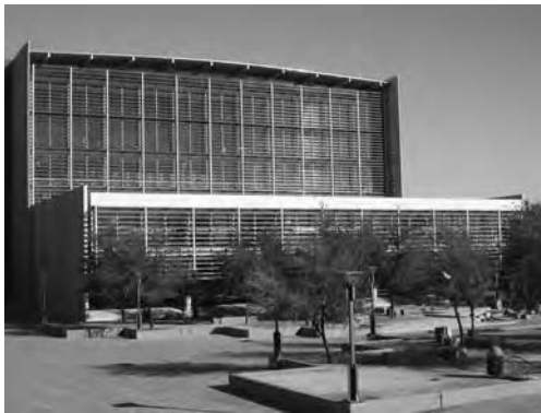
Fig. 14.11 Fixed horizontal louvers on the south façade at the Phoenix Public Library, Phoenix, Arizona. (Photo © 2004 by Walter Grondzik; all rights reserved.)
