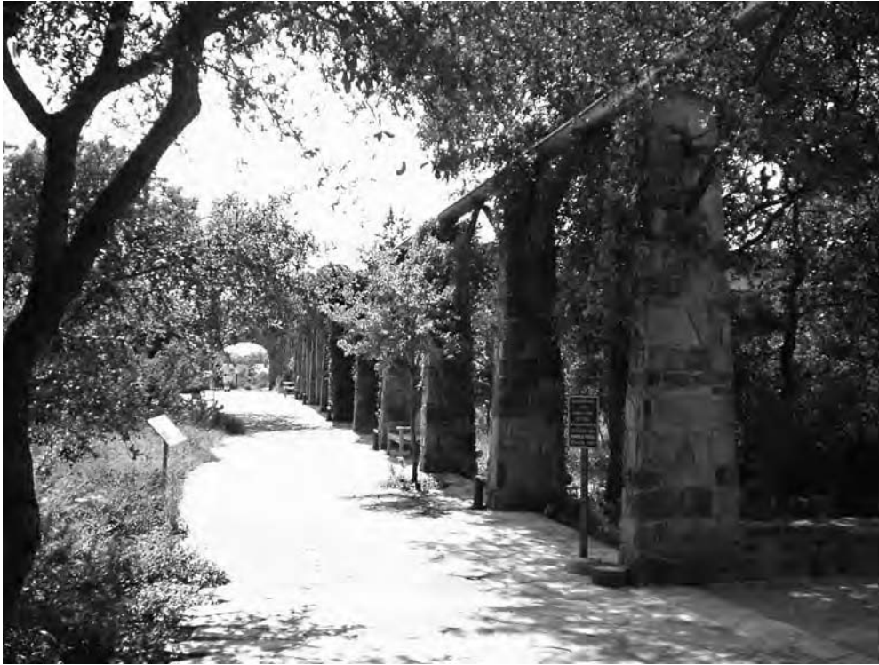
Fig. 20.31 Rainwater harvesting system on locally-sourced stone arches along the entry path surrounded by oak trees. (Photo © 2009 Alison Kwok; all rights reserved.)
