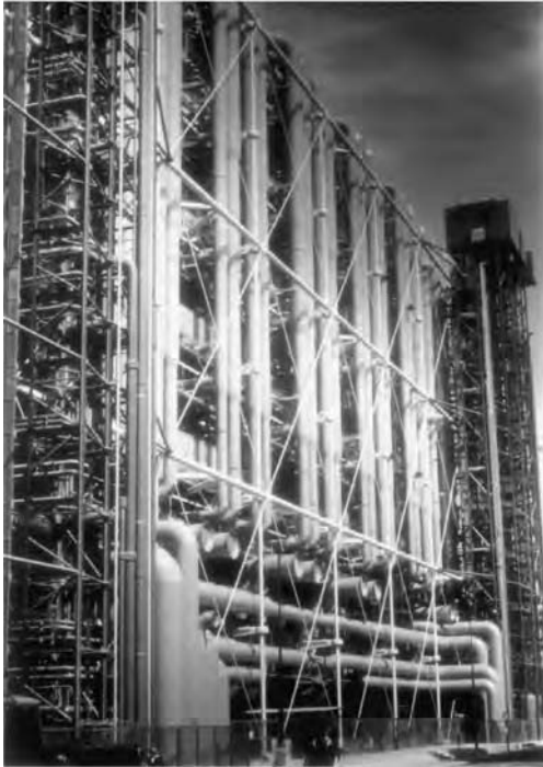
Fig. 10.7 Centre Georges Pompidou, Paris. A view of the mechanical support systems. Piano + Rogers, architects. (Photo by John Tingley.)
