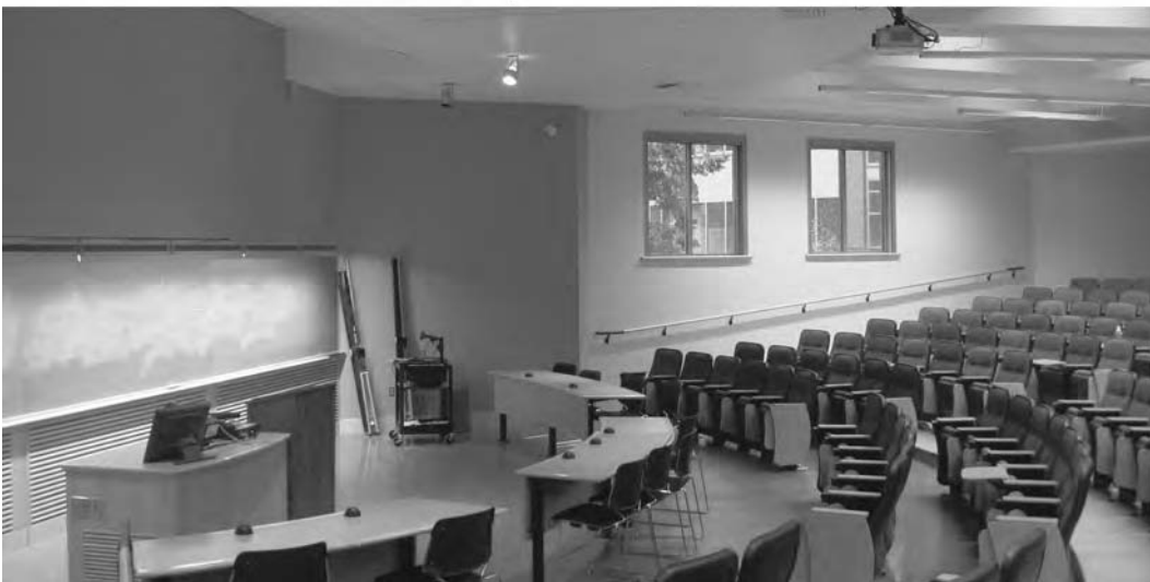
Fig. 16.12 Typical lecture room lighting utilizes 45° cutoff baffled parabolic reflector troffers for minimum direct and reflected glare, adjustable track lights for demonstration table illumination, and an asymmetric reflector for chalkboard lighting. The large display area on the front wall of the room will not experience veiling reflections with the illustrated lighting arrangement.
