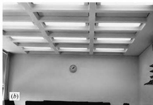
Fig. 16.22 A coffer-ceilinged room (a) is illuminated with 1 \times 4 ft ( 0.3 \times 1.2 m) two-lamp units in alternate coffers. The appearance both unlighted (a) and lighted (b) is symmetrical. (Photos by B. Stein.)
