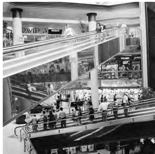
Fig. 33.20 Unusual angular design of multiple ramps in a shopping mall in Brisbane, Australia. The use of ramps rather than escalators permits shopping carts and bulky packages to be moved with ease between the building levels. (Photo courtesy of O&K Rolltreppen, Germany.)
