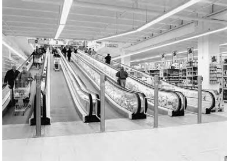
Fig. 33.21 Multiple inclined ramp installation in a European department store (three up, two down). Of interest in this installation are the level entries, lighted balustrades, the ease with which shopping carts are handled on the wide pallet, and the use of the space between the transparent balustrades for merchandising. (Photo courtesy of O&K Rolltreppen, Germany.)
