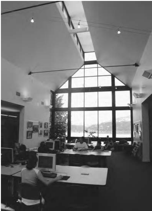
Fig. 1.16 Seek common solutions. The “atrium” of the Hood River County Library, Hood River, Oregon, provides a central hub for the library, daylighting, views (spectacular), and stack ventilation. (Photo © 2004 Alison Kwok; all rights reserved.)
