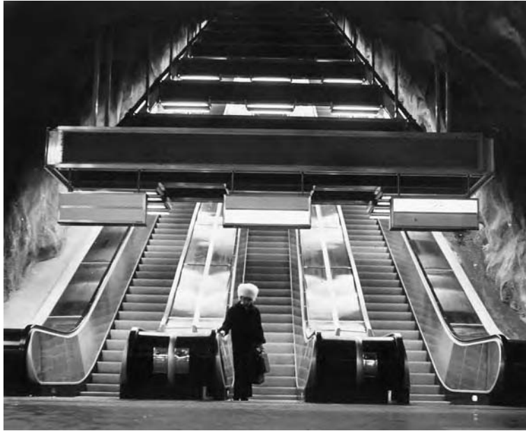
Fig. 33.9 Among the longest moving stairways in Europe are those installed in the Stockholm subway system. This parallel bank of three escalators is 230 ft (70 m) long with a 108-ft (33-m) rise. Unlike American standards of 30° incline, 100-fpm (0.51-m/s) speed, and 32- or 48-in. (0.81- or 1.22-m) size, these units are at 27.3° incline, 147.6-fpm (0.75-m/s) speed, and 40-in. (1.02-m) width. (Photo courtesy of O&K Rolltreppen, Germany.)
