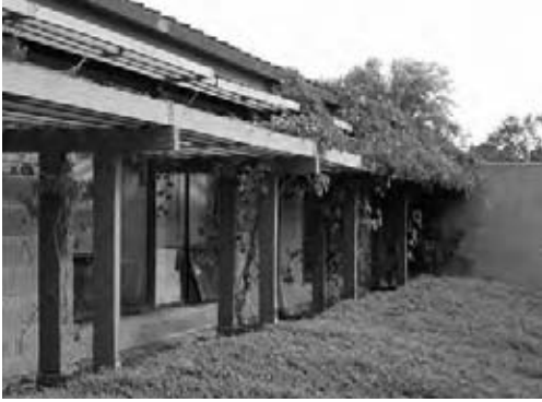
Fig. 7.1 The envelope is more than a surface. This south-facing office façade in Oregon forms a microclimate zone that buffers the transition between indoor and outdoor conditions. Groundcover plants at eye level for seated occupants and deciduous vines overhead give a seasonally changing view to the outdoors through a façade that also admits winter sun, year-round daylight, and summer breeze. (Photo by Amanda Clegg.)
