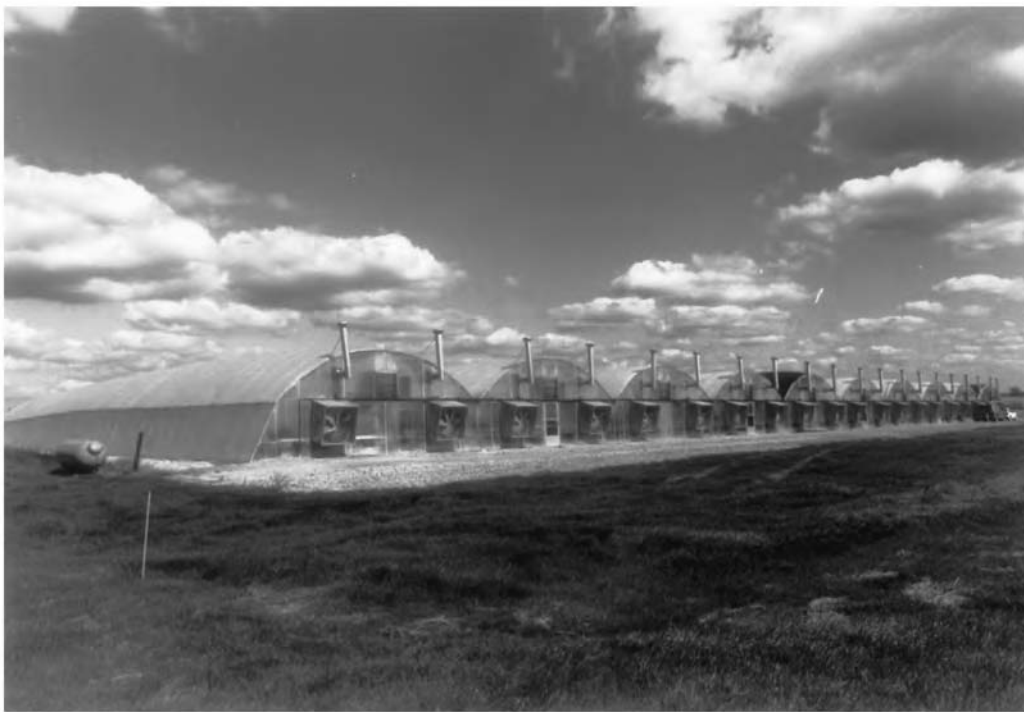
Fig. 23.2 A 45,000-ft 2 (4180-m 2 ) greenhouse built over part of a 70-acre (28-hectare) Michigan landfill utilizes "landfill gas" (including about a 65% methane component) both to fuel space heaters and to generate electricity for lighting. Waste heat from the generator also contributes to space heating. (Photo by George P. Graff. Courtesy of Willow Run Farms, Inc., Ypsilanti, MI.)
