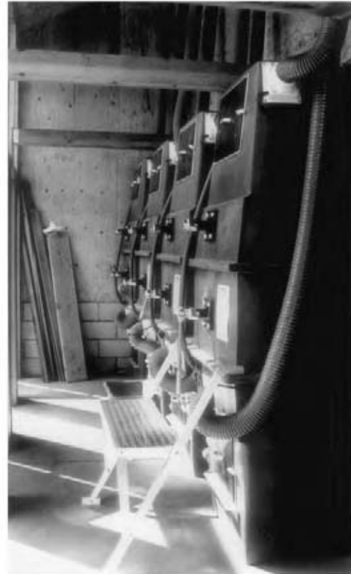
Fig. 22.5 The Phoenix composting toilet's tank serves either two toilets or one toilet and one food waste inlet. (a) Schematic section; rotatable tines mix waste and control the movement of compost to the access area for eventual removal. The fan exhausts air from the Phoenix tank to control odors. Passing behind the air baffles, air makes frequent contact with the compost pile, ensuring aerobic decomposition. After passing through the compost pile and receiving secondary treatment in the bottom of the Phoenix, liquid is periodically sprayed on top of the compost pile to keep the pile moist and inoculate fresh waste with decomposing organisms. Each tank is 39 in. (1000 mm) wide and 61 in. (1550 mm) long, and requires another 5 ft (1525 mm) in front for maintenance access, and is available in three heights: 55 in. (1400 mm), 73 in. (1850 mm), and 92 in. (2350 mm). Another 12 in. (300 mm) above the top of the tank is convenient for maintenance. (b) Four chambers with their rotatable tines serve the Vogelsang High Sierra Camp at Yosemite National Park, California. (Courtesy of Advanced Composting Systems, Whitefish, MT.)
