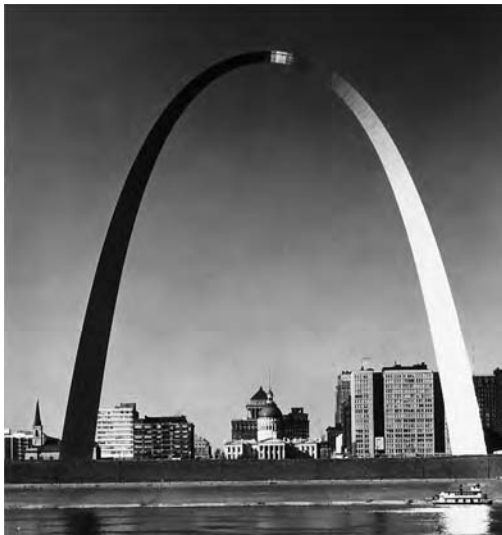
Fig. 32.10 The St. Louis Gateway Arch has a 10-passenger inclined elevator in each leg. Placement of doors, arrangement of the counterweight, and size of the shaft all depend upon the angle of incline. The car moves 82 ft (25 m) horizontally during its 386 ft (118 m) of total travel at an incline of approximately 12^\circ . (Photo courtesy of Bethlehem Steel Corporation, which supplied the elevator rope for this installation.)
