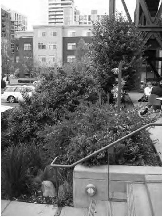
Fig. 20.10 Bioswale at the EcoTrust building in Portland, Oregon, captures storm water runoff from the green roof of the building and other surfaces. (Photo by Nathan Majeski.)
