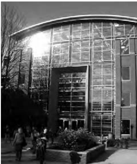
Fig. 29.20 South façade of the Lillis Business Complex, Eugene, Oregon. The atrium glazing incorporates PV cells in a recent example of building-integrated PVs. (Photo © 2004 by Alison Kwok; all rights reserved.)
