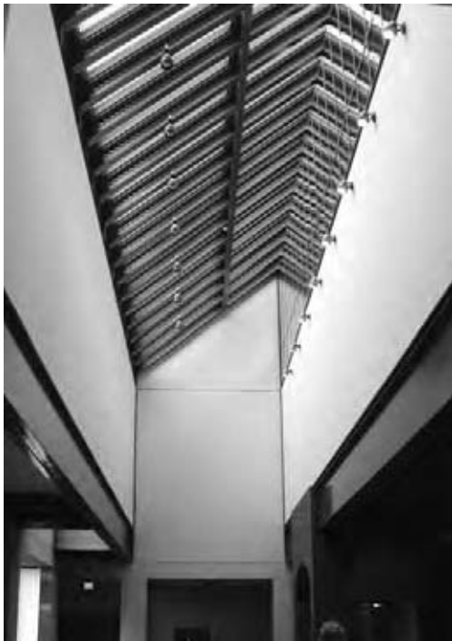
Fig. 14.15 Clerestory skylights with louvers at the U.S. Holocaust Memorial Museum in Washington, DC (Pei, Cobb, Freed & Partners, 1993). (Photo © 2004 by Alison Kwok; all rights reserved.)
