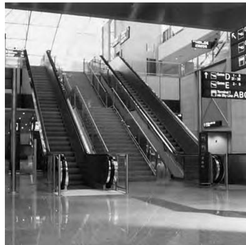
Fig. 33.8 Escalators in transportation terminals are subject to periods of very heavy use. To avoid crowding at the entrance to the up (left) moving stair, the balustrade is effectively extended with a glass-sided divider. Passengers on the down (right) escalator are guided by large overhead signs and a standing sign at the base and balustrade extension to avoid hesitation and bunching. Note also the large open area in front of both units. (Photo courtesy of O&K Rolltreppen, Germany.)
