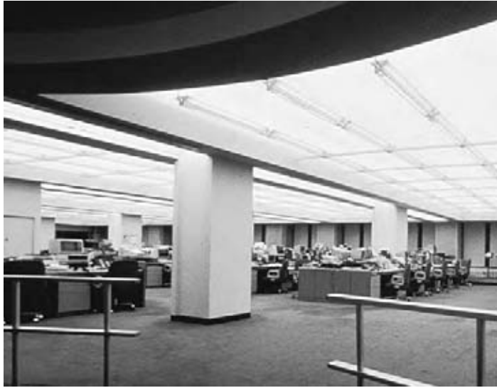
Fig. 16.18 Semi-indirect lighting installation in a New York stock brokerage office utilizing the fixture shown in Fig. 16.17. Every desk is equipped with a VDT. The translucent sides of the fixture are within the acceptable 5:1 luminance ratio to the ceiling recess luminance and therefore should not create a reflected glare problem. (Courtesy of Zumtobel-STAFF Lighting Co.)
