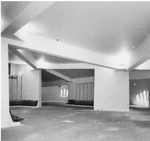
Fig. 16.10 Schools frequently utilize spaces for multiple functions. This space, normally used as a dining area, doubles as an assembly room. High-intensity, indirect tungsten-halogen units, tucked into concrete beam junctures, provide sufficient light for both uses.
