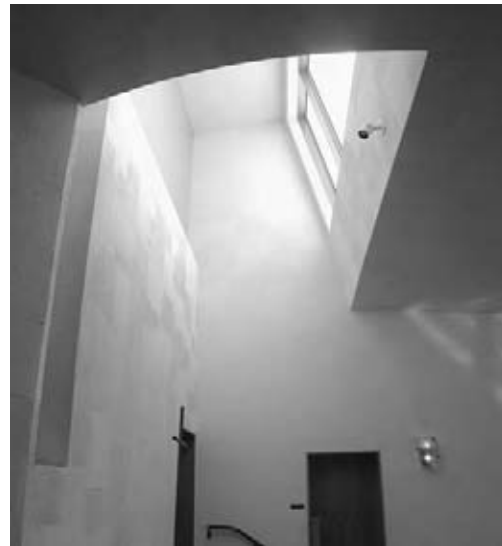
Fig. 14.13 (a) A skylight near a north wall provides reflecting surfaces for uniform light distribution and reduces the potential for glare. (b) One of the "bottles" of light (skylight) at St. Ignatius Chapel at Seattle University in Seattle, Washington (Steven Holl, 1995). (Drawing by Erik Winter; photo by Alison Kwok; © 2004 Alison Kwok; all rights reserved.)
