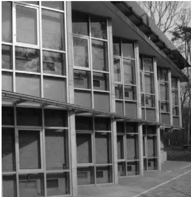
Fig. 8.61 South-facing, sawtooth Trombe wall with shading to prevent overheating in the summer. (© Lord, Aeck & Sargent, Inc.; used with permission.)
