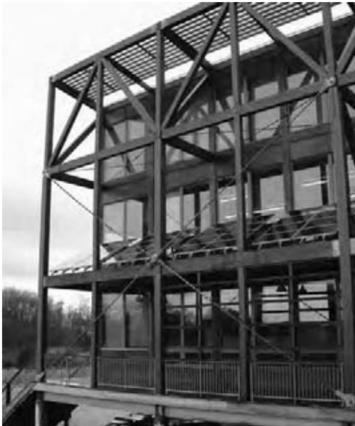
Fig. 2.14 South (bay side) façade of the Philip Merrill Environmental Center showing PV panels, daylighting/solar apertures, and shading elements. Energy collection has informed this façade. (Photo © 2004 Walter Grondzik; all rights reserved.)
