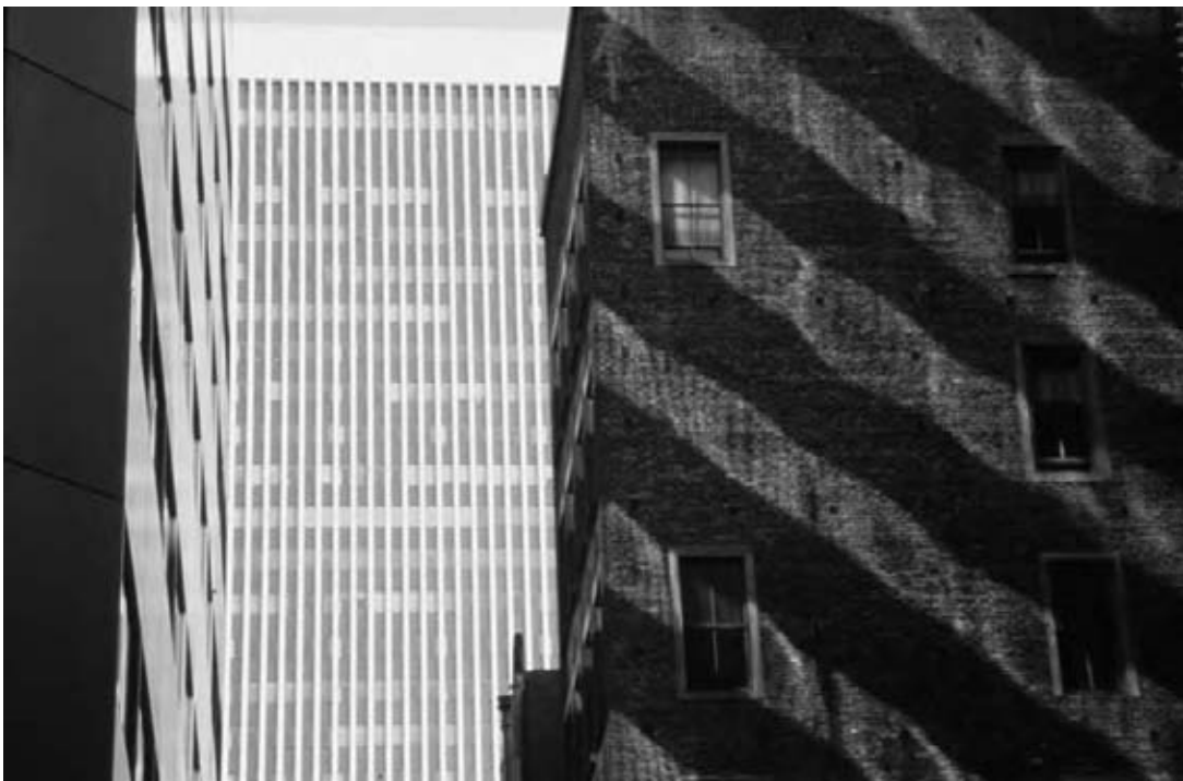
Fig. 3.17 Mirror-glass windows in a newer office building (left) in San Francisco, California, cast strong reflections on the north- and west-facing walls of an older building next door. Although this reflected radiation/heat might be welcome in winter, the resulting glare can be intense. In summer, the older building is particularly disadvantaged by additional thermal loads. (© 2009 Alison Kwok; all rights reserved.)
