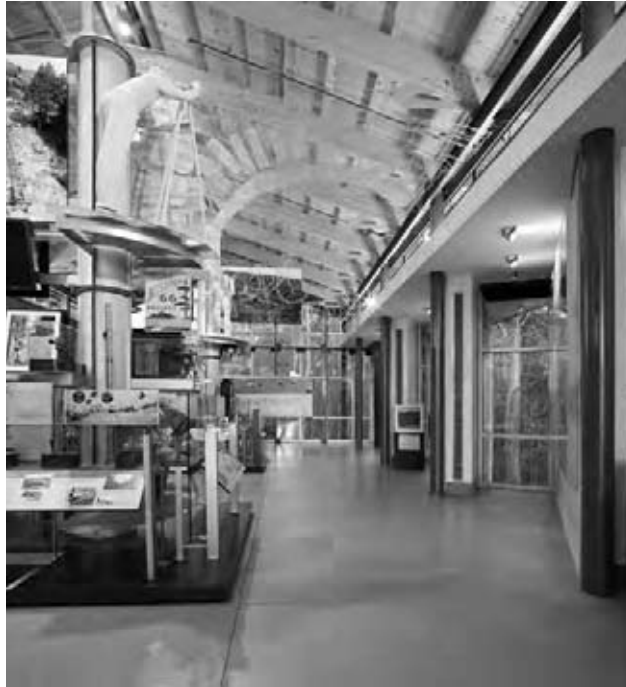
Fig. 8.62 Exhibit space along the Trombe wall; note supply vents in the edges of the Trombe wall. (© Jonathan Hillyer Photography, Inc.; used with permission.)
