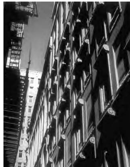
Fig. 24.5 Rolling metal shutters, housed in valences above each window, punctuate the exterior of this downtown Pittsburgh building opening onto a narrow street. The shutters can protect the building's contents from an exterior fire, but can also protect the narrow street from a fire inside the building. Note the exterior fire escapes across this narrow street. These are no longer permitted, partly because smoke plumes rising from windows can make such stairs unusable long before heat from a fire becomes a threat.
