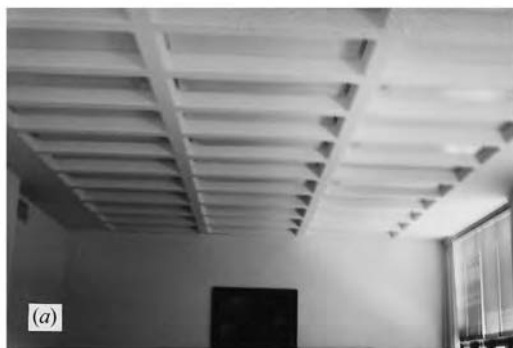
Fig. 16.22 A coffer-ceilinged room (a) is illuminated with 1 \times 4 ft ( 0.3 \times 1.2 m) two-lamp units in alternate coffers. The appearance both unlighted (a) and lighted (b) is symmetrical. (Photos by B. Stein.)
