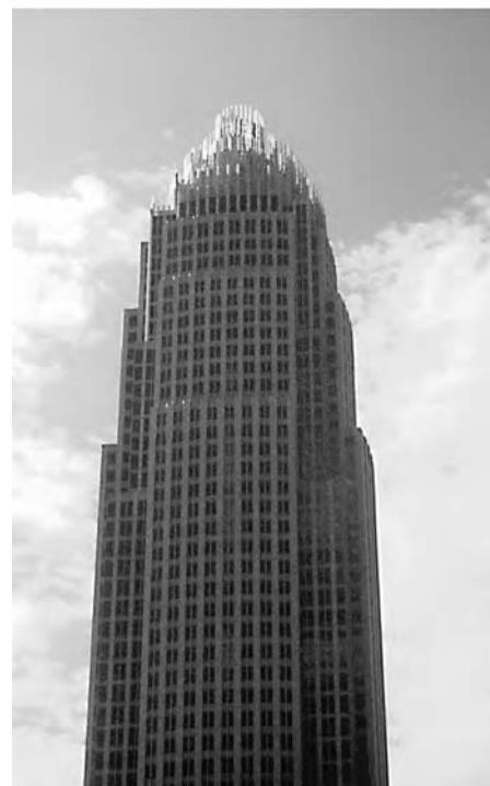
Fig. 24.31 Lightning rods (air terminals) enliven the silhouette of the Bank of America Corporate Center in Charlotte, North Carolina. (Photo by Dale Brentrup.)
