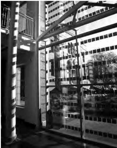
Fig. 29.23 View from the atrium of the Lillis Business Complex; the integrated PV cells provide partial shading and a lively lighting pattern. (Photo © 2004 by Alison Kwok; all rights reserved.)
