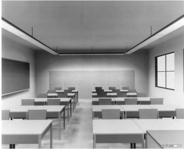
Fig. 16.7 Computer-generated image of a 24-ft-W × 28-ft-L (7.3-m by 8.5-m) classroom using a perimeter layout of 16.4-ft (1.2-m) luminaires in a 14-ft × 22-ft (4.3-m by 6.7-m) rectangle suspended 18 in. (457 mm) from the ceiling and 9 ft (2.7 m) above the finished floor (AFF). The luminaires use T8 triphosphor lamps and high-frequency electronic ballasts. Average horizontal luminance on the desks is 74 fc (800 lux), and average vertical luminance on the chalkboards is 39 fc (420 lux). Room power density is 1.8 W/ft 2 (19 W/m 2 ). (Courtesy of Zumtobel-STAFF Lighting Co.)
