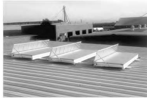
Fig. 21.8 A solar still can be used to provide a small daily quantity of pure water; this installation serves a laboratory. (Courtesy of McCracken Solar Co., Alturas, CA.)
