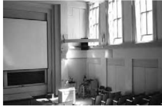
Fig. 14.5 (a) With higher windows, daylight extends farther into a space. (b) High windows in a classroom at the University of Oregon. (Drawing by Erik Winter; photo by Nathan Majeski.)
