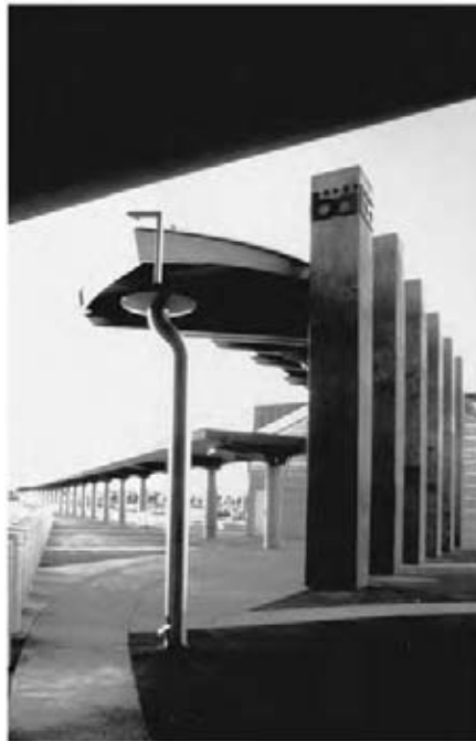
Fig. 20.24 A downspout terminates the roof with flair at the Pleasanton BART (Bay Area Rapid Transit) station near San Francisco. (Photo by Jane Lidz.)
