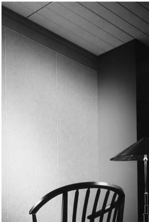
Fig. 19.8 Acoustic wall panel consists of a rigid backing covered with either mineral fiber or fiberglass and finished with any of a wide selection of fabrics. NRC averages 0.6 for mineral fiber substrate and 0.8 for fiberglass for contact mounting (A mounting) and 0.7/0.9 when the panels are mounted on 2-cm (nominal ¾-in.) furring strips (D-20 mounting). The latter mounting is particularly effective in increasing absorption below 500 Hz. (Photo courtesy of Armstrong World Industries.)
