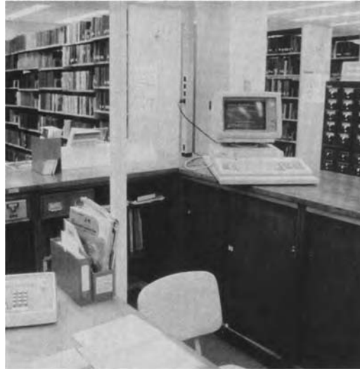
Fig. 27.45 Power poles extend down from the ceiling to any desired height. In this library, power is required above the base cabinets, and the power pole is easily arranged to supply it. (Courtesy of Wiremold Company.)
