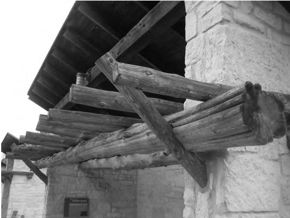
Fig. 20.32 Wood was reused from the site to create overhangs and trellises. (Photo by Jake Moore; © 2009 Alison Kwok; all rights reserved.)
