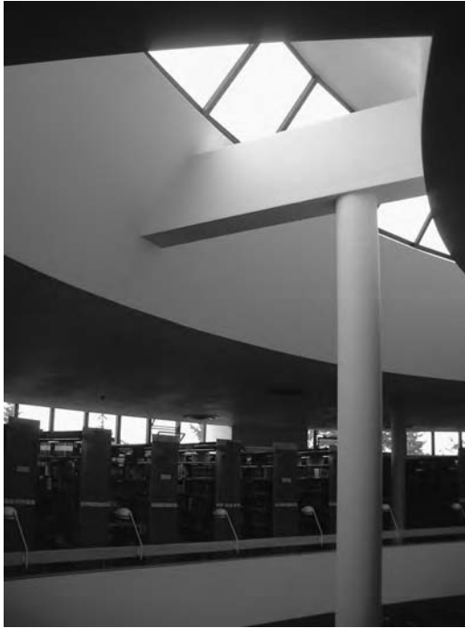
Fig. 1.13 Letting nature do the work—via daylighting. Mt. Angel Abbey Library, St. Benedict (Mt. Angel), Oregon, designed by Alvar Aalto. (Photo by Amanda Clegg.)
