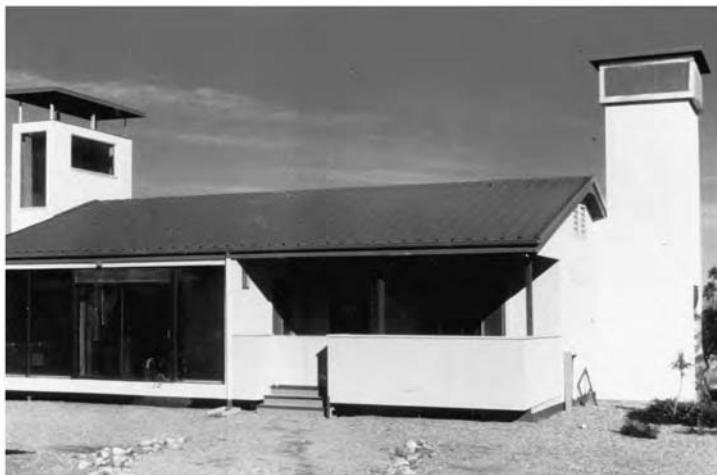
Fig. 8.19 An experimental residence in Tucson, Arizona, is passively and evaporatively cooled by a cooltower (at the right in the photograph). Hot, dry air passes through the wetted pads at the tower's top and undergoes a drop in DB temperature that causes it to fall, entering the residence at the bottom of the tower. The tower at the left is a solar chimney to help speed the flow of warmed exhaust air.
