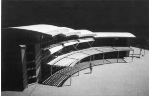
Fig. 1.6 Scale model analysis of shading devices for the Real Goods Solar Living Center. This is the sort of detailed analysis that would likely occur during schematic design. (Photo, model, and analysis by Adam Jackaway; reprinted from A Place in the Sun with permission of Real Goods Trading Corporation.)
