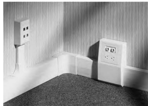
Fig. 27.19 Three-section nonmetallic baseboard-type raceway measures 4 in. H and 1.5 in. D (100 × 38 mm). The three sections are intended for telephone, power, and data cabling. The junction box on the right protrudes so as not to lessen the raceway wiring space. It is equipped with vertical dividers to keep the three types of wiring completely separated. The elevated wall box on the left contains telephone and data cable outlets and connects only to the low-voltage portions of the raceway. (Photo courtesy of Hubbell, Inc.)
