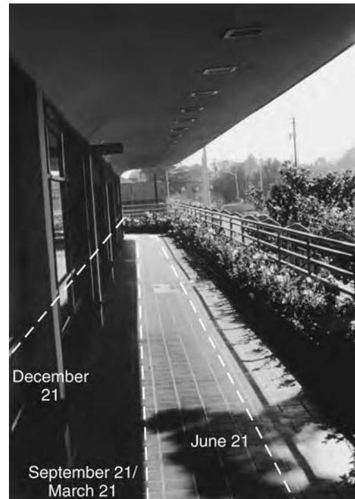
Fig. 3.37 Fixed overhang sun control. This south-facing exterior corridor in Oregon is open to the air year-round. Low winter sun fills the corridor, and some of its heat is stored by the tile floor. In cold weather, however, the offices connected by the corridor are disadvantaged by unbuffered exposure to cold air. In summer, little of the corridor is exposed to sun, improving comfort. Sun control is identical in the (cool) spring and (warm) fall with such fixed shading.
