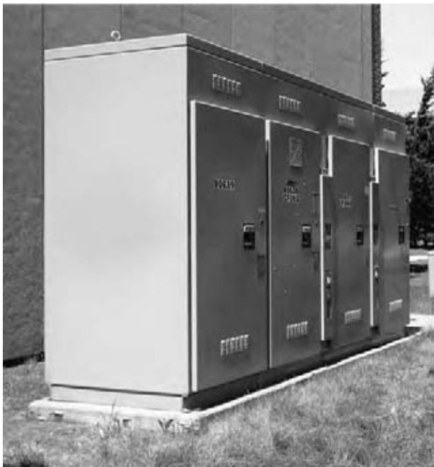
Fig. 26.27 Four-bay (section), power-operated, high-voltage service entrance switchgear rated 13.8 kV, consisting of (see the single-line diagram inset, and reading from left to right) a fused feeder section, two bays with parallel incoming lines and automatic transfer in the event of power failure, and a second switch and fuse feeder section. Fuses are electronic, with circuitry designed to provide a trip signal when excessive current is sensed, rather than simply relying on the thermal characteristic of a fusible element. This gear, which measures 93 in. H × 172 in. W × 44 in. D (2.4 × 4.4 × 1.1 m) and weighs 8000 lb (3630 kg), is suitable for interior or exterior installation. (Courtesy of S&C Electric Co.)
