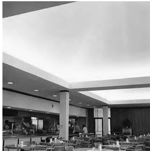
Fig. 16.11 Institutional cafeteria illuminated by cove lighting in a deep pyramidal coffer. Lighting is even, glare-free, soft in quality, and pleasant, yet of sufficient intensity to permit using the cafeteria as a working-meeting space. (Photo by B. Stein.)
