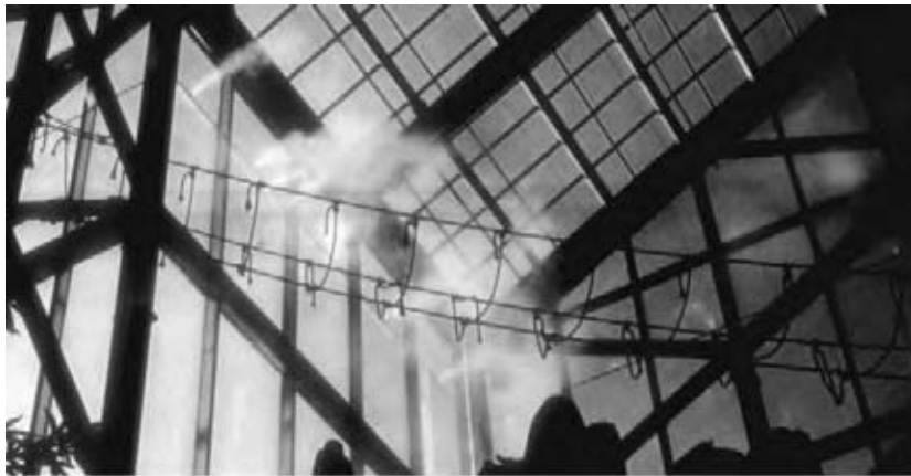
Fig. 10.52 With more glass area than floor area, the Frederick Meijer Conservatory near Grand Rapids maintains a tropical environment in Michigan's winter. (a) A perimeter tunnel delivers air evenly around the walls, heated by finned tubes just above the planting level. (b) A separate "wind" system provides a continuous breeze from diffusers in the vertical ducts to strengthen plants' root systems. (c) A fogging system maintains tropical humidity while adding evaporative cooling under summer conditions. (Photos by Roger Van Vleck; courtesy of Fishbeck, Thompson, Carr & Huber, Ada, MI.)
