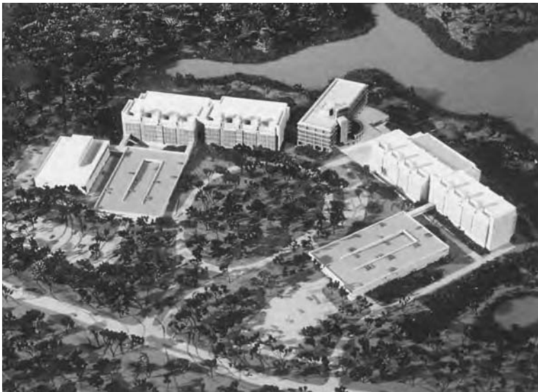
Fig. 5.2 The campus of the U.S. Environmental Protection Agency at Research Triangle Park, North Carolina, features concentrated parking separate from the buildings. High exhaust stacks disperse air from laboratories; intakes are kept well away from exhaust. (Courtesy of Hellmuth, Obata + Kassabaum, Washington, DC.)
