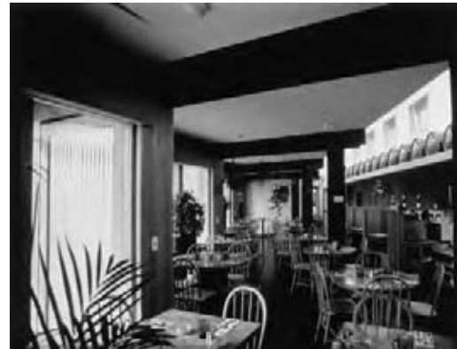
Fig. 1.21 Manage storage. A concrete floor and barrels located high along the north wall provide thermal storage (for both heating and cooling) in the Cottage Restaurant, Cottage Grove, Oregon. (Photo by G. Z. Brown.)
