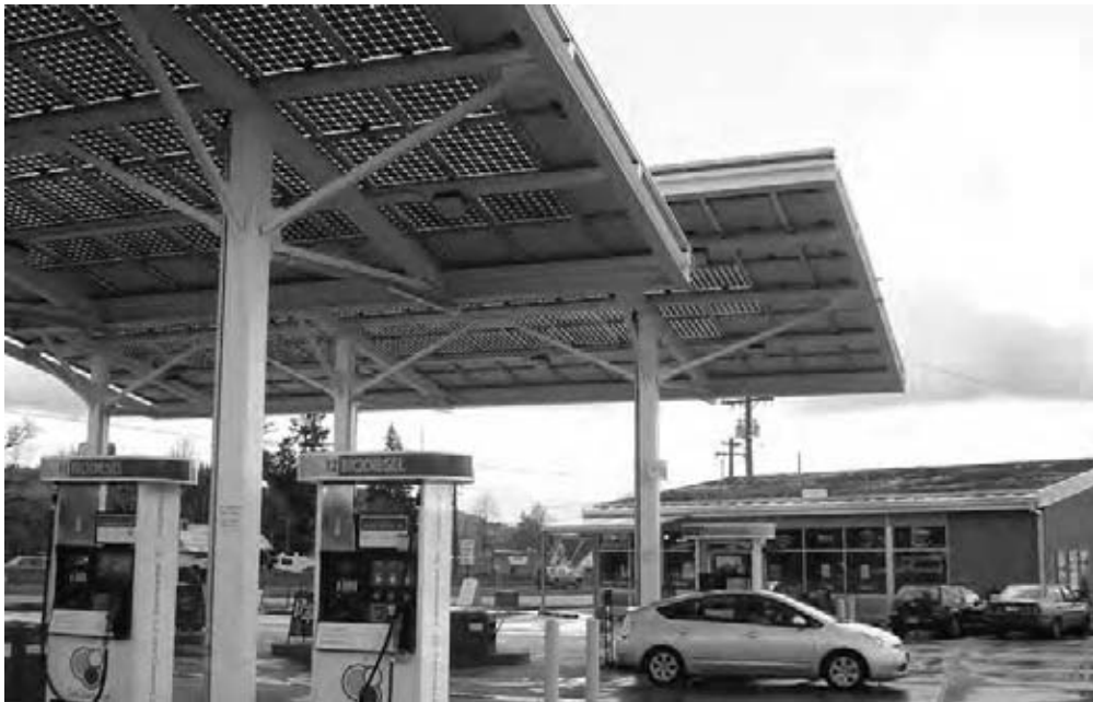
Fig. 2.8 “Building” integrated photovoltaics (BIPV) provide shelter, shading, and power for a fueling station/convenience store in Eugene, Oregon. Note the green roof on the store and the biofuel pumps. (Photo by Nathan Majeski.)
