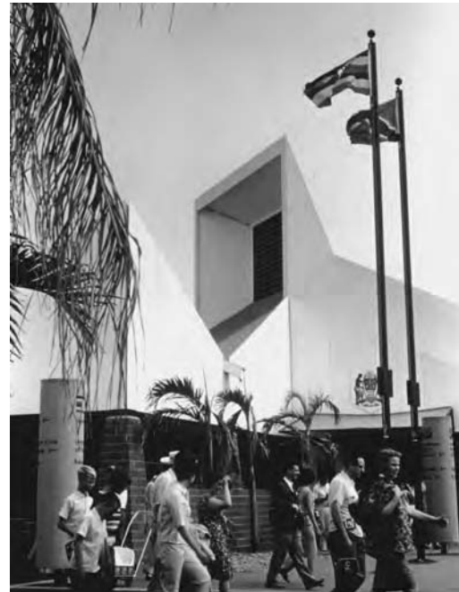
Fig. 3.31 Cooling with the wind. The air inside this exhibition hall is heated by lights and crowds of people. It rises via the stack effect and is sucked out of the large clerestory opening by the prevailing winds. Note that winds do not blow into this high opening but create a negative pressure outside the opening, encouraging an outward flow of air from the exhibition space. (African Place at Expo '67, Montreal, Canada; John Andrews, architect.)
