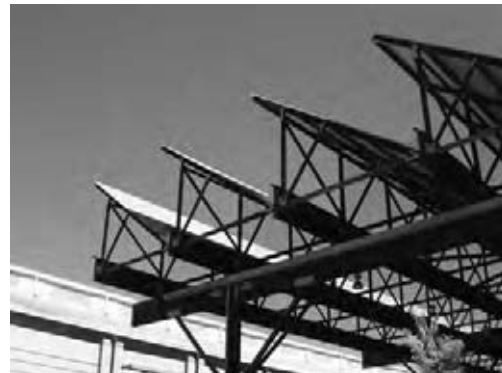
Fig. 3.35 This roof over a covered outdoor tennis facility at the University of Oregon, Eugene, was designed to ward off rain-bearing south winds in winter. Direct glare from the sun is also unwelcome; instead, north skylight is admitted along with reflected light from roof surfaces. Gutters at the lower edge of each roof plane carry away rainwater; the courts stay dry for all but a few days each year. (Unthank Seder Poticha Architects. Photo by Amanda Clegg.)
