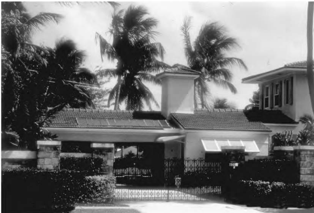
Fig. 21.26 Solar water heaters are widely used. This house in Miami, Florida, incorporates a storage tank above the collector, which is enclosed in the chimney-like form. This permits passive (thermosiphon) circulation without a pump. (Photo by M. Steven Baker.)
