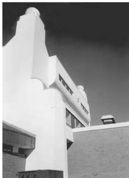
Fig. 5.7 Two wind-gravity (turbine) ventilators accent the skyline of the addition to Barton Hall at the University of New Hampshire. These draw hot exhaust air from the auditorium; cool outdoor air is admitted through low windows and shutters in the auditorium's north wall. (Courtesy of Banwell White Arnold Hemberger & Partners, Inc., Hanover, NH.)
