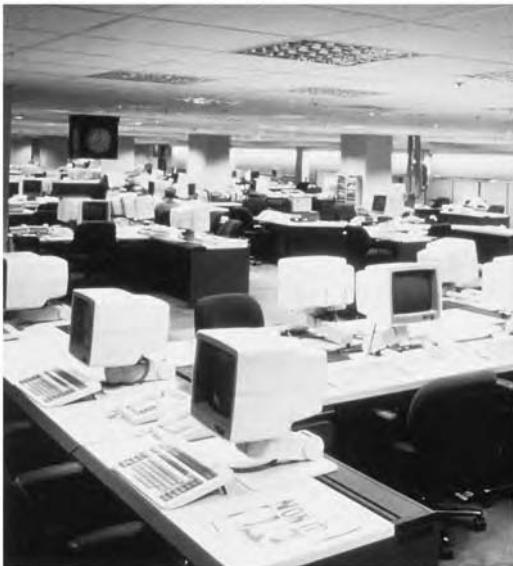
Fig. 16.20 The illustrated installation shows a newspaper office with a VDT on every desk and a variety of viewing directions. The lighting fixtures utilized are deep-cell specular parabolic louver units, which typically have low surface brightness and crosswise batwing distribution. Note particularly that the VDT screens are deeply recessed into the monitor case to minimize glare and that each VDT is mounted with tilt and swivel capability. (Courtesy of Zumtobel-STAFF Lighting Co.)
