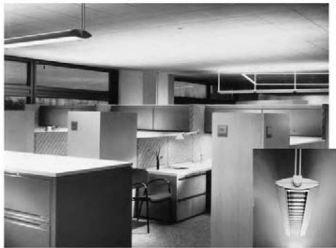
Fig. 16.19 A direct-indirect luminaire (see insert) with batwing uplight distribution can be used in a space with ceilings as low as 9 ft (2.7 m) and even less, without excessive ceiling brightness, as shown in this open-plan landscaped office. (Courtesy of Zumtobel-STAFF Lighting Co.)
