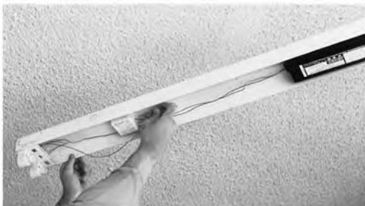
Fig. 15.26 This type of compact solid-state electronic circuit reduces ballast power input by approximately 30% and lamp output by about 28%, resulting in a net gain in efficacy. The power factor remains above 90%. Similar units are available for larger power decrease. They can be mounted on the lamp end or in the fixture channel, as shown. An ancillary benefit is cooler ballast operation, resulting in extended life. (Photo courtesy of Remtec Systems.)
