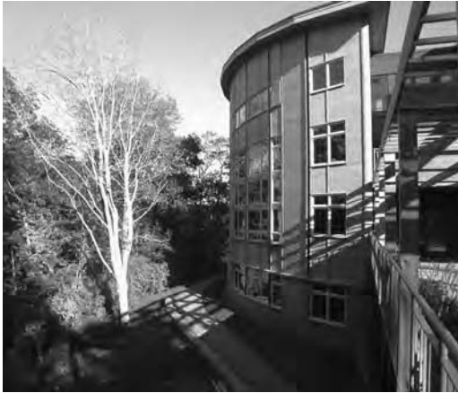
Fig. 1.26 Exterior photo of the completed and occupied WHRC. (Photo © Alison Kwok; all rights reserved.)
