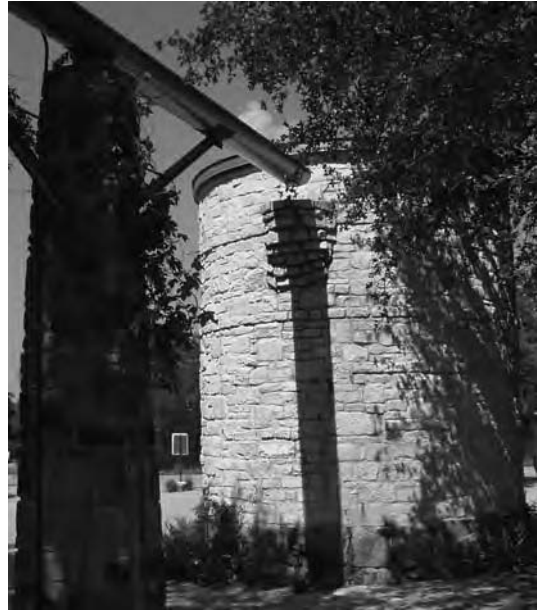
Fig. 20.29 Entry cistern fed by aqueducts from the site's rain-water harvesting system. (Photo © 2009 Alison Kwok; all rights reserved.)
