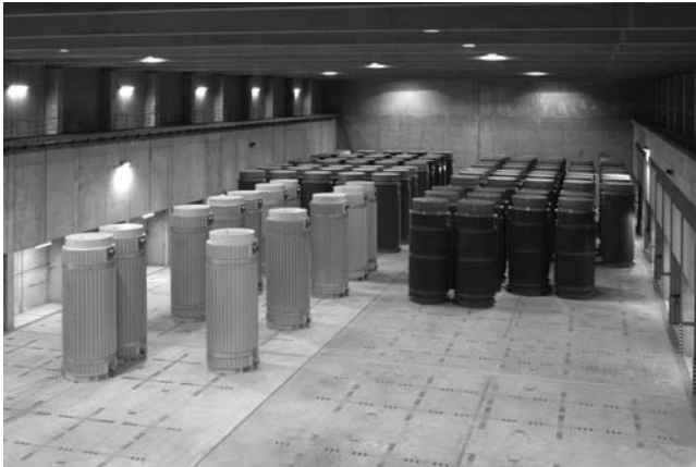
14.6 Storage of spent nuclear fuel in dry storage casks (Gorleben, Germany).
