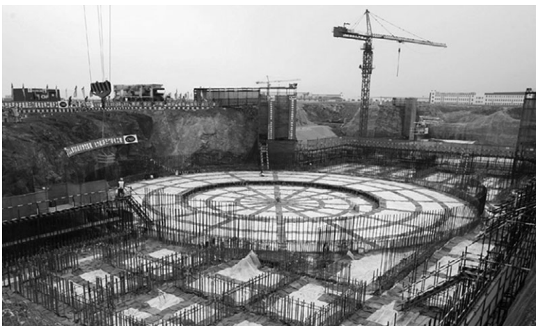
9.1 Advanced concrete mixing and pouring at Sanmen 1 (China).
