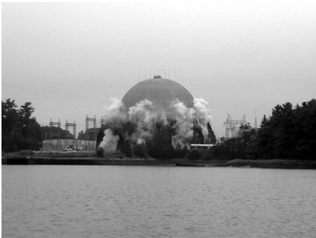
24.6 Maine Yankee containment building demolition.
