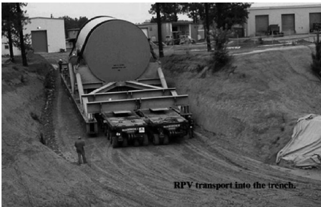
24.4 Maine Yankee reactor vessel disposal.
