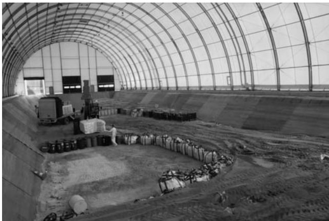
14.16 Disposal of very low-level waste at the disposal facility for very low-level waste at Morvilliers, France (© Emmanuel Gaffard).
