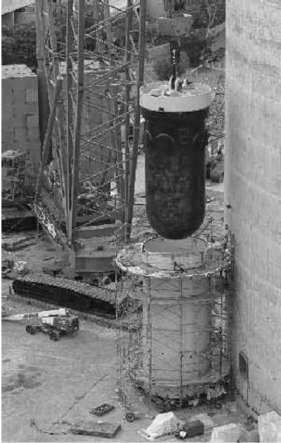
24.2 San Onofre Unit 1 reactor vessel removal.
