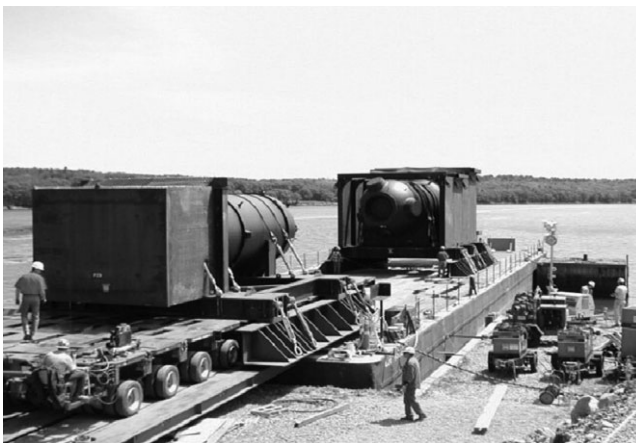
24.5 Maine Yankee steam generators on barge.
