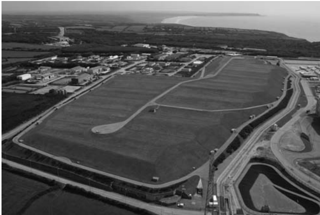
14.14 Aerial view of the Centre de la Manche disposal facility in France. The disposal facility has been closed and covered with clay and grass (© Zorilla Production).
