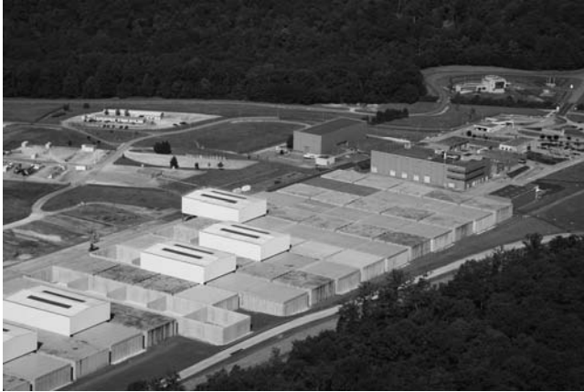
14.13 Aerial view of the Centre de l'Aube disposal facility for low-level waste in France (© 4 vents).
