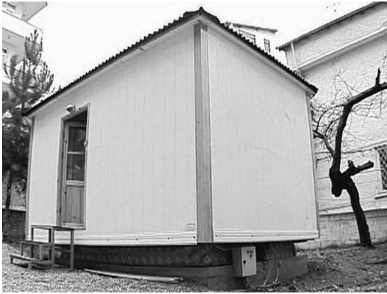
Figure 4.3 Earthquake simulator: outside view.
