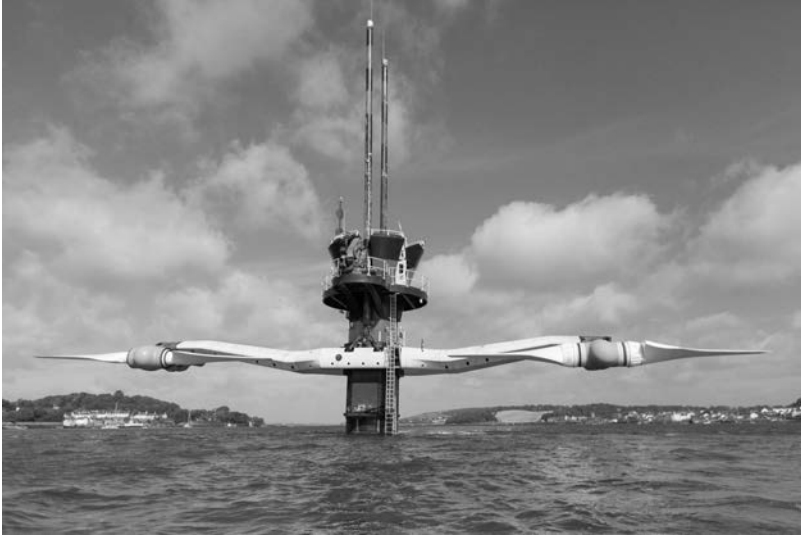
Figure 2.10 SeaGen device, turbines lifted above sea-level for inspection and maintenance (reproduced by permission of Marine Current Turbines Ltd)
