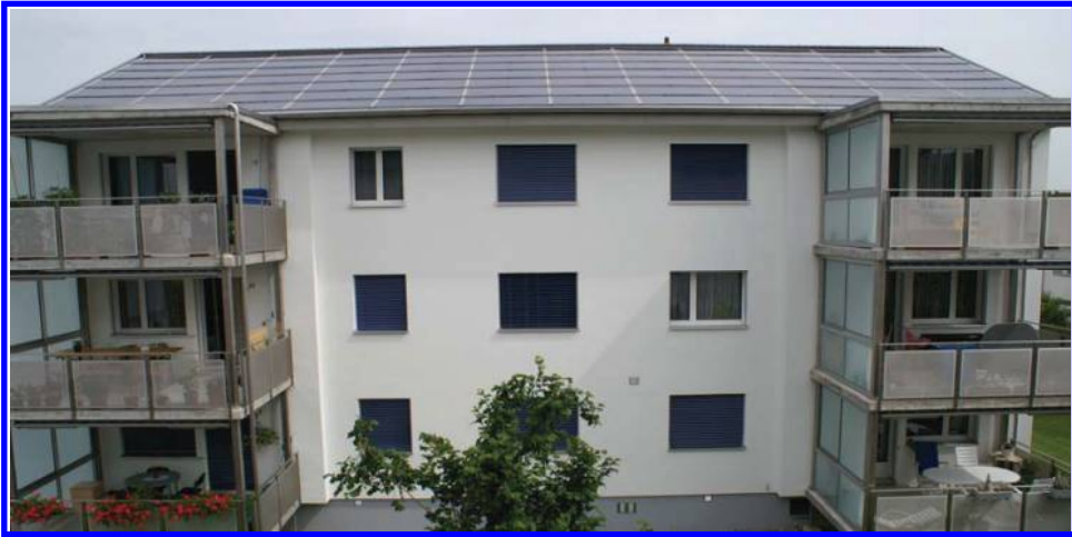
Figure 41. With investments of about 100 000 CHF per apartment unit, the six-family house in Staufen, Aargau, from 1967 reduced its total energy need from 122 000 kWh/a to 15 000 kWh/a or by 88%. Increase in efficiency amounts to 62 000 kWh/a, whereas the 15 000 solar-powered heat pump and the solar installation produce approximately 45 000 kWh/a. The increase in efficiency could have been even higher if the refurbishment was done according to the standard of MinergyP/passive buildings instead of just Minergy; see Swiss Solar Prize 2008, p. 24/25.
