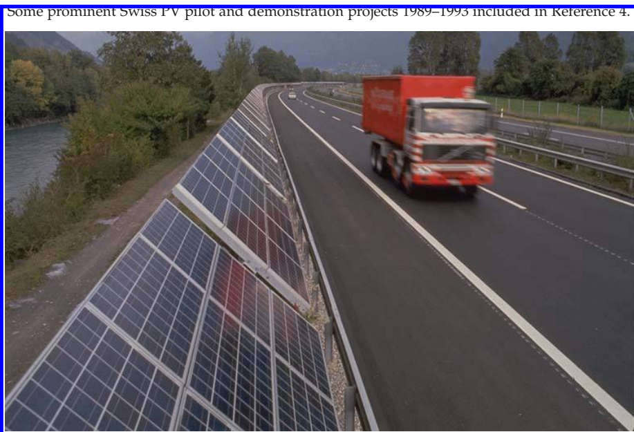
World's first PV-Soundbarrier — 100 kWp, Domat/Ems (near Chur, Switzerland), 1989.
