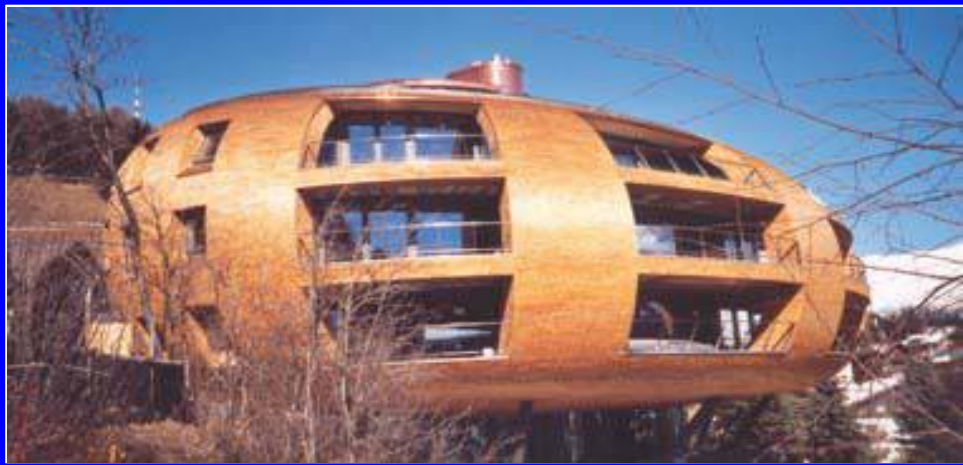
Figure 39 Chesa Futura in St. Moritz was built by Lord Norman Foster in 2002. Thanks to its envelope with 50 cm of insulation, the big energy losses are reduced by 70 to 95%.
