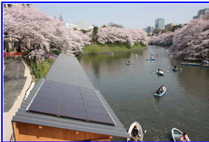
Figure 4. Thin-film silicon PV system, Chidorigafuchi, Tokyo.
