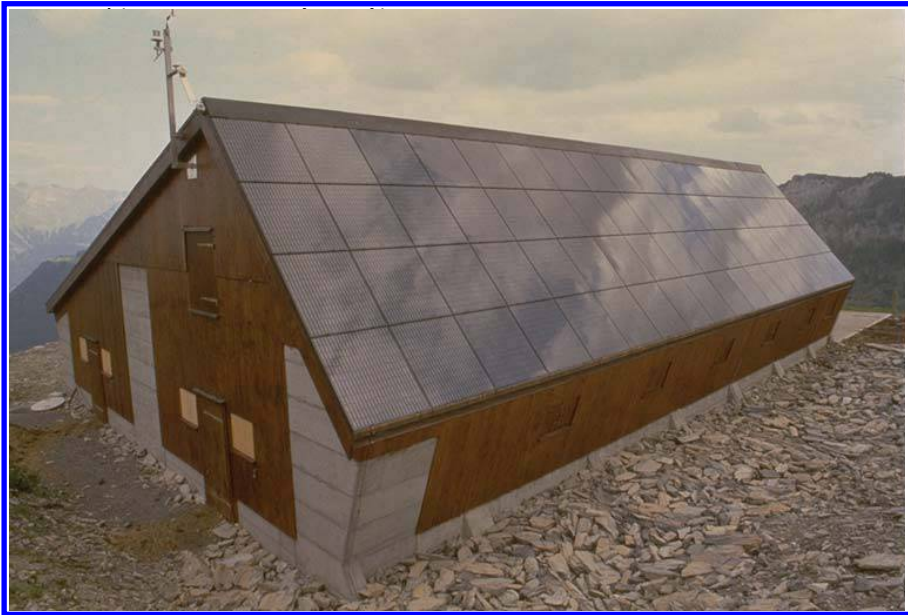
Alpine BIPV-Dairy — 13.3 kWp, Alp Findels Pfäfers, 1991.
