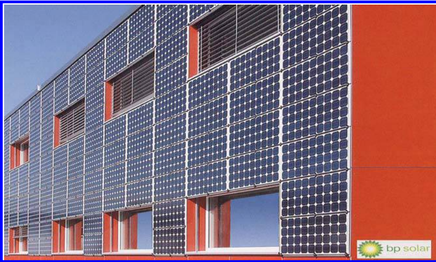
Figure 36. Wattwerk's PV installation has a capacity of 30 kWp. It produces 24 500 kWh/a, and only needs 13 800 kWh/a. The excess of solar electricity therefore is 10 500 kWh/a, enough to supply the company's solar-powered electric cars which are used by the employees to supervise the solar projects in the region. Wattwerk is owned by Heinrich Hollinger, a veteran and successful Tour de Sol participant. He was awarded the Swiss and European Solar Prize in 2004.
