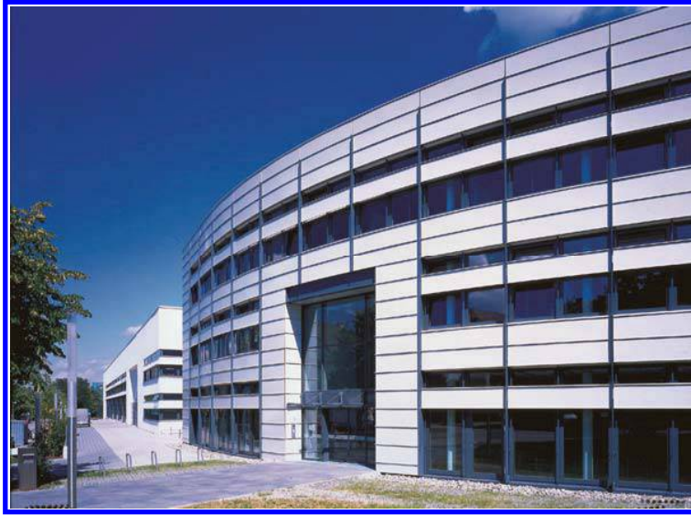
Figure 1.1. Front view of Fraunhofer ISE.
