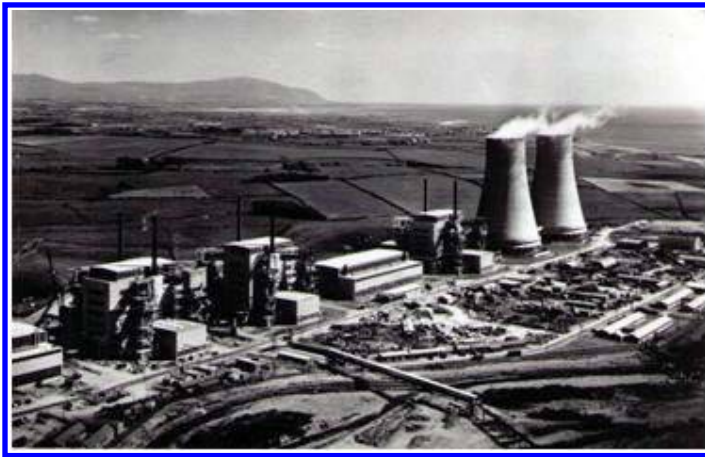
Figure 4. Windscale Nuclear Plant/UK.
