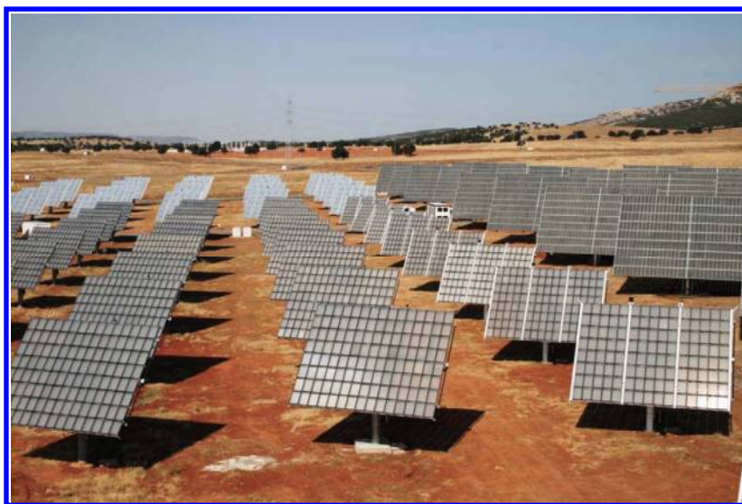
Figure 3. 800 kW MJC CPV panels installed at the central Puertollano site of ISFOC. Modules of three different companies are installed there.
