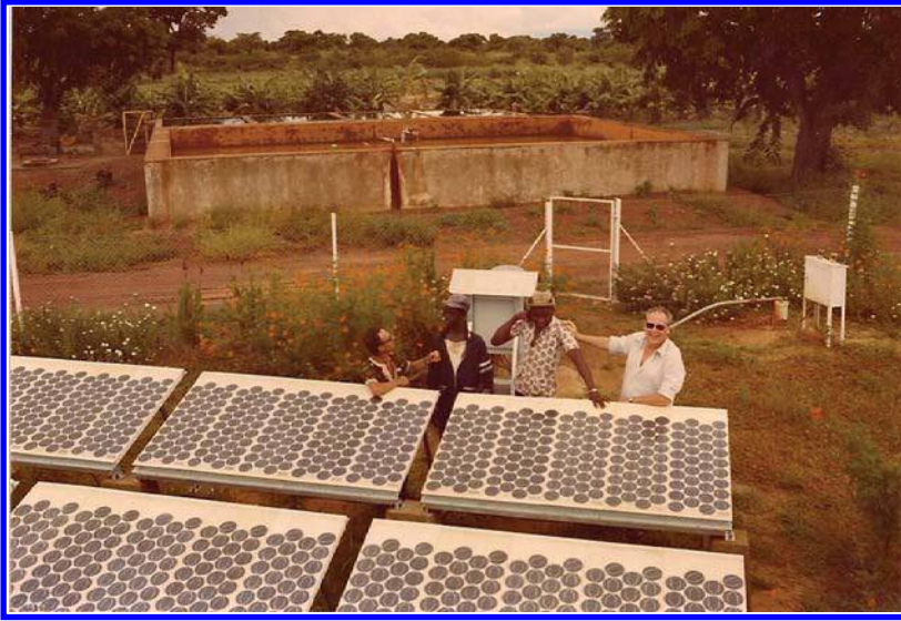
Figure 40. A French Catholic priest, Father Bernard Verspieren, who installed hundreds of PV pumps in West Africa; he arranged to make the boreholes and do the installations in one day.
