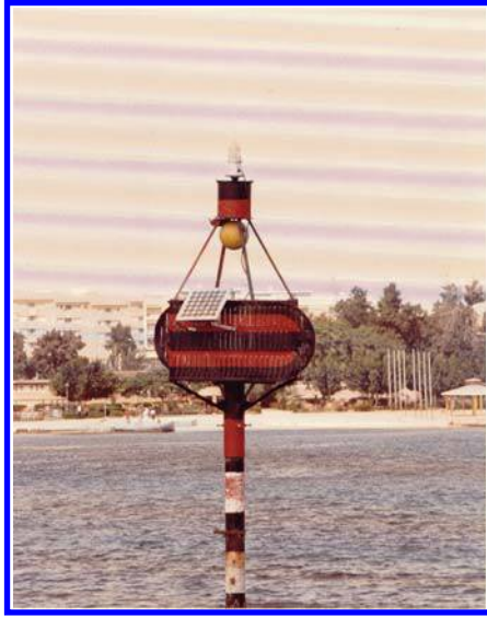
Figure 6. Suez Canal — solar powered navigational aid — 1982.
