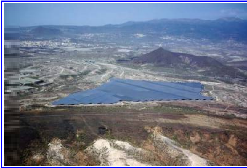
Figure 3. PV plant Solten 20 MW in Tenerife produced in 09 pro Watt 1.859 kWh a world record.
