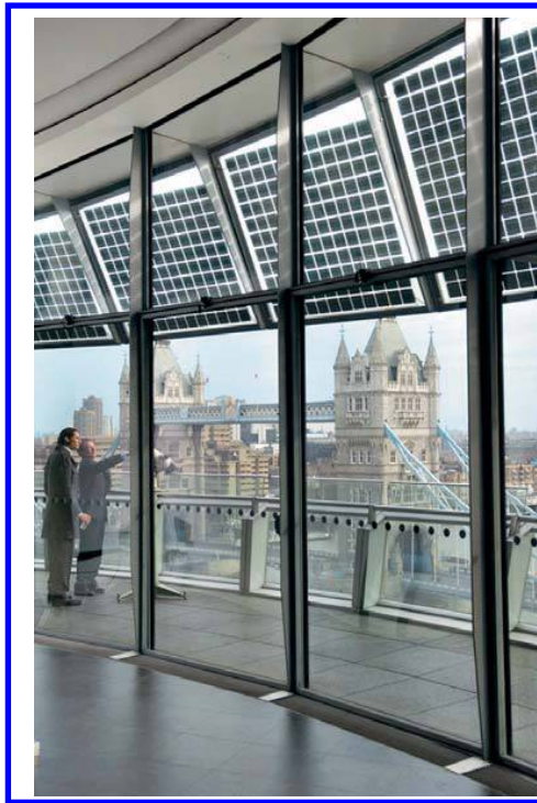
Figure 11. City Hall, London includes an array of photovoltaic panels on its roof, which were proposed from the outset but not finally fitted until 2007. These now complement the many other passive systems deployed to reduce energy consumption. For most of the year the building requires very little active heating – the major potential energy demand comes from cooling. To assist passive or low-energy cooling, the building is naturally ventilated for most of the year, with openable windows in the office spaces; heat generated by people, computers and lights is recycled; and cold ground water is pumped up to supply chilled ceilings.
