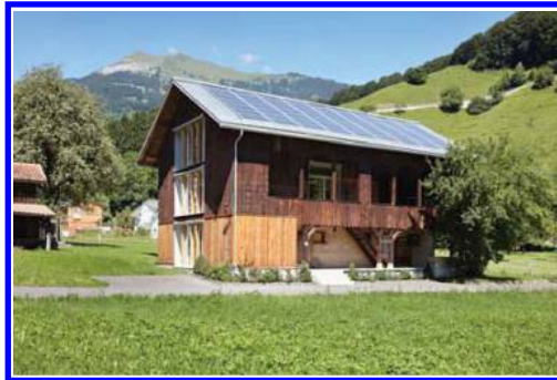
Figure 44. PEB refurbishment in Grüşch with a use of 15 000 kWh/a, and a production of 31 000 kWh/a. Self-supply: 207%. This PEB sells about 4 500 kWh/a (130%) to the grid.
