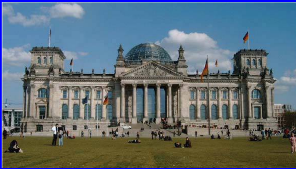
Figure 38. Energetic refurbishment of old and cultural buildings: The Bundestag from 1896 was refurbished by Lord Norman Foster in 1998 and is now using exclusively renewable energies. CO 2 emissions were reduced by 95% (PV installation of 37.5 kWp and biomass plant of 2.35 MW). If such a historic cultural building can energetically be refurbished by Lord Foster, this is also possible for other buildings. Further examples are the refurbishments by Karl Viriden in Basel where the energy needs were reduced up to 93% (see part 5).
