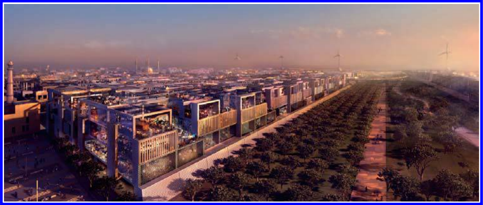
Figure 1. Masdar, Abu Dhabi. This pioneering development explores sustainable technologies and the planning principles of the traditional Arab walled city to create a desert community that will be carbon neutral and zero waste. Designed for a population of 90 000 people, it includes a new university and the headquarters for Abu Dhabi's Future Energy Company, together with special economic zones and an Innovation Centre. The city comprises two clearly defined quarters, the larger of which will be complete first. The surrounding land will accommodate wind and photovoltaic farms, enabling the community to be energy self-sufficient.
