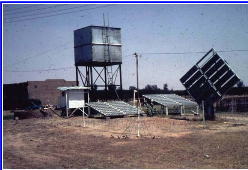
Figure 2. Solar pump test site, Energy Research Centre, Khartoum, Sudan, 1980.
