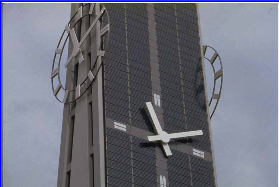
PV-Powered Church — 19 kWp, Steckborn (Canton of Turgau, TG), 1993.
