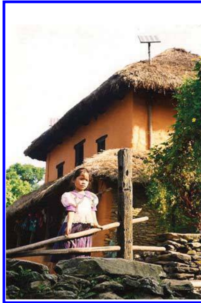
Figure 45. PV in a non-electrified village in Nepal.
