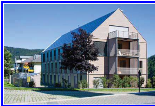
Figure 43. This PlusEnergy Building for 7 families in Bennau/Schwyz uses 62 000 kWh/a, and produces 70 000 kWh/a. This corresponds to a self-supply of 110%.
