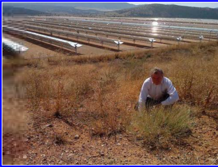
Figure 27. W. Palz at a 50-MW solar thermal power plant with “mirror trough” concentrators at Puertollano, Spain, October 2009.
