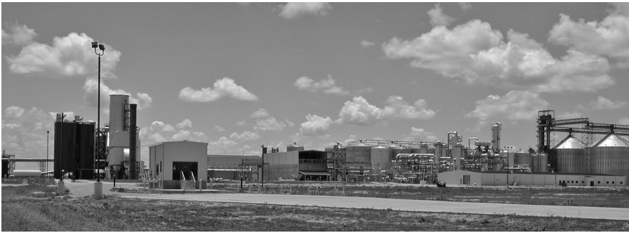
FIGURE 10.14 Ethanol plant near Herford, Texas.
