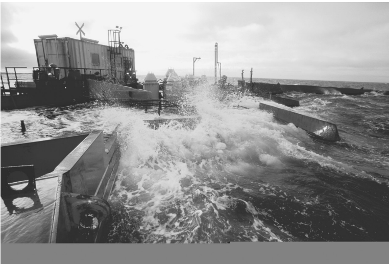
FIGURE 12.22 Prototype floating reservoir system, Nissum Bredning, Denmark. (Courtesy of Wave Dragon, http://www.wavedragon.net .)
