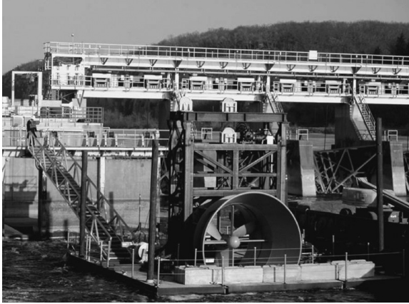
FIGURE 12.12 In-river system, 250 kW, on Mississippi River, Hastings, Minnesota. (Courtesy of Hydro Green.)
