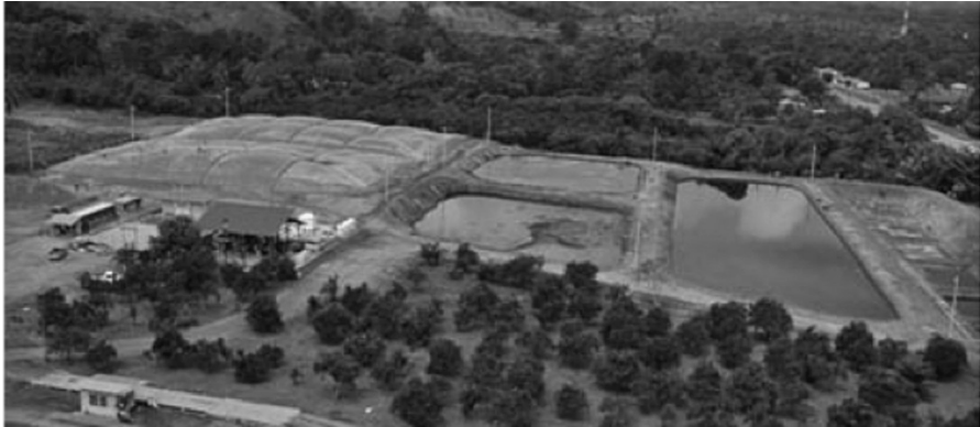
FIGURE 10.9 Palm oil plant near San Pedro Sula, Honduras. Biogas lagoons have plastic covering (top left).
