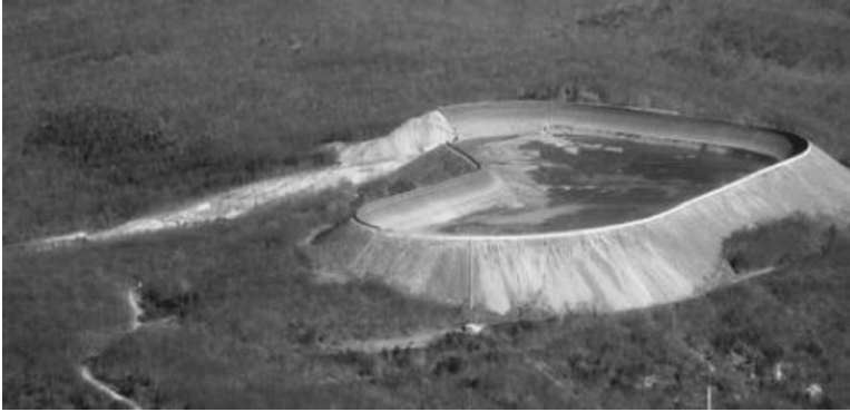
FIGURE 13.8 Upper reservoir for Taum Sauk pumped hydro plant, Missouri. Notice scouring of the creek due to wall failure. (Source: U.S. Geological Survey photo 037.)
