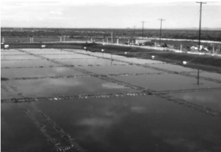
FIGURE 7.19 El Paso solar pond; notice wave suppression devices.
