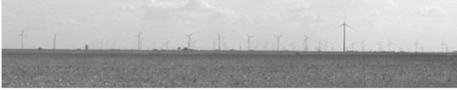
FIGURE 14.1 Visual aspect of wind turbines near Hitchland, Texas, looking south. Foreground: 3.2 km to one turbine, Vestas V 90, 3 MW, diameter = 90 m, 80-m tower; middle left, 4.4 km to row of eight Suzlon wind turbines, 1.25 MW, diameter = 64 m, 72-m tower; background, John Deere 4 wind farm, 9.5 km to first row, 14.5 km to back row, 38 Suzlon wind turbines, 2.1 MW, diameter = 88 m, 80-m tower.
