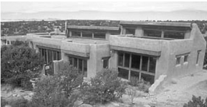
FIGURE 8.1 Passive solar home with direct gain; Trombe walls and large thermal mass provide most heating needs of an adobe home in Santa Fe, New Mexico. (From EERE, http://www.eere.energy.gov .)
