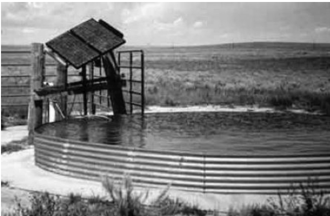
FIGURE 6.22 PV with passive tracker for pumping water for livestock. (From National Center for Photovoltaics, National Renewable Energy Laboratory (NREL), http://www.nrel.gov/ncpv .)
