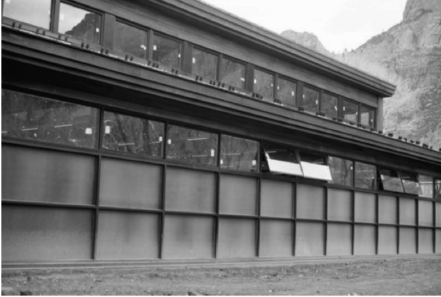
FIGURE 5.9 Visitor center has windows and clerestory for direct gain and daylighting and Trombe wall for indirect gain. The Trombe wall is the lower two rows of glass. That glazing is a single-covering, high-transmittance, patterned glass. Notice that the windows can open for ventilation. (National Renewable Energy Laboratory (NREL), http://www.nrel.gov/learning/re_solar_hot_water.html .)
