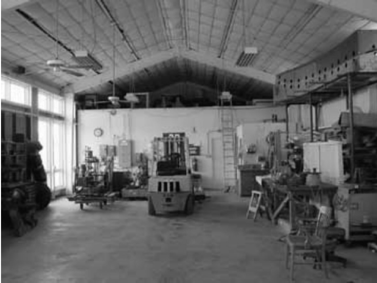
FIGURE 8.9 Interior of workroom showing that electrical lights are not needed due to daylighting.
