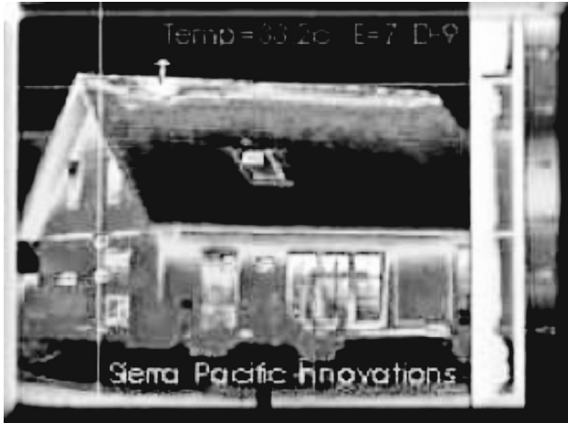
FIGURE 4.5 Infrared image for heat loss from a house. (Image, Sierra Pacific Innovations.)
