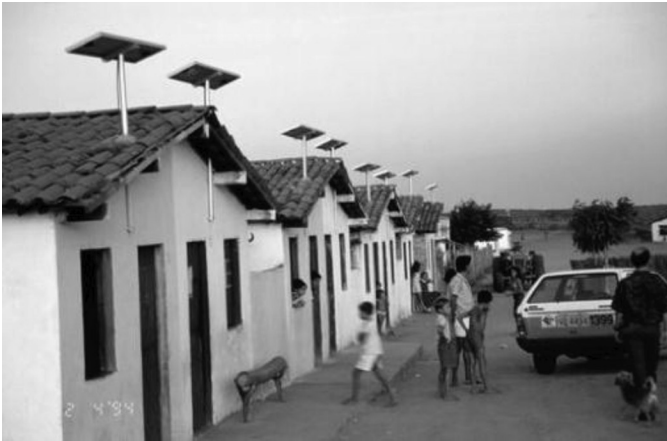
FIGURE 6.19 PV systems (50 W) for two fluorescent lights, village of Cacimbas in the state of Ceara, Brazil. Notice the tilt angle of the collectors. (From National Center for Photovoltaics, National Renewable Energy Laboratory (NREL), http://www.nrel.gov/ncpv .)
