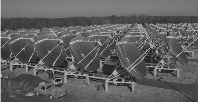
FIGURE 7.15 Solar Total Energy System, 144 dishes, 7 m diameter, at textile plant near Shenandoah, Georgia. The dishes provided thermal energy for process heat and air conditioning at a nearby textile mill. (From National Center for Photovoltaics, NREL, http://www.nrel.gov/ncpv .)
