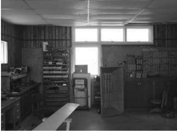
FIGURE 8.6 Concrete block wall filled with vermiculite, 6 ft high, on north wall. High windows on north and low windows on south open for nighttime flushing during summer.
