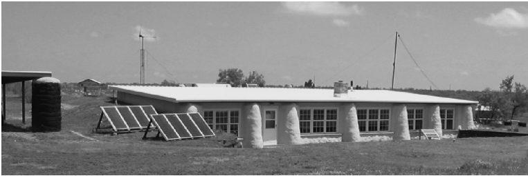
FIGURE 8.14 Off-grid home near Amarillo, Texas. South windows for passive, direct gain; PV; wind turbine; and tank for rainwater collection. (Courtesy of David Stebbins.)
