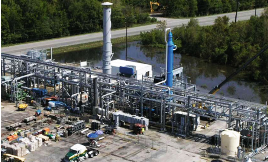
Fig. 10.5 Intermediate-scale test unit capable of producing up to 100 TPD of oxygen (Reproduced from Anderson et al. [8] with permission of Elsevier)
