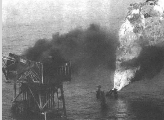
The Piper Alpha Platform After the Accident
