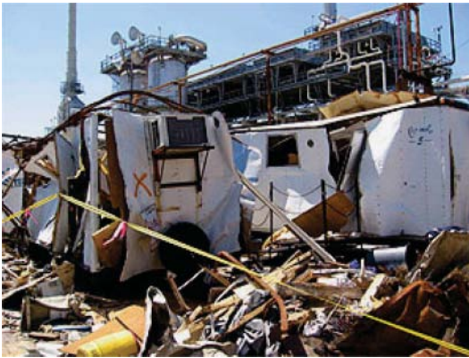
Damaged contractor's trailer
