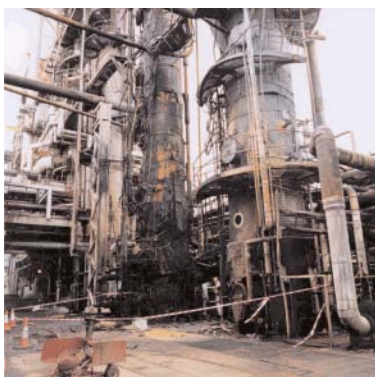
Figure 1a Refinery damage after a fire.
