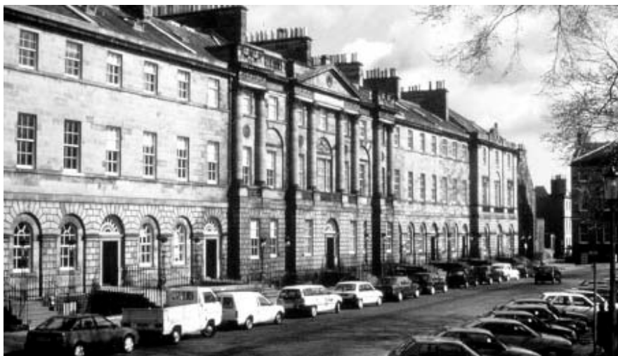
Figure 3.11. North wing of Robert Adam’s Charlotte Square, 1792: nine terraced houses lining the north side disguised as a single palace-front design to which developers had to adhere. (Source: Author’s collection)
