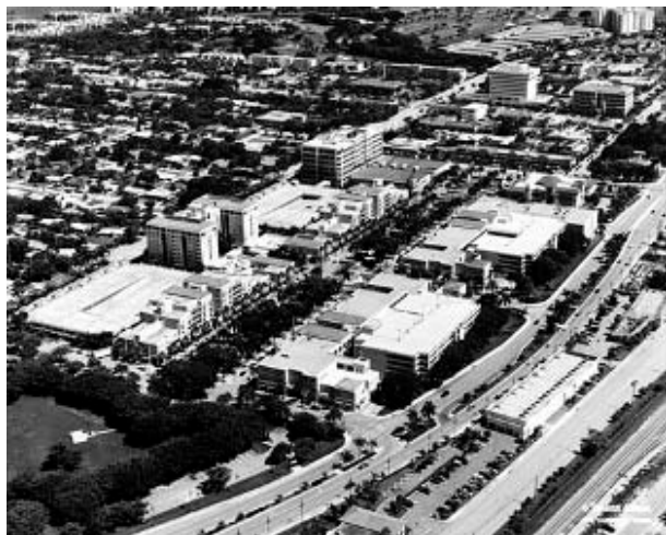
Figure 11.9. Aerial view of Mizner Park in Boca Raton, Florida, where a failed shopping mall has been replaced with a walkable mixed-use district with retail, offices, and apartments, supported by parking garages.
