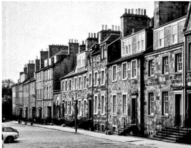
Figure 3.6. West side of George Square, Edinburgh, begun in 1766. Note the heterogeneous nature of the houses, altogether more relaxed in their scale and materials than subsequent developments in the New Town. (Source: Author's collection)
