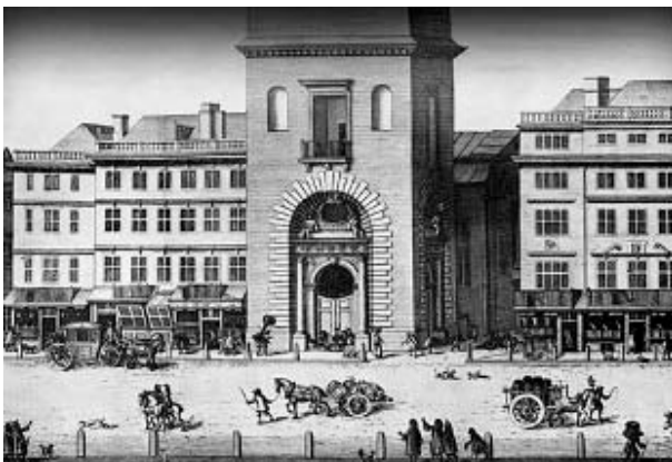
Figure 2.2. Elevation of Cheapside, showing the front of St Mary-le-Bow. The houses would have been of type authorized for ‘high and principle’ streets. (Source: Reddaway, 1940)
