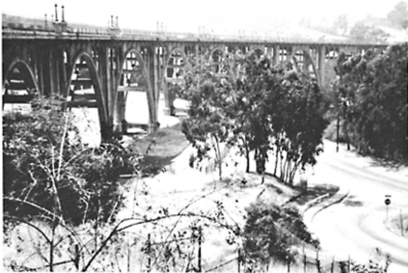
Fig. 1. Colorado Street Bridge
