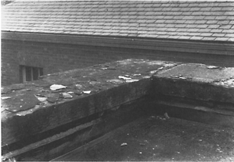
Plate 1. Frost damage attributed to the formation of ice lenses.
