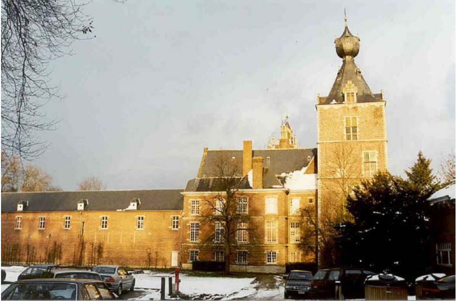
Figure 1. Exterior view of the castle (photo: Paul Van Aerschot)
