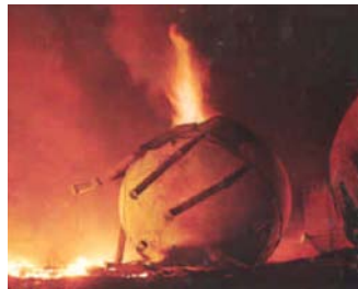
Figure 4 Fire at refinery storage area. Eighteen firefighters were killed during this incident, when the first sphere BLEVEd.
