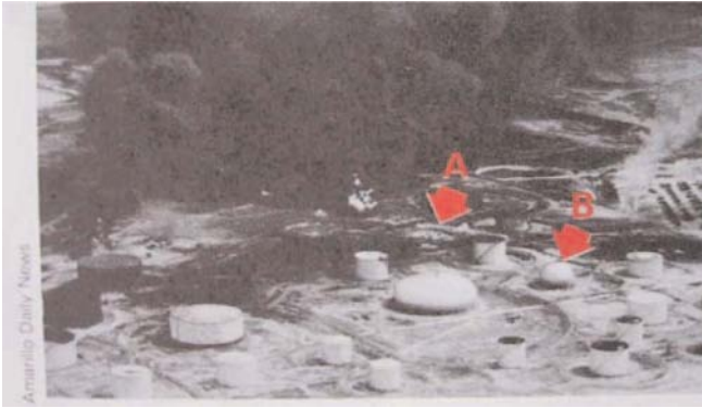
Figure 60 The spheroid at 'A' ruptured and caused the tank fire shown. Flame impingement from a relief valve weakened the spheroid shell. The spheroid at 'B' is the companion to the one at 'A'.
