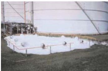
Figure 76a Example of foam blanket over an LNG spill. This foam was applied by fixed foam pourers but, for condensate spills, portable foam application will achieve the same results if the response crews are well trained.
