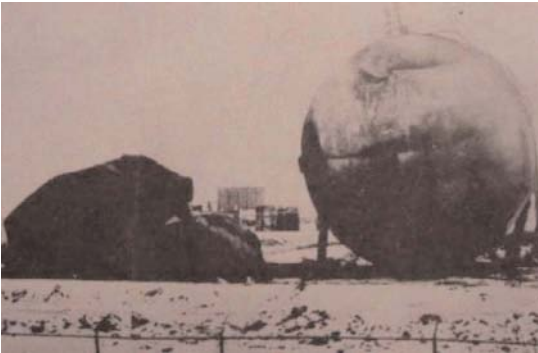
Figure 36 The sphere at the left (which contained butane) was pumped over. The spilled butane ignited, and the resulting fire ruptured the sphere shell.
