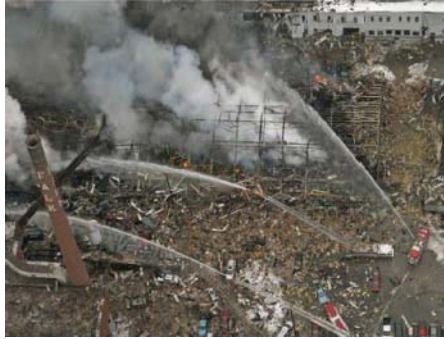
Figure 5c This factory was destroyed and three employees killed in what was reported to be a propane explosion.
