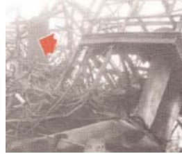
Figure 16 Propane enriched with oxygen detonated. Ignition was probably caused by iron sulphide. The three propane storage drums (Figure 15) fragmented. Arrow (Figure 16) indicates remains of one of the propane storage drums. Other equipment was damaged by fire from the released hydrocarbons.
