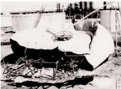
Figure 31a Spheroid rupture was caused by low-grade explosion. Vacuum damage was due to an outrush of water following explosion.
