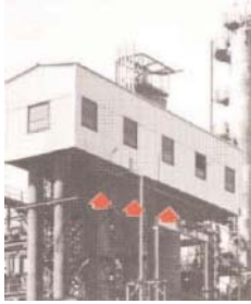
Figure 15 Arrows indicate location of three propane storage drums near an alkylation unit.
