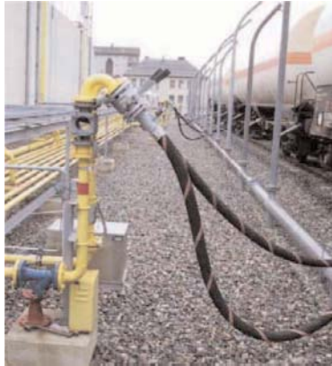
Figure 47 Example of rail car unloading station using flexible hoses.
