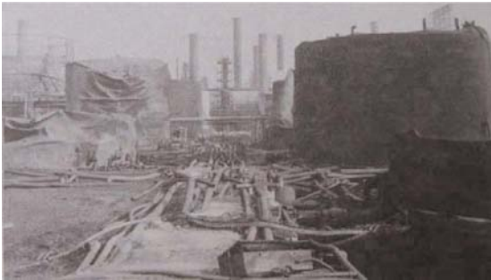
Figure 50 Screwed pipe failure due to fire.
