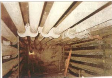
New roof hangers.
