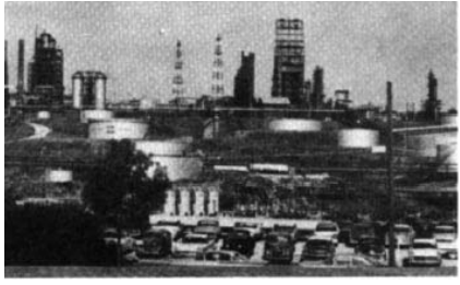
Figure 35 Location of operating units above adjacent tankage (right illustration) is preferred to location of units below tankage (left illustration).
