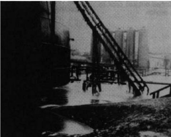
Figure 33 Hot asphalt and a leaking steam coil result in a foamover.
