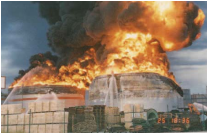
d. Two tanks fully involved.
