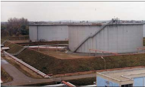
Figure 36 Grade against oil-water flow. For example, if unit dock is at normal ground elevation, pipe alley should be below unit grade and combination fire wall and road above unit grade.
