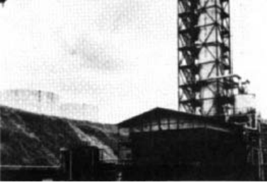
Figure 35 Location of operating units above adjacent tankage (right illustration) is preferred to location of units below tankage (left illustration).
