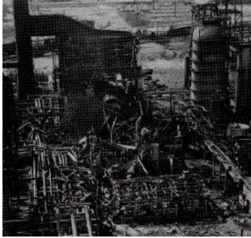
Figure 24 A fluid hydroformer being brought onstream was destroyed by a series of internal detonations. Air accidentally entered the unit and contaminated the circulating inert gas and naphtha vapours. This air backed in through one or both valves in the catalyst circulating lines which had failed to close even though exterior inspection indicated them to be closed. The most probable source of ignition was the heated walls of the recycle gas furnace tubes. The explosion was violent enough to throw a 65-ton piece of steel 1,200 feet (365 m).
