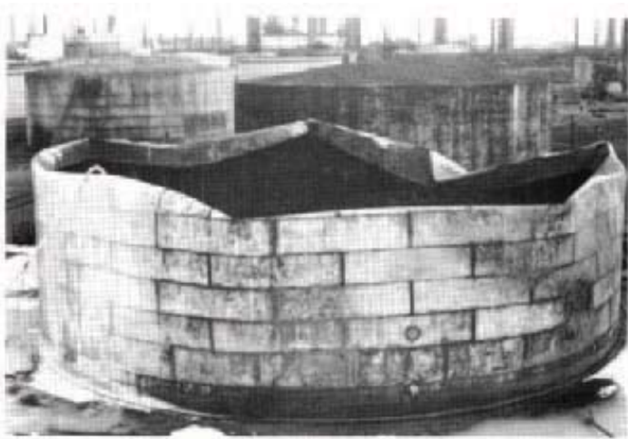
Figure 8a Iron sulphide ignited an explosive atmosphere in this reduced-crude storage tank. Air entered when stock was pumped down. A partially submerged steam suction heater is believed to have vaporized some of the lighter fractions and also to have dried the iron-sulphide deposits.
