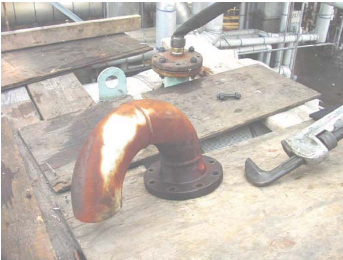
Figure 57a Vent and water hose installed.
