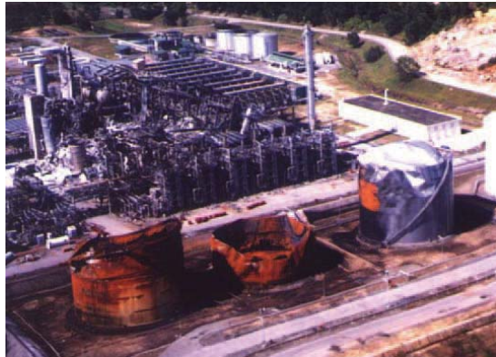
Figure 49 Explosion on a cryogenic distillation column.
