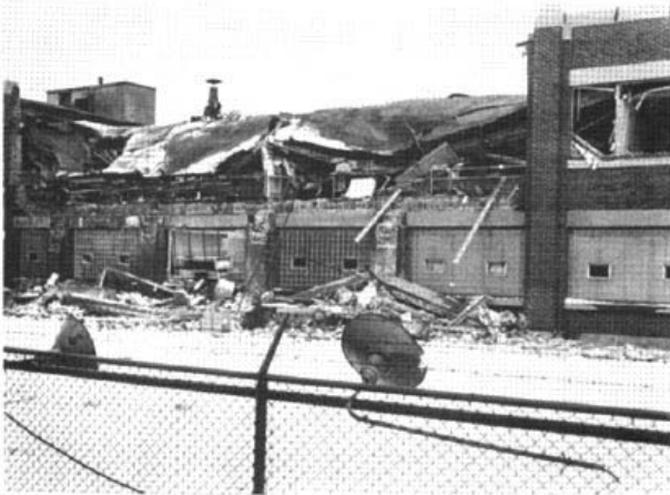
Figure 38 Damage to this laboratory building resulted from a flash fire and explosion following the rupturing of a sampling container.
