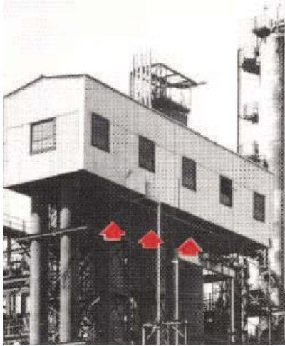
Figure 3 Arrows indicate location of three propane storage drums near an alkylation unit.
