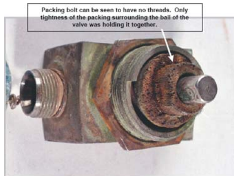
Condition of the sample point valve
