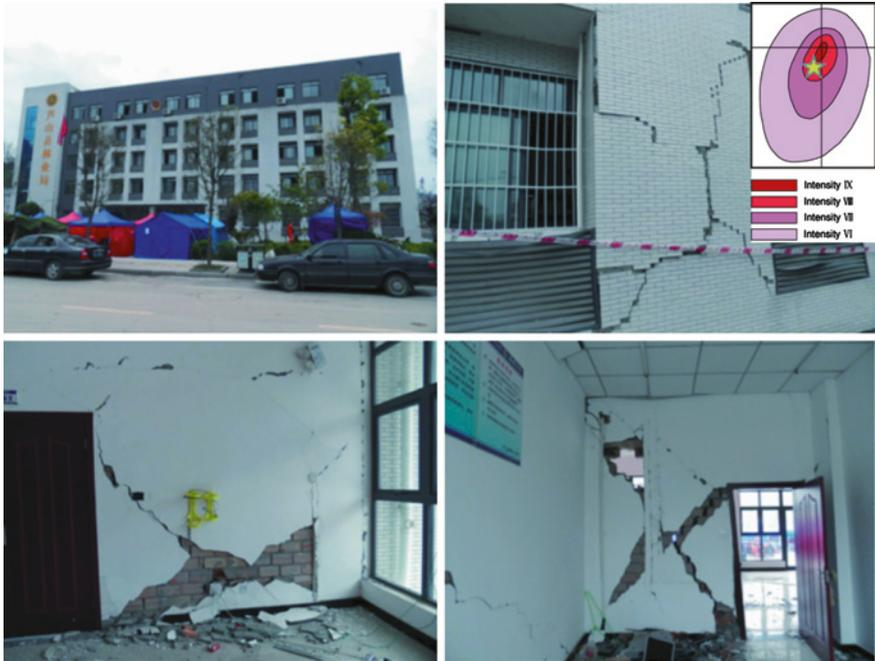
Fig. 8.6 Damage of the infilled wall in an office of the Lushan Forestry Bureau, picture from Gong et al. (2013)
