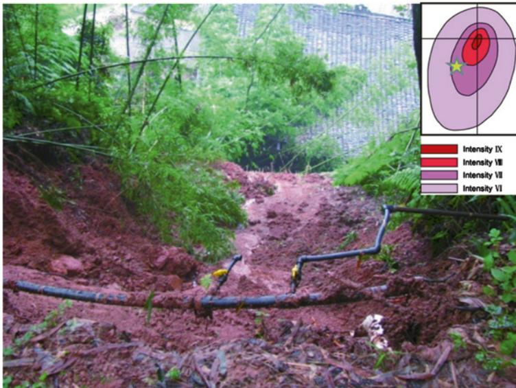
**Fig. 8.16** Damage of pipe of Ren Yi Water Company at Tianquan County
