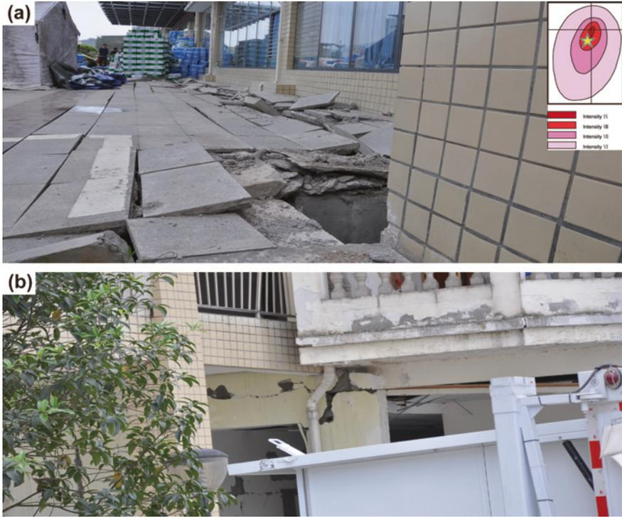
**Fig. 8.10** Damage of the Lushan Hospital. **a** Damage of the connection between the main building and the attachment. **b** Damage of the connection between the main building and the attached building
