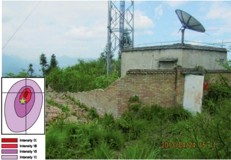
**Fig. 8.14** Collapse and electricity power cut in a base station of China Unicom Sichuan Branch, Longmen Town, Lushan
