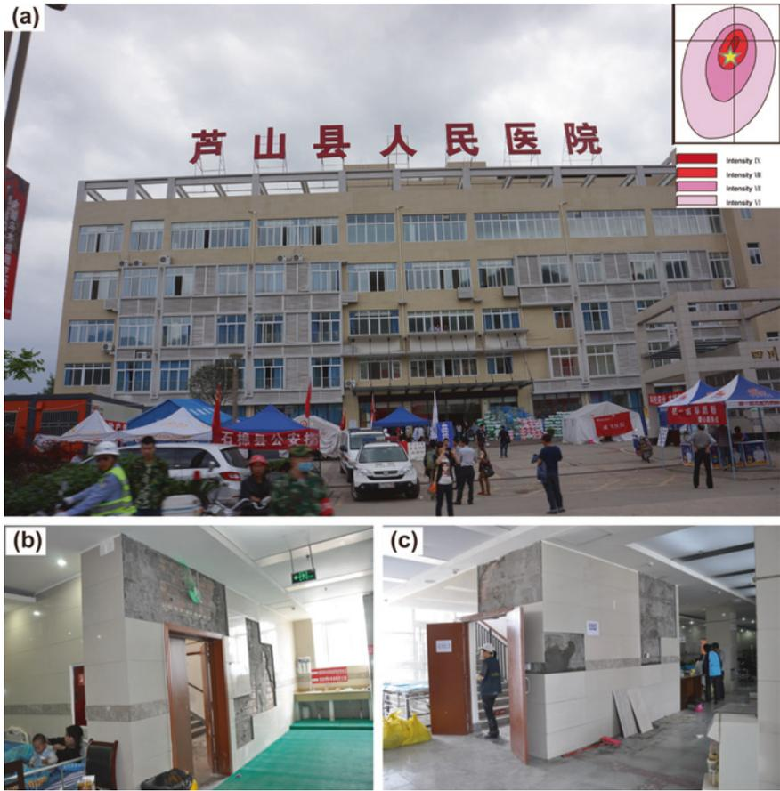
**Fig. 8.8** Damage of a base-isolated structure: the Lushan Hospital. Investigation indicated that the main structure was basically undamaged, with slight detachments of the in-door decorations. The building came into use just 5 days after the Lushan earthquake
