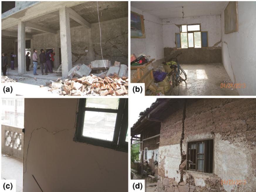
**Fig. 8.2** Damages of typical buildings located in different intensity zones. **a** Damage of a frame construction in Baosheng Town, Lushan (Intensity IX). **b** Cracks of a brick masonry building in Feixianguan Town, Lushan (Intensity VIII). **c** Cracks of a brick masonry building in Lieshi Town, Yingjing (Intensity VII). **d** Expanded cracks of a loam wall building with existing cracks in Sanjiao Town, Hanyuan (Intensity VI)
