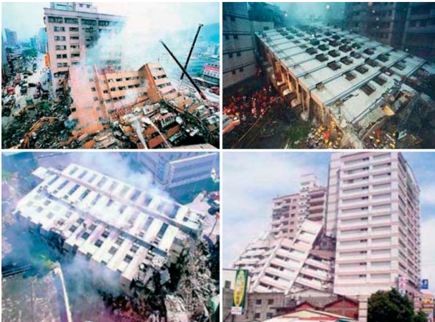
Fig. 33.1. Buildings damaged in the great Chi Chi earthquake on September 21, 1999 in Taiwan. More than two thousand lives were lost
