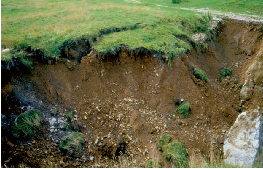
Fig. 5.36 Slumped cover block in the side of doline I in the Pádis-2 area
