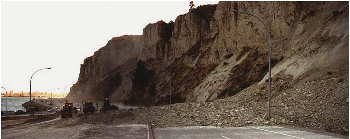
Fig. 4.5. Dry silt flow near Peachland, British Columbia (photo courtesy of Mr. J. Valentinuzzi, British Columbia Ministry of Transportation and Highways)
