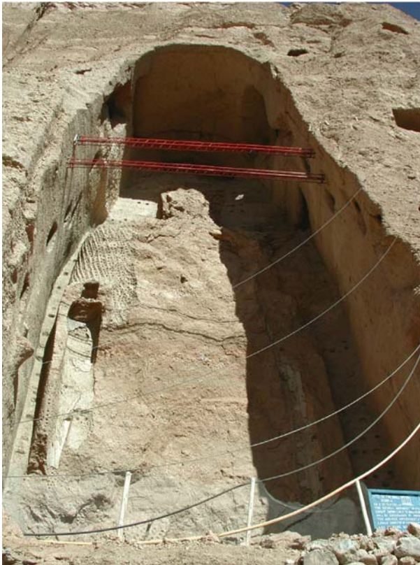
Fig. 25.33. The temporary beam ( left ) and steel rope ( right ) for the temporary support of upper Eastern part of Eastern Giant Buddha
