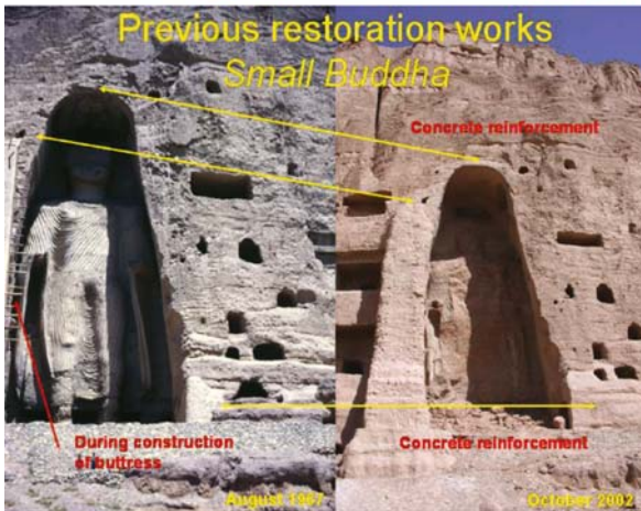
Fig. 25.23. Reshaping and consolidation with cement in both Western and Eastern Giant Buddha
