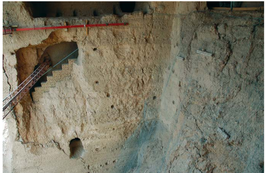
Fig. 25.43. The metallic net protecting from the detachment and fall of small stones from the shear band of destroyed statue
