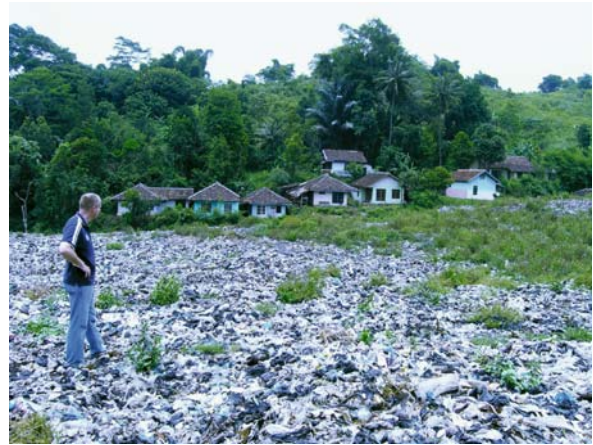
Fig. 10.7. Houses which survived the failure of landfill
