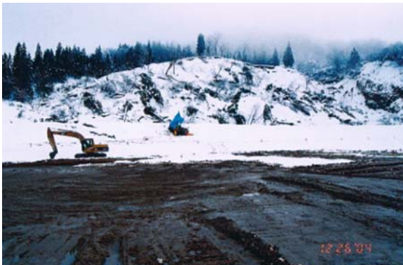
Fig. 21.14. Excavation of the displaced soil mass
