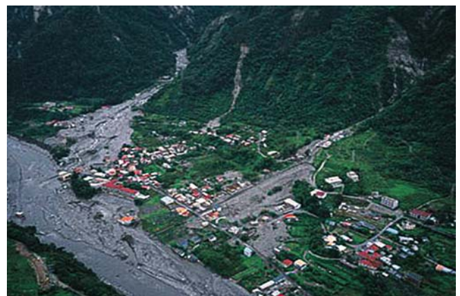
Fig. 26.1. Debris flow disaster of Song-Her village in central Taiwan. The village is partially buried by debris flows and original small stream outbursts into debris flow river of more than 30 m wide. This scenario is typical in Taiwan (Photo provided by Water and Soil Conservation Bureau, Taiwan)
