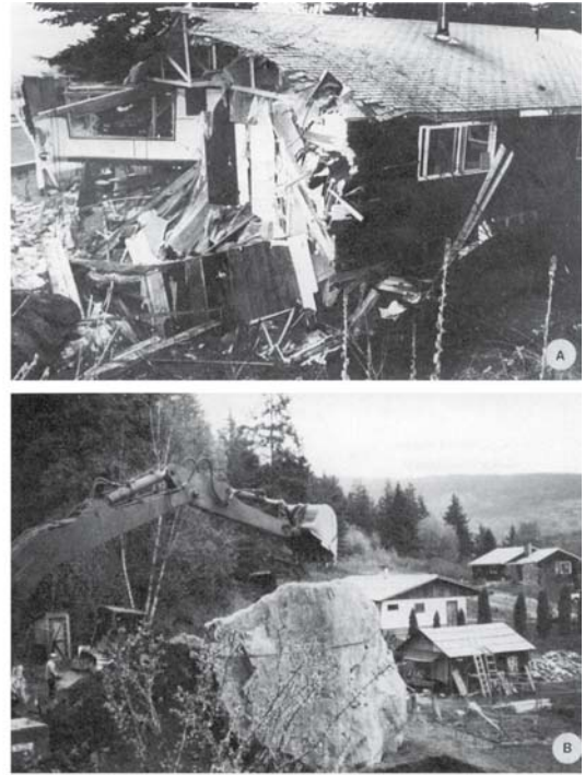
Fig. 4.4. Dynamic analysis of a 100 tonne rock fall. a Damage, b boulder (Hungr and Evans 1985)
