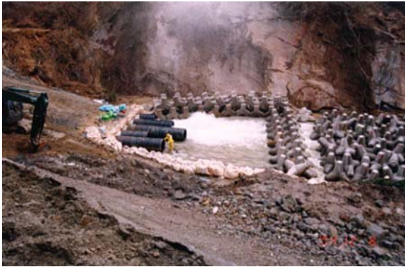
Fig. 21.12. Alternative diversion pipe-lines
