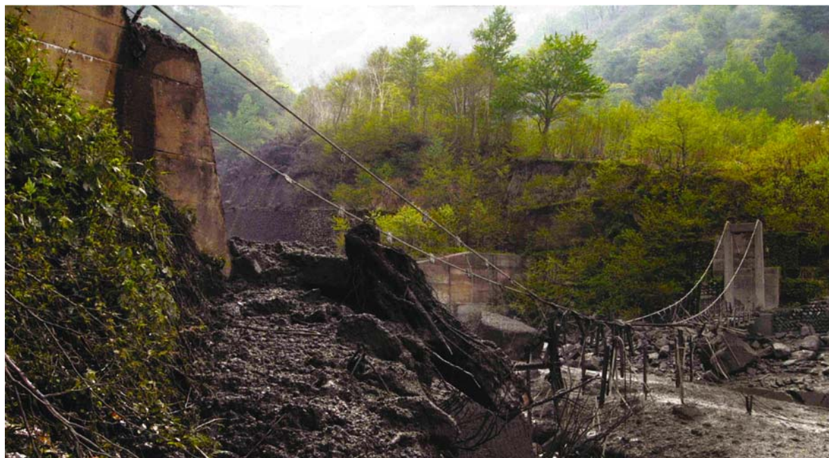
Fig. 11.10. The suspension bridge that was completely destroyed by the May 2004 debris flow in the Bettou-dani (photo courtesy of the Kanazawa Office of Rivers and National Highways, MLIT)
