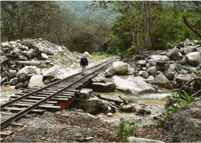
Fig. 24.5. The railroad after reparation – situation in September 2005 (photo by V. Vilímek)
