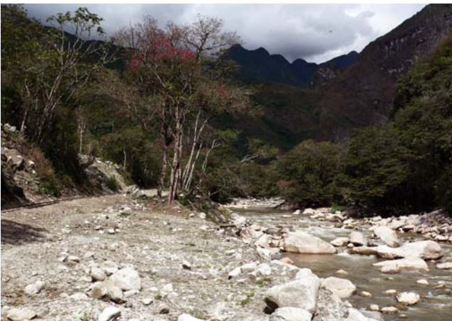
Fig. 24.6 The riverbed of Urubamba River. All the material from the debris flow was already removed from this area (photo by V. Vilímek)
