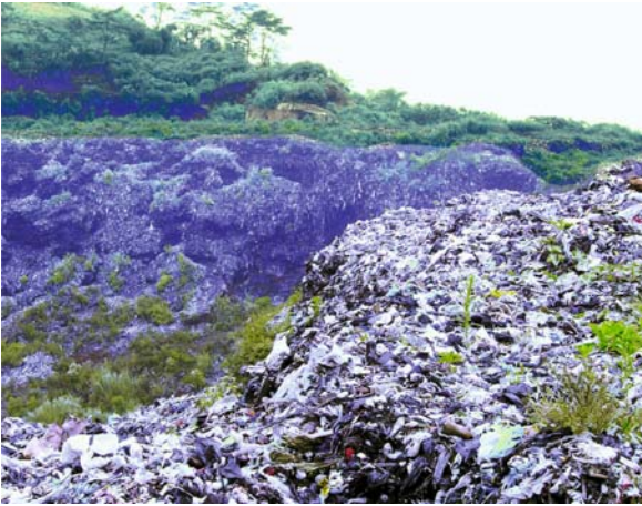
Fig. 10.3. Head scarp of landfill failure
