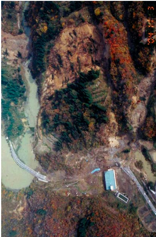
Fig. 21.8. Plane view of the Higashi-Takezawa Landslide
