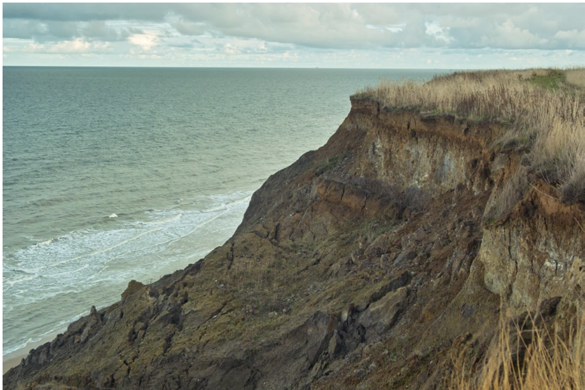
Fig. 4 Cliff collapse is common along sections of the North Norfolk coast
