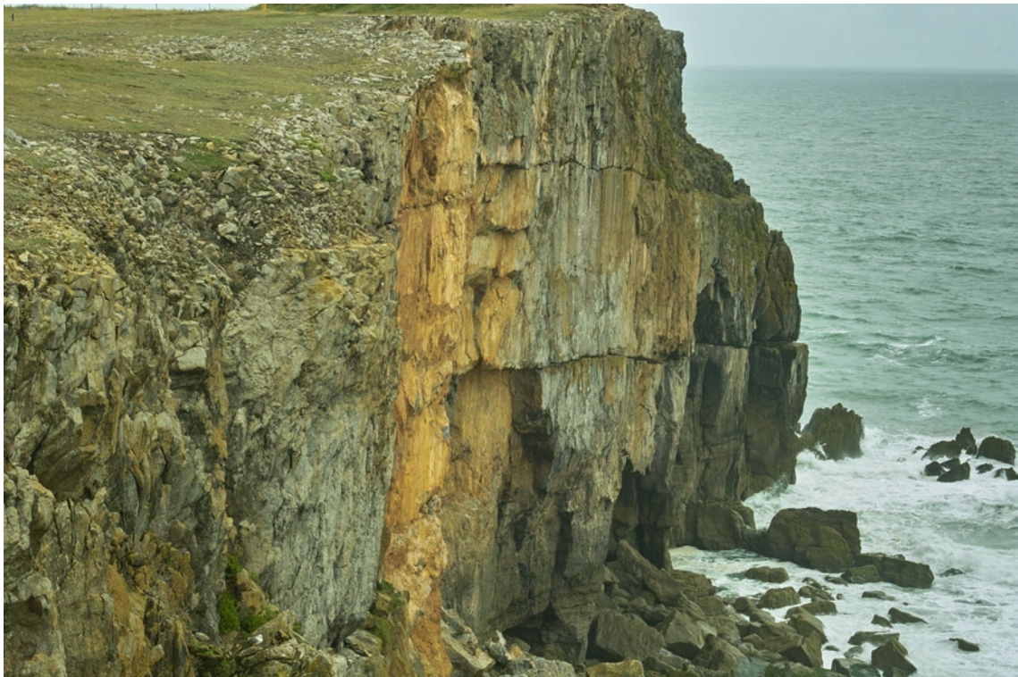
Fig. 5 An unstable cliff at St Govans in Pembrokeshire
