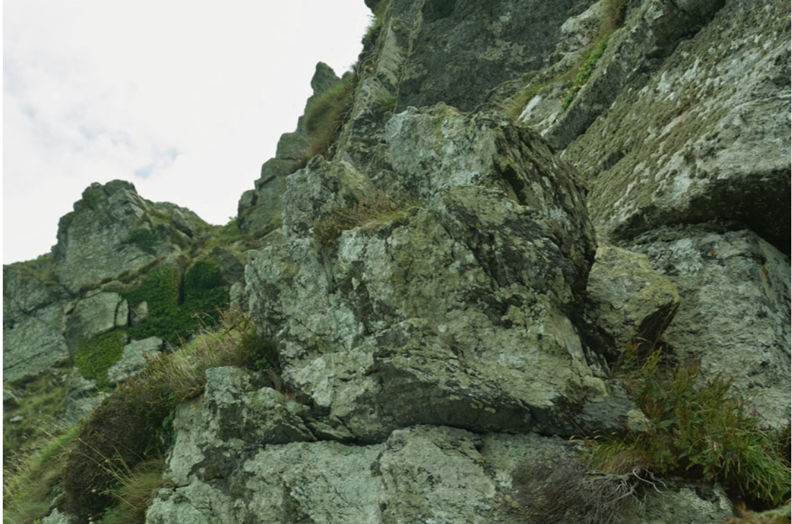
Fig. 5 The exposed rocks are sometimes of a loose and fragile composition
