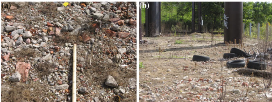
Fig. 10.7 Demolition site showing extensive accumulation of artifacts comprising “hardcore” (Detroit, Michigan USA). Scale marked in 10 cm intervals. Photos by J. Howard
