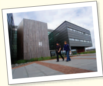
PHOTO GALLERY Here is where deCODE genetics does much of its work in Iceland. Icelandic Photo Agency/Alamy Limited
