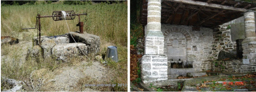
Fig. 13.9 Public water fountains and wells in Greece
