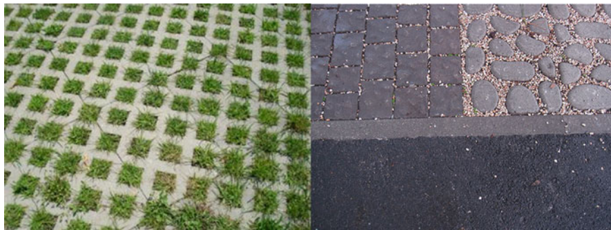
Fig. 13.17 BMPs: Grid system filled with grass (Source: http://www.plantmoreplants.com/press-photo/category/ ) & permeable pavements
