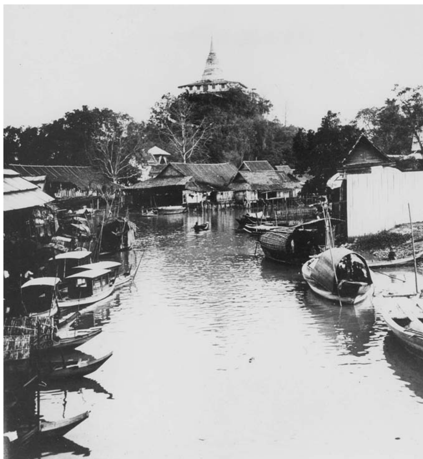
Plate 1.1 The aquatic city: houses along a main canal surrounding the walls of Krung Thep (c. 1890s). (Photo: Courtesy National Archives of Thailand)
