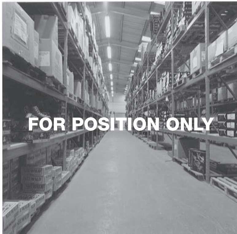
Figure 16.4 Adjustable pallet racking (courtesy of Redirack Limited)
