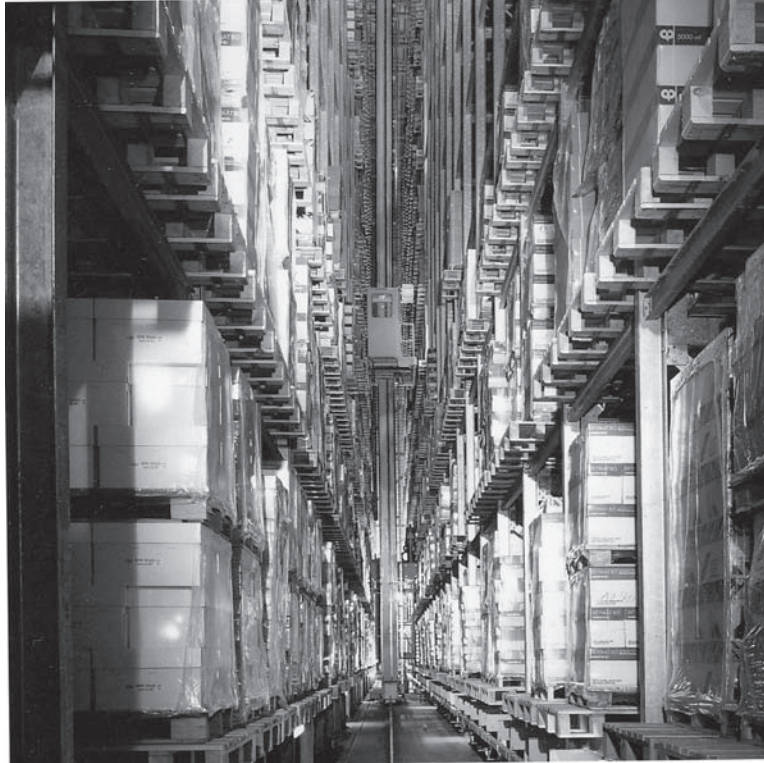
Figure 19.2 Stacker crane (courtesy of Morris Material Handling)
