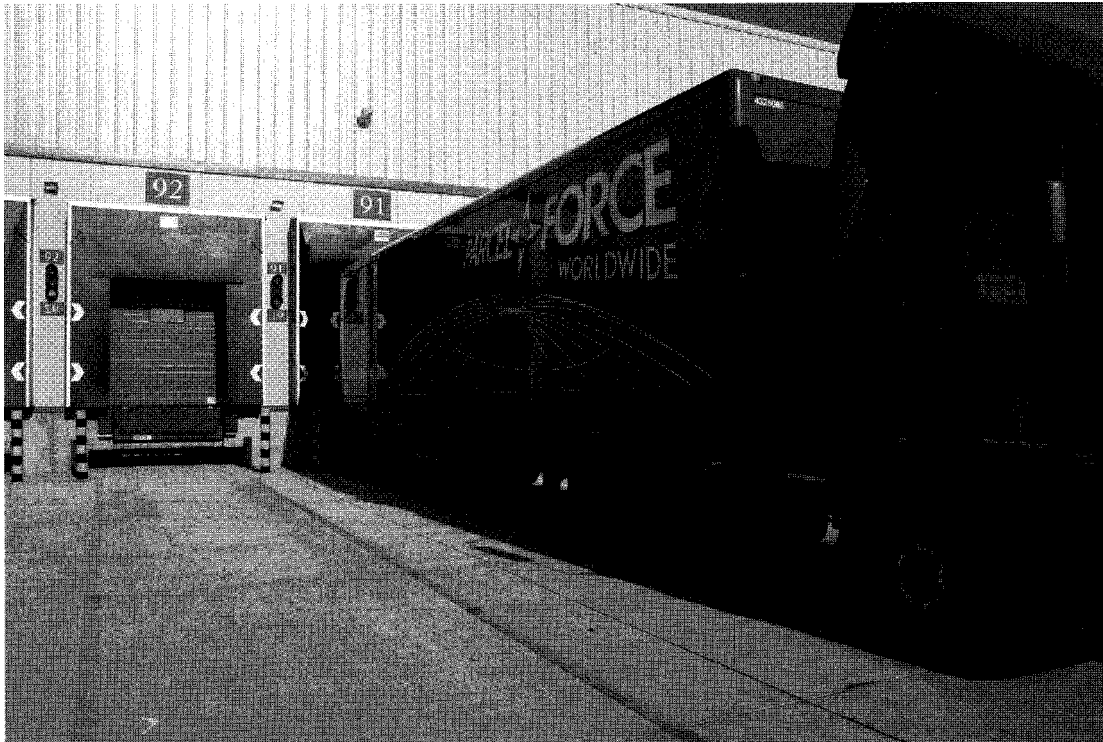
Figure 18.1 Raised docks fitted with dock levellers (courtesy of Stertil)
