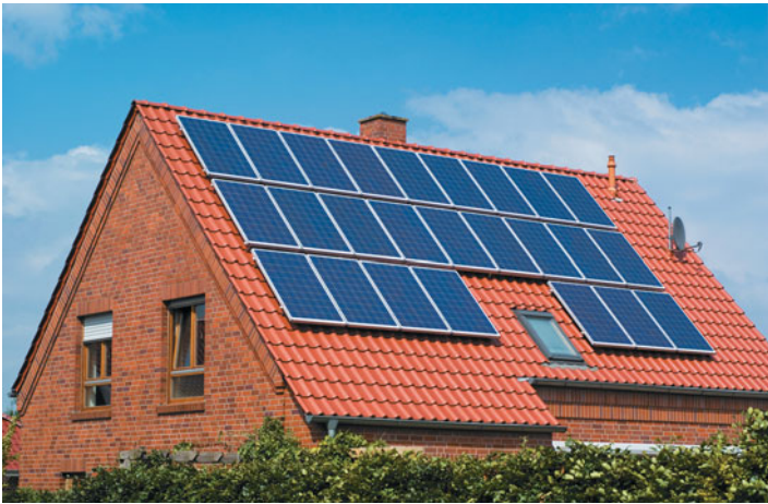
b) Photovoltaic solar panels. Photovoltaic panels can provide enough electricity to power a home.
