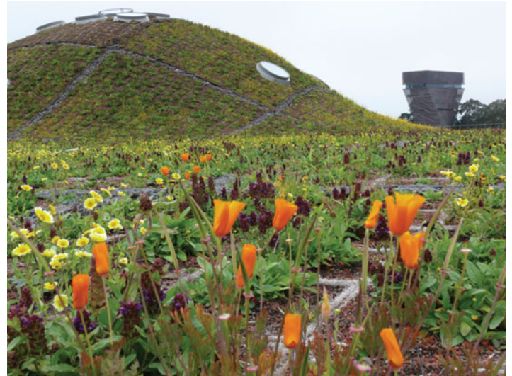
Figure 24.14 A green roof. The roof of the California Academy of Sciences building in San Francisco is covered with native plants and recycled materials.
