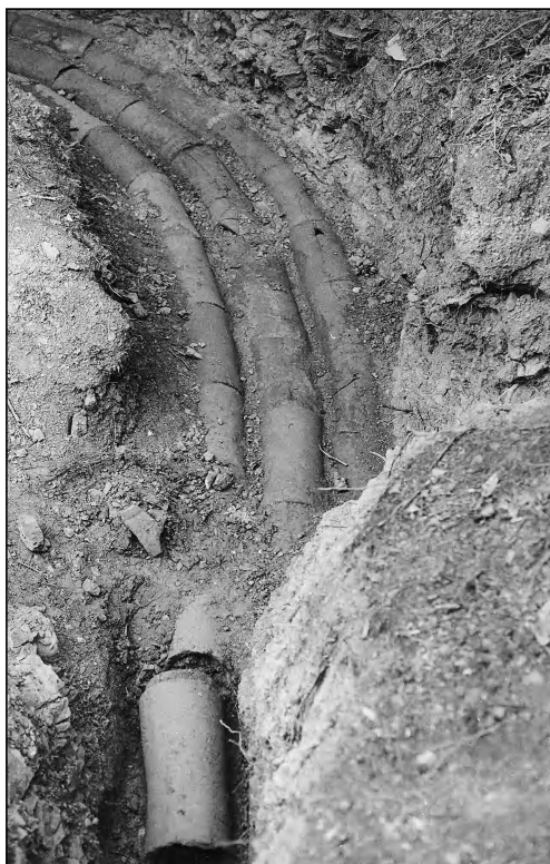
Figure 5.9 The three clay pipelines of the Mandradag aqueduct (photo of G. Garbrecht).
