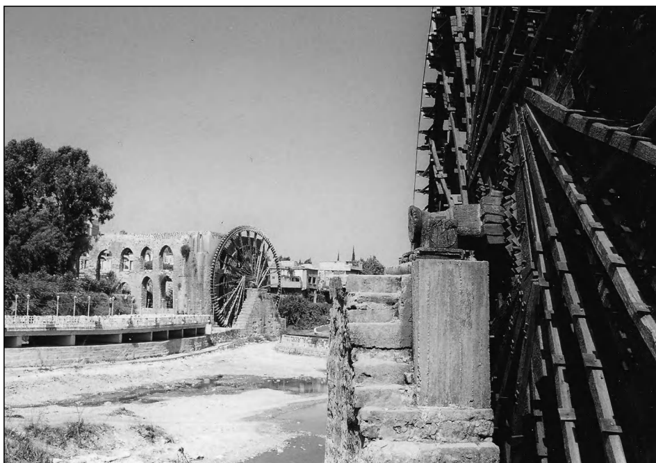
Figure 7.19 In the foreground, the axle of the noria al-Gisriyya at Hama; and in the background the noria of al-Mamuriyya, dating from 1453. Prior to its first reconstruction, this latter noria was the second largest in size (after the noria of al-Mohammadiyya). (Photo by the author).
