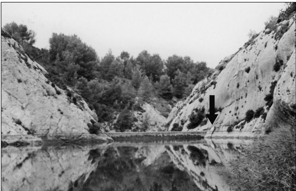
Figure 6.26 In the Baume valley, site of the Gorge of Peyrou, seen from the reservoir. The arrow shows the location of the keyway of the Roman dam, at the right extremity of the present-day dam (photo by the author).
