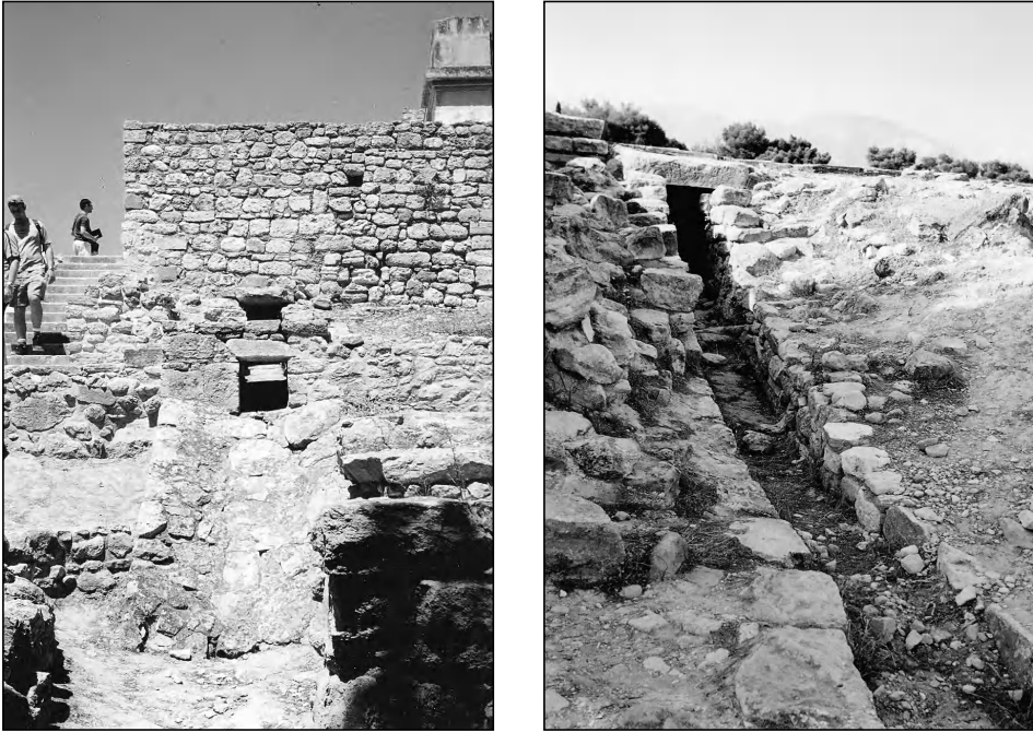
Figure 4.5. Outlets of the principal collectors of two Minoan palaces (photos by the author): - left, near the east entry of the Knossos palace; right, south of the Phaestos palace (under the large central court).
