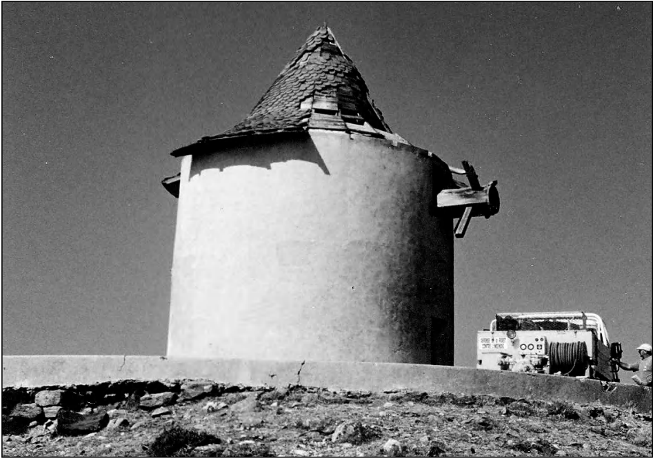
Figure 9.9 Remains of a tower mill on a hilltop in the northern extremity of Corsica. In this particular case, the unit cannot be turned into the wind (photo by the author).
