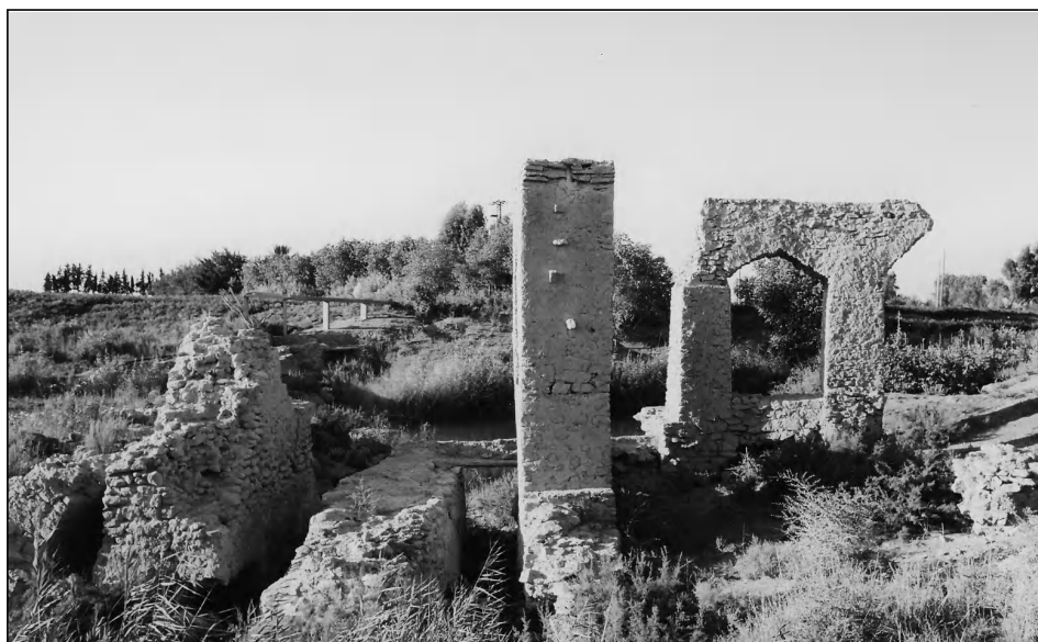
Figure 7.13 Remains of a noria at Rwashed on the Khabur, immediately upstream of its confluence with the Euphrates. This noria had three identical wheels. At the left one can see the three canals and at the right, the remains of the aqueduct (photo by the author).
