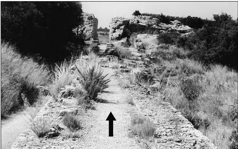
Figure 6.19 Barbegal: the remains of the canal of the left-hand aqueduct, and the notch in the rocky outcrop that marks its end (the right-hand aqueduct, though it cannot be seen in this photo, turns sharply before the rocky outcrop and continues its route toward Arles) (photo by the author).
