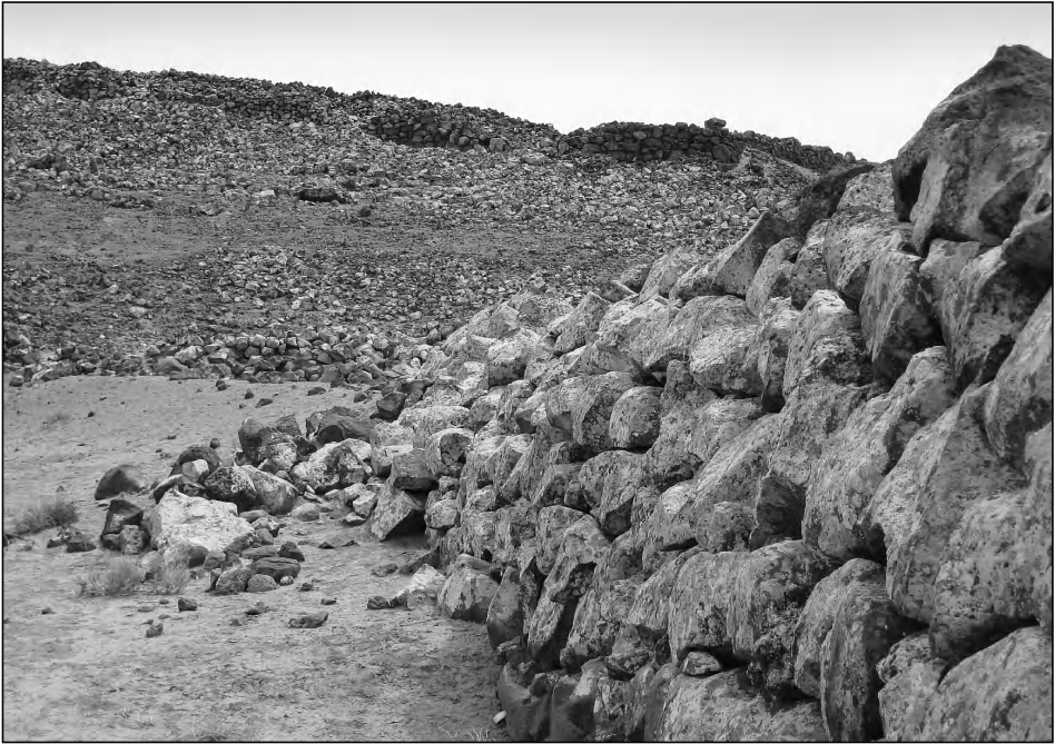
Figure 2.6b. The upstream wall of the dam forming reservoir IV in Jawa, looking toward the east. In the background, one can see the wall of the upper city of Jawa (photo by the author).
