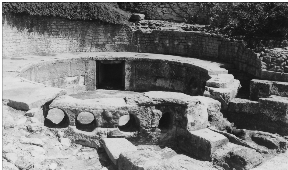
Figure 6.17 The castellum of Nîmes: this distribution basin is the terminal point of the Nîmes aqueduct. It is visible in the city, on rue de la Lampèze (photo by the author).
