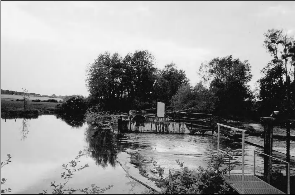
Figure 9.6 The dam on the Serein (renovated in modern times) that forms the race of Pontigny. At the left one can see the start of the race (photo by the author).
