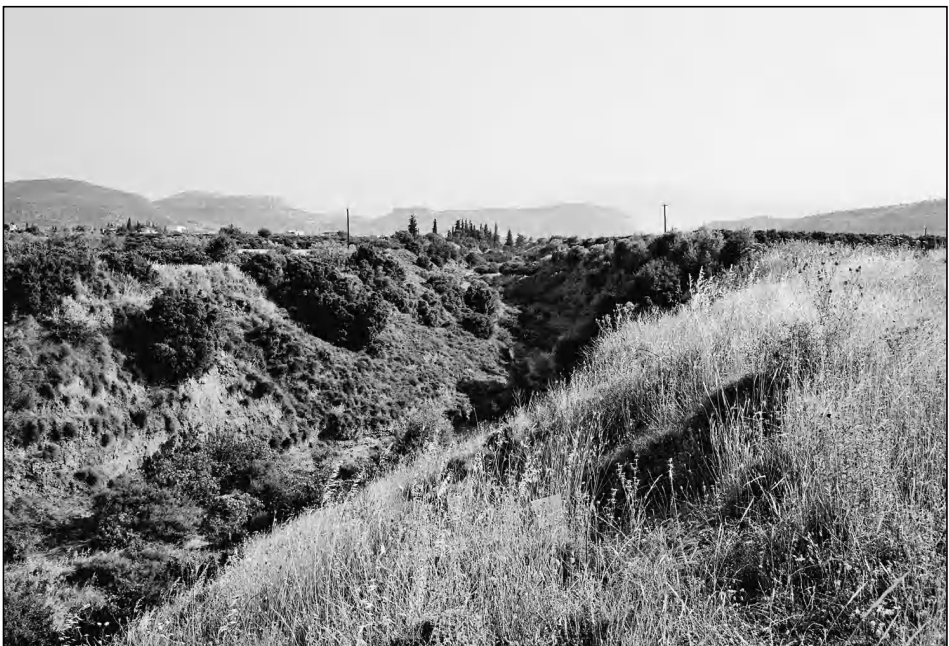
Figure 4.14 Lakissa diversion canal, looking from the top of the Kofini dam (photo by the author).
