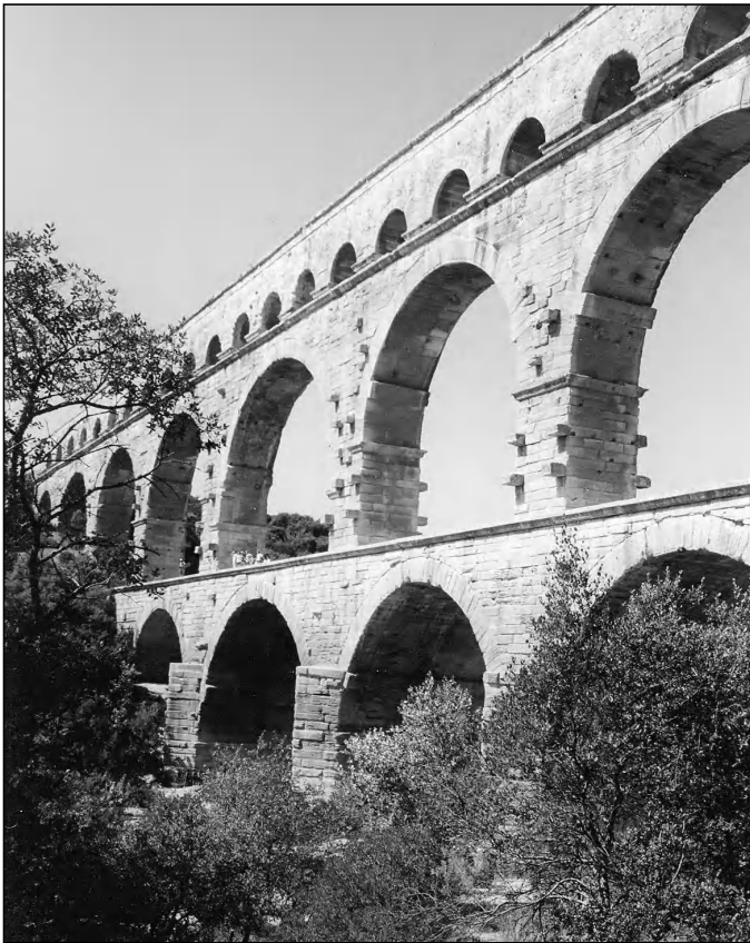
Figure 6.15 The Pont du Gard, supporting the aqueduct of Nîmes across the Gardon (photo by the author).
