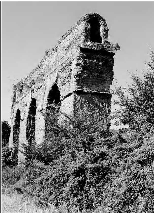
Figure 6.6 The Anio Novus, one of the greatest Roman aqueducts, supported by arches in the Anio valley, between Tivoli and Castel madama. The canal, still lined with opus signinum, is well conserved. This aqueduct was built in 52 AD near the end of the reign of emperor Claudius (who also was responsible for the Aqua Claudia aqueduct), and is some 87 km long. It carries water captured from the Anio river, in the Sabine mountains near Subiaco. (photo by the author).
