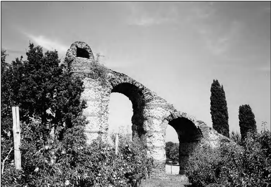
Figure 6.40. Aqueduct of Gier for Lyon: seen from the upstream end of the siphon of Yzeron, at the place called “le plat de l’air”. From left to right: hidden behind the trees, the arches that support the canal, the remains of the head tank, and the ramp, the inclined plain that carried the lead pipes descending into the valley to the bridge-siphon (photo by the author).
