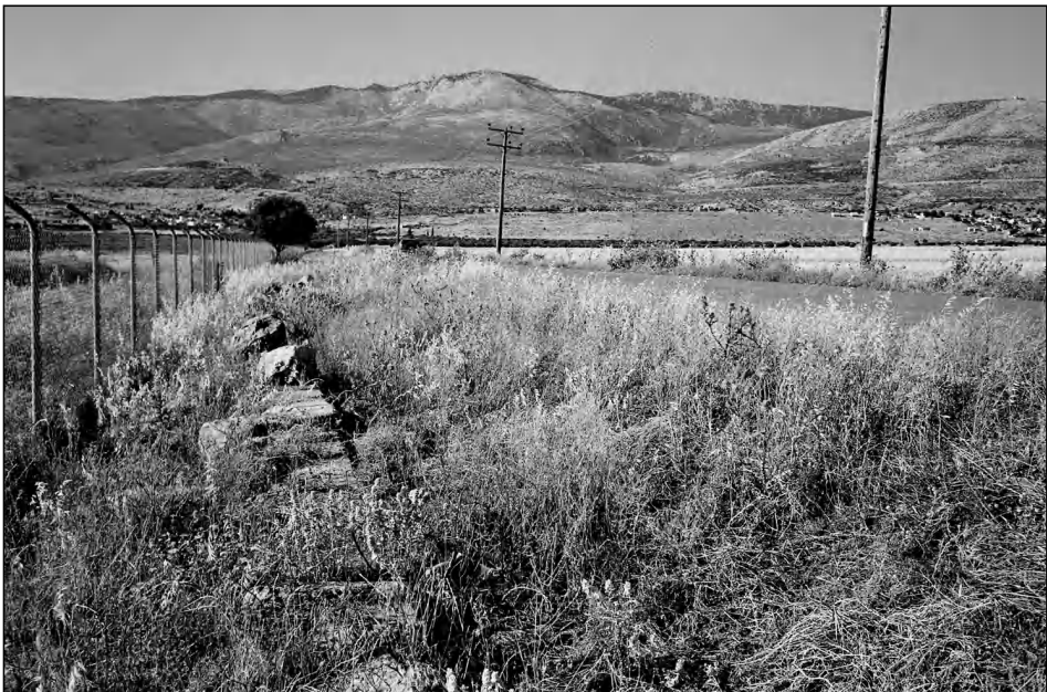
Figure 4.11 Remains of the Kineta dam (Thisbe), 1,200 m long. The modern road was built on top of the ancient dam; at the left, remains of the wall of large cut stone (photo by the author).
