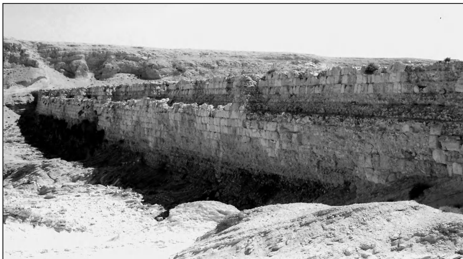
Figure 6.34 In a land of minerals, the dam of Harbaqa across the valley of a Wadi. The impoundment is today completely filled in, but the dam enables the fill to retain sufficient moisture for farming. View from downstream (photo by the author).
