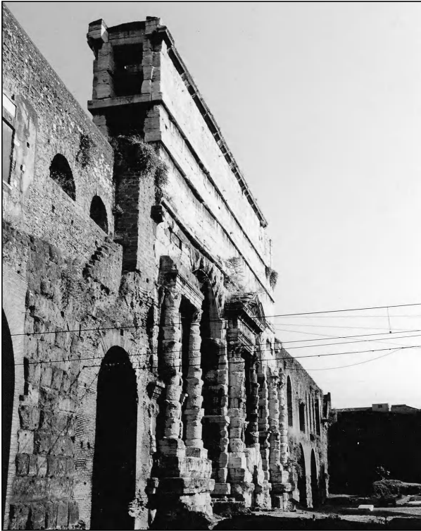
Figure 6.9 The Aqua Claudia and the Aqua Anio Novus on the same arches, at the Porta Maggiore of Rome. The aqueduct was integrated into the new city wall under the emperor Aurelius, in the 4th century AD (photo by the author).
