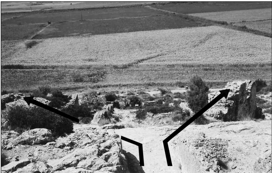
Figure 6.22 Roman flour mill at Barbegal: view from the summit of the rock outcrop where the aqueduct arrives; to the left and the right, in the form of a V, one can see the two walls that carried the two divergent lateral canals. These canals delivered water to the two "mill" canals that, in turn, cascaded down the slope and supplied the two banks of water wheels (photo by the author).
