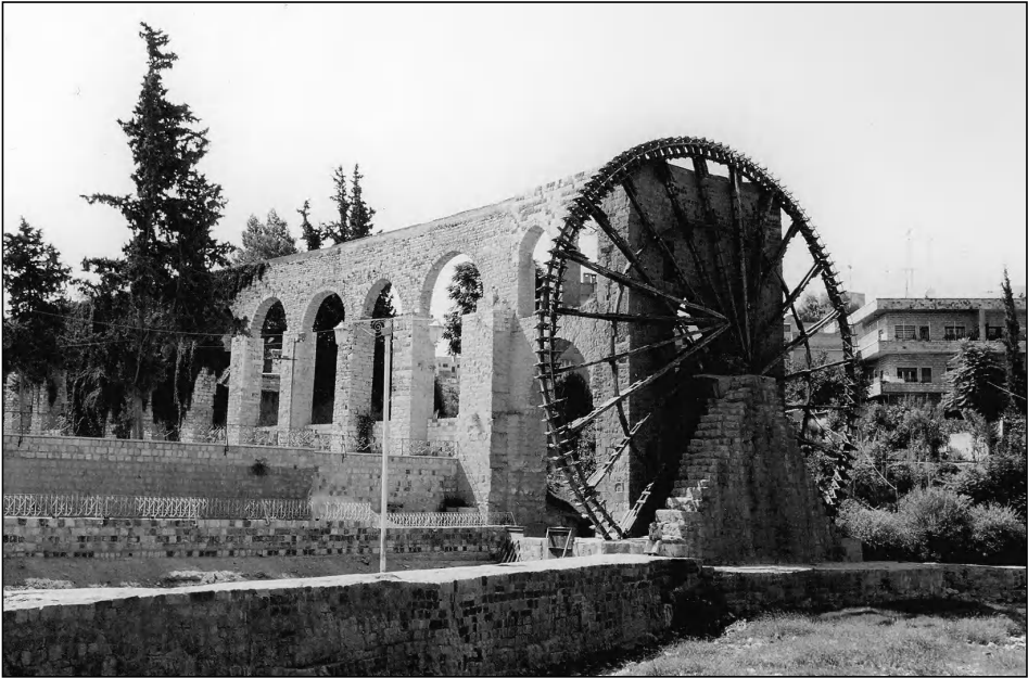
Figure 7.7 The noria al-Muhammadiya and its aqueduct at Hama, dated as 1361 from the inscription on a pillar of the aqueduct. As are the other norias of Hama, this one has been maintained and regularly renovated since its initial construction. With a diameter of 21 m, it is the largest known ancient noria (photo by the author).
