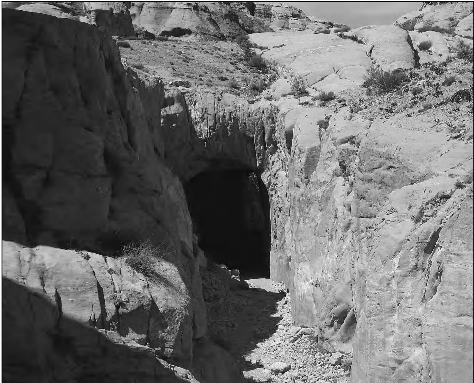
Figure 5.13b. The tunnel constructed by the Nabateans to redirect the flood waters of the Musa wadi towards the el-Mudhim wadi. The tunnel is, at its entrance, 9 m high and 6 m wide (photo by the author).
