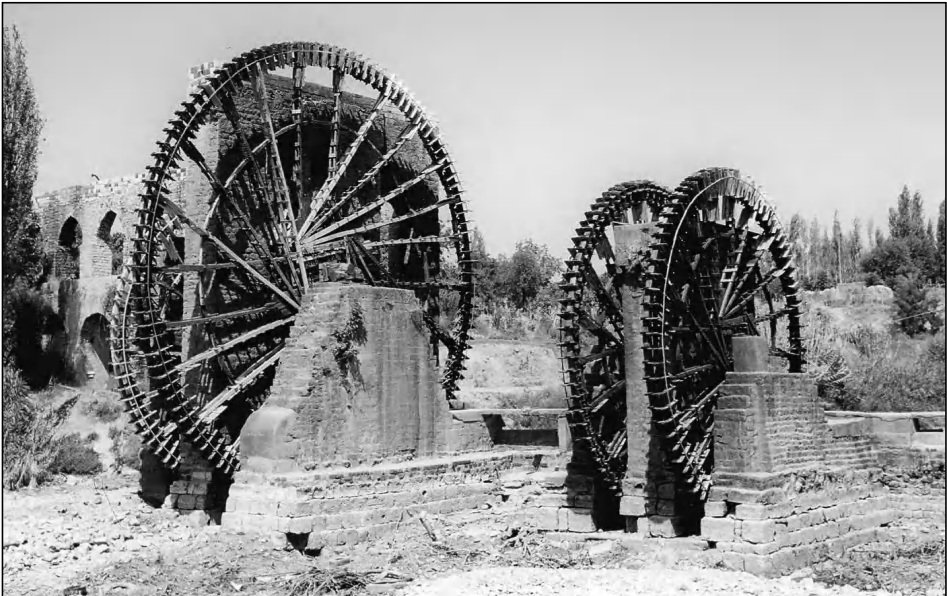
Figure 7.8 The group called the “four norias” at the entrance of the Orontes into Hama. The aqueduct of the two norias at the right has disappeared (photo by the author).
