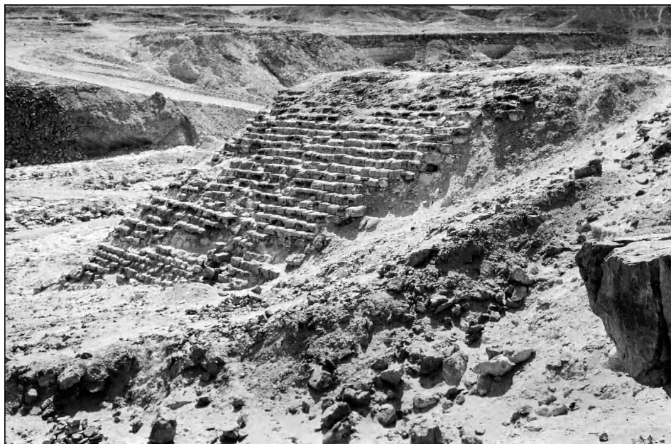
Figure 3.3 Remains of the Sadd el Kafara dam (about 2600 BC), on the right bank of the wadi Garawi . The oldest known large dam. View from upstream (photo of G. Garbrecht)
