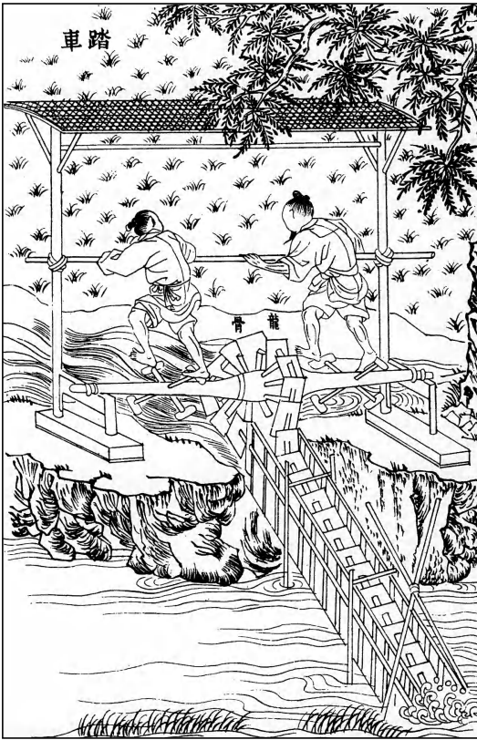
Figure 8.18 The square-pallet chain pump, or dragon backbone machine; this is the most widespread lifting machine in China. Above, Chinese illustration from 1637 (after Needham and Ling, 1965); below, western engraving from 1757 (Chambers – ancient archives of ENPC).
