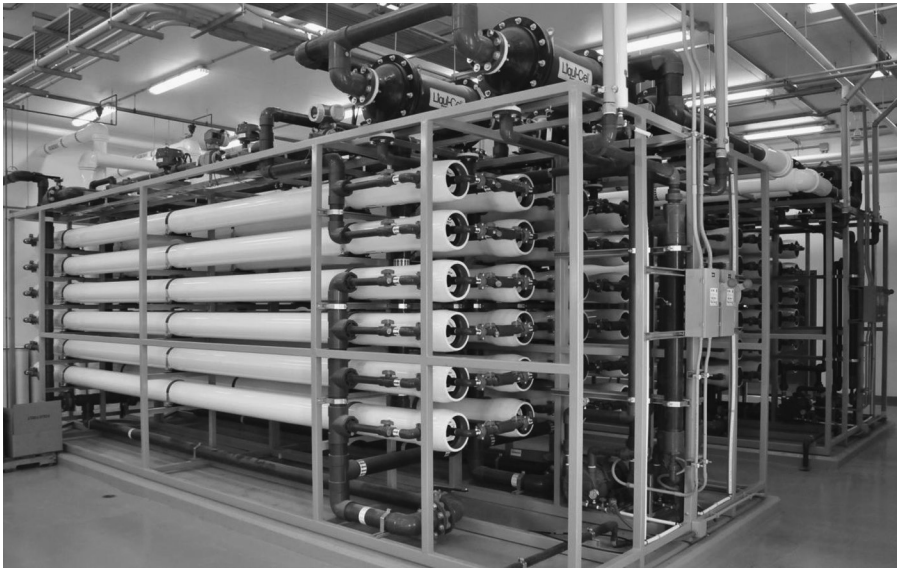
FIGURE 9.6 An RO membrane filtration system using spiral wound modules.
